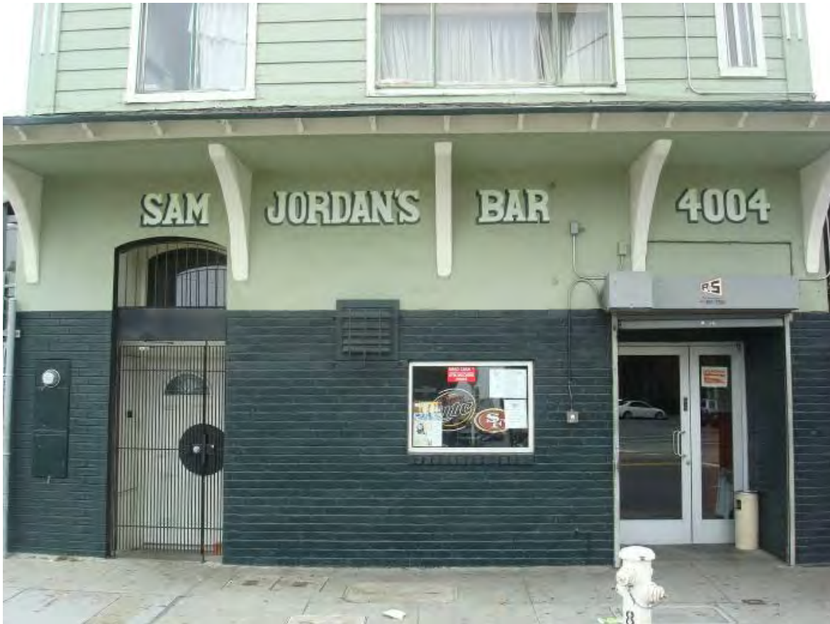
First story, primary facade.
