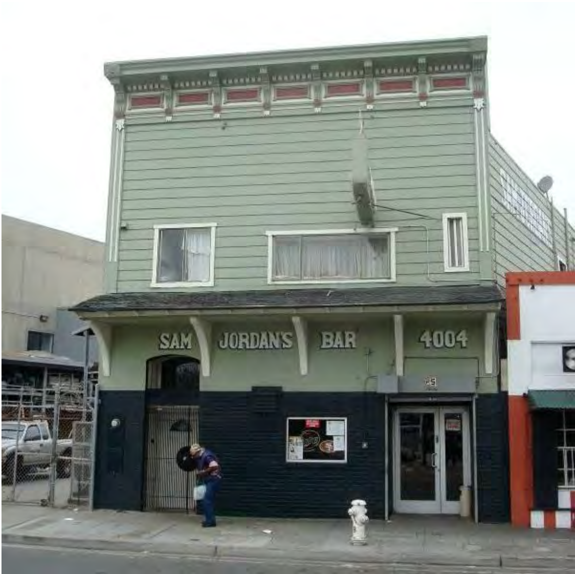
4004-4006 Third Street, Sam Jordan's Bar, primary facade.
