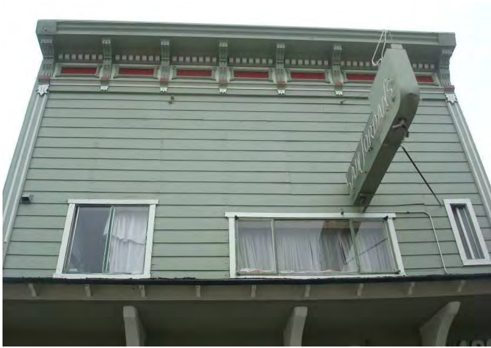
Second story, primary facade.
