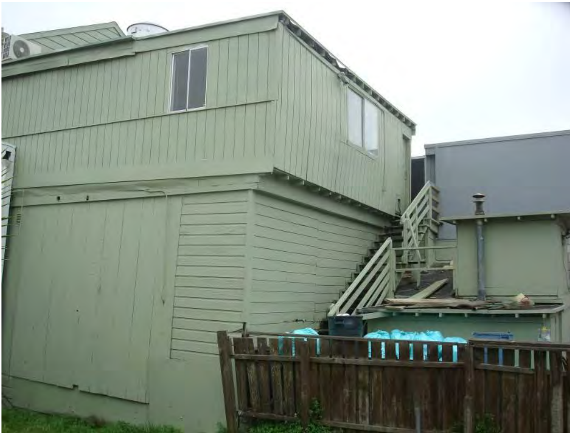
North-west corner of the building, showing rear addition.
