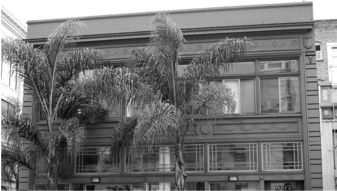
Upper portion of 1033-1037 Polk Street, showing classical ornament. Arthur S. Bugbee, architect, 1920. Auto parts stores occupied the two storefronts from 1920 into the early 1930s.
