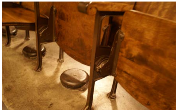
Figure 41. Heating units beneath seats.
