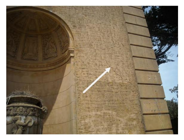
Photo 4.2 Crack at the Existing Wall
