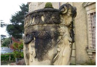
Figure 5.17: Urn covered in general soiling, east elevation.
