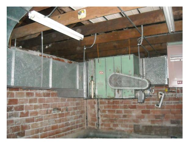
Photo 4.11 Mechanical Equipment with No Seismic Bracing
