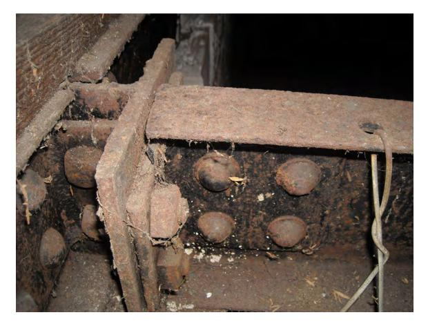
Photo 4.4 Corrosion at Steel Connection
