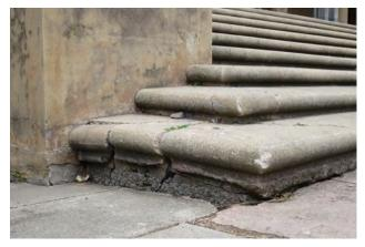
Figure 5.30: Damaged stairs, east elevation.
