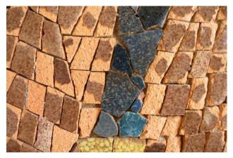
Figure 5.38: Grout loss and spalling of glazed surface, north wall.
