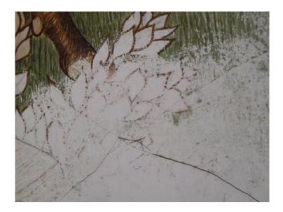
Note: Cracks, and the remains of the original design, are noted in this area of water penetration near the bottom edge of the west wall.
