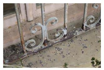
Figure 5.24: Corrosion of the metal grill at the large, 16-lite paired casement sash window, east elevation.
