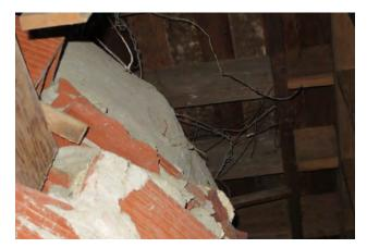
Figure 5.12: Backside of a recessed apse showing pre-cast elements held in place using steel wires.
