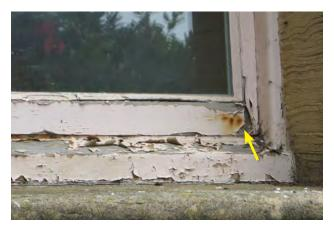
Figure 5.20: Typical paint failure and corrosion of fasteners at north, west and south elevation windows.
