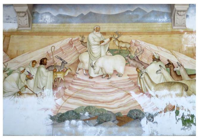
Figure 5.51: West wall mural area above the large central window showing damage and loss, main lounge (100).
