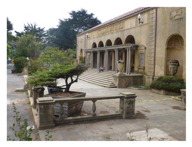
Photo 2.2 Loggia East Steel Columns with Precast Concrete Surroundings
