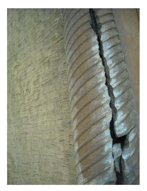
Photo 4.7 Damaged Precast Door Surrounding
