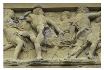
Figure 5.13: Concrete deterioration, frieze above the main entrance.
