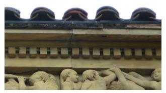
Figure 5.3: Damaged cornice exhibiting wood deterioration and cracked concrete, east elevation.
