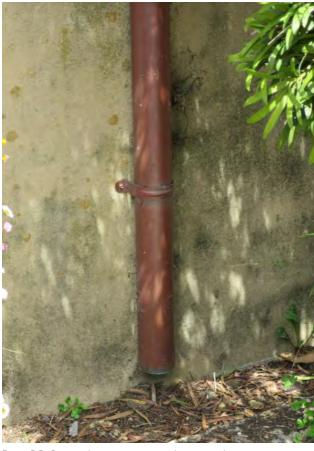
Figure 5.5: Copper downspout on east elevation without an extension.
