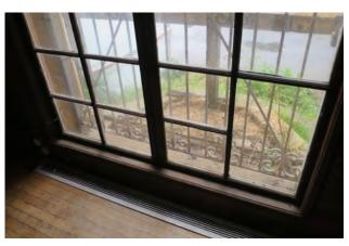
Figure 5.23: Missing mullion at the 16-lite paired casement sash window, east elevation.
