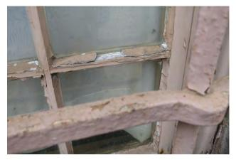
Figure 5.22: East elevation window exhibiting paint and glazing putty failure.
