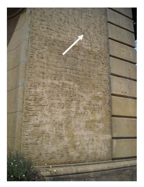
Photo 4.1 Crack at the Existing Wall
