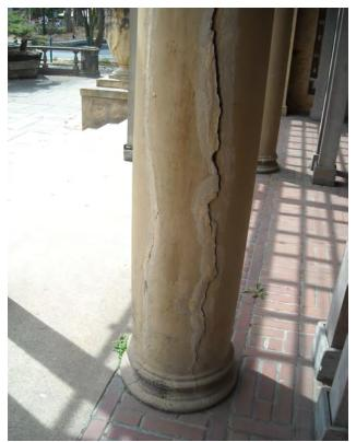
Figure 5.58: Crack at a loggia column. (Source: SOHA)
