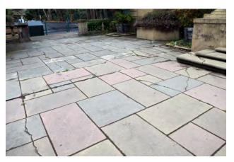
Figure 5.31: Cracks in the pavement, east elevation.
