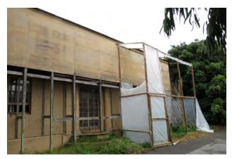
Figure 5.8: Wood framed scaffold at west elevation.
