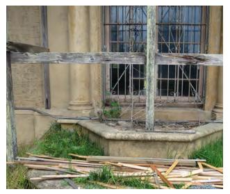
Figure 5.9: Wood framed scaffold at west elevation .
