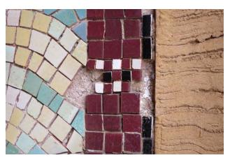
Figure 5.37: Missing tiles, north wall.
