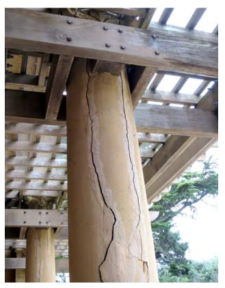
Figure 5.14: Column deterioration at the east loggia.
