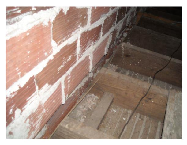
Photo 4.3 No Attic Floor to Wall Connection
