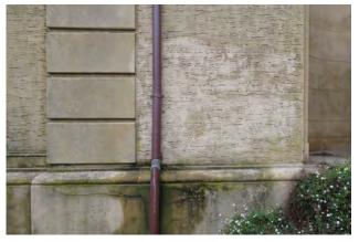
Figure 5.18: Overpaint on the stucco, east elevation.
