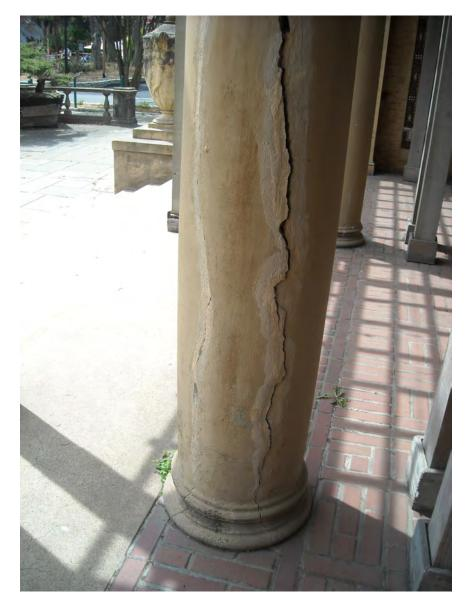
Photo 4.6 Large Cracks at Precast Steel Column Surrounding
