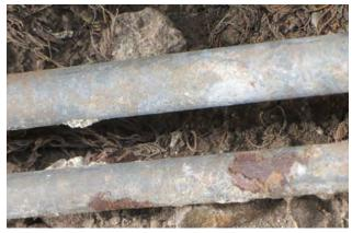
Figure 5.63: Corroded piping in crawlspace.
