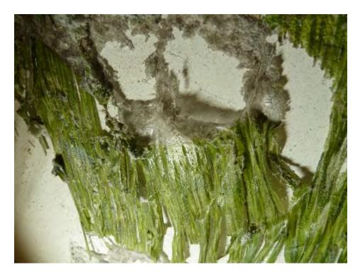
**Note:** Details on the west wall of previously restored areas, consisting of acrylic emulsion paints, seen here in raking light. These paints are film-forming and do not allow the plaster to breathe. The paint is pushed from the wall by moisture and/or salts, and has fallen onto the ledges below the west wall.
