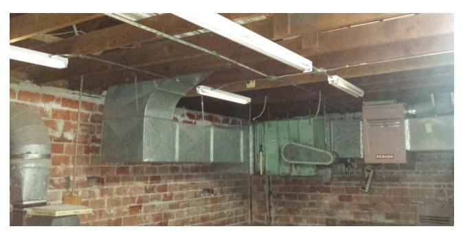
Figure 5.61: Ceiling-hung furnace in the south attic.
