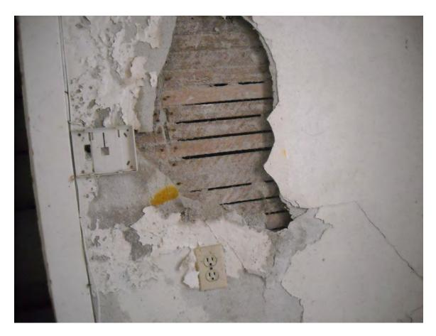
Photo 4.10 Damaged Lath and Plaster
