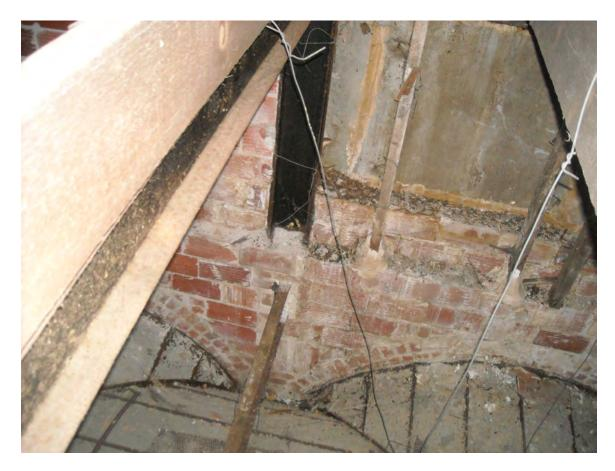
Photo 4.9 Frieze Panels with Inadequate Support
