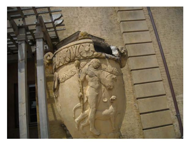
Photo 4.8 Damaged Precast Concrete Urn
