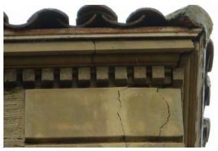
Figure 5.4: Damaged cornice showing corroded flashing, south elevation.
