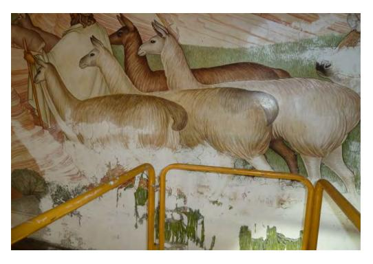
Note: A large expanse of paint loss exists in the lower section of the west wall. Former repairs have failed, indicating that the water damage to this wall is a consistent problem, requiring extensive repair. Preservation of the mural cannot succeed without halting the water penetration and ambient environmental fluctuations.
