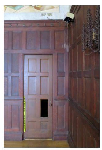
Figure 5.47: East elevation door in the main lounge (100) missing a panel.
