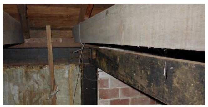
Figure 5.56: Framing above loggia. Note the backside of the precast frieze panel on the back wall.
