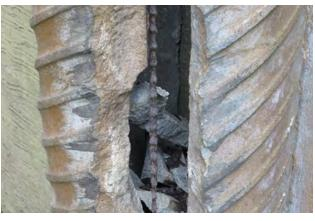
Figure 5.15: North elevation entrance column deterioration.
