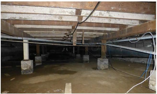
Figure 5.6: Soil around the foundation piers was found to be wet.
