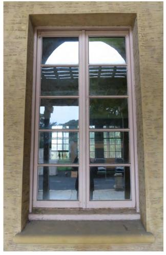
Figure 5.19: 5-lite paired casement sash window at the east loggia.
