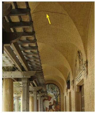
Figure 5.33: Crack in the ceiling highlighted by dark discoloration.
