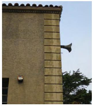
Figure 5.10: Full-height crack at corner, south elevation.
