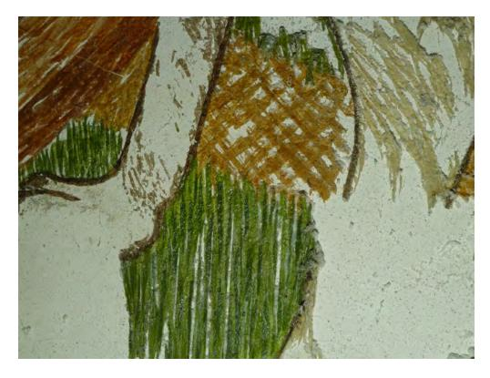
**Note:** Another detail of a restored area on the west wall, consisting of acrylic emulsion paints. These paints are film-forming and do not allow the plaster to breathe. The paint is pushed from the wall by moisture and/or salts. Acrylic emulsion paints fall away in sheets, unlike the crumbling of the original (thinner) egg tempera.
