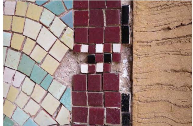
Figure 5.37: Missing tiles, north wall.
