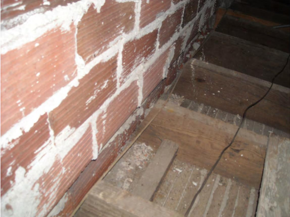
Photo 4.3 No Attic Floor to Wall Connection
