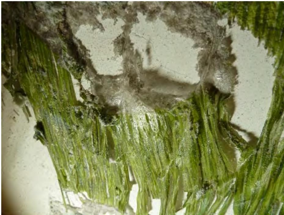
**Note:** Details on the west wall of previously restored areas, consisting of acrylic emulsion paints, seen here in raking light. These paints are film-forming and do not allow the plaster to breathe. The paint is pushed from the wall by moisture and/or salts, and has fallen onto the ledges below the west wall.
