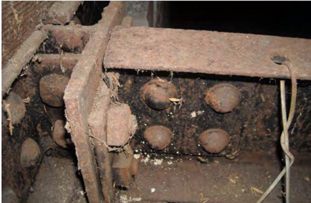
Figure 5.57: Corrosion at steel connections (Source: SOHA)
