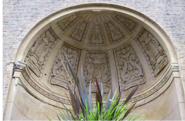
Figure 5.11: Deterioration of a recessed apse ceiling, east elevation.
