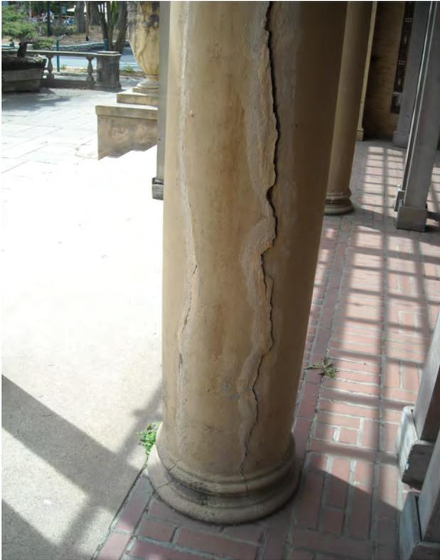
Figure 5.58: Crack at a loggia column. (Source: SOHA)
