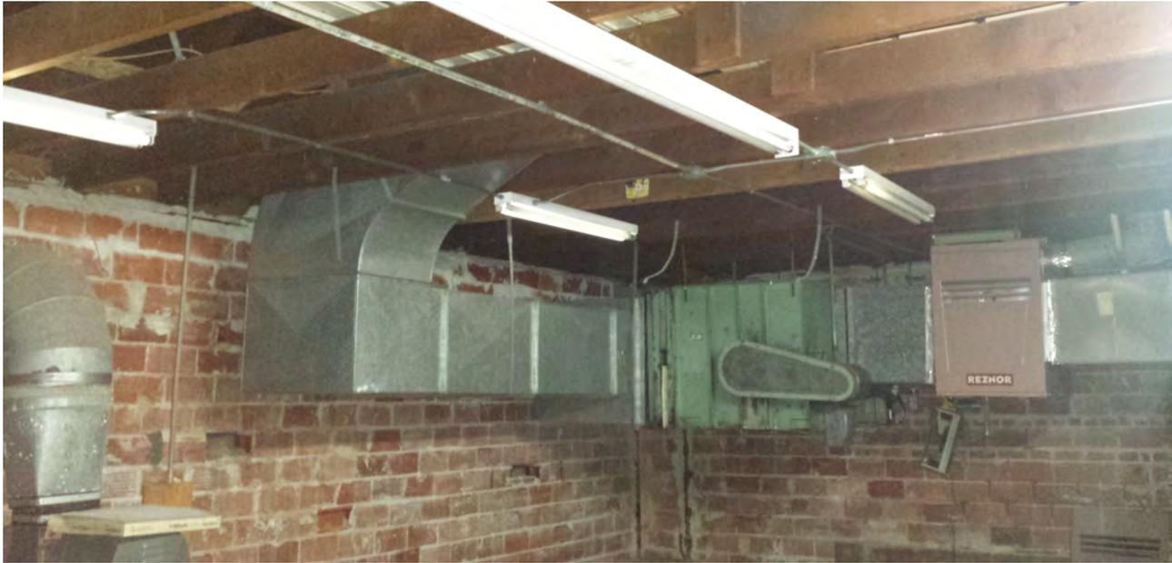
Figure 5.61: Ceiling-hung furnace in the south attic.
