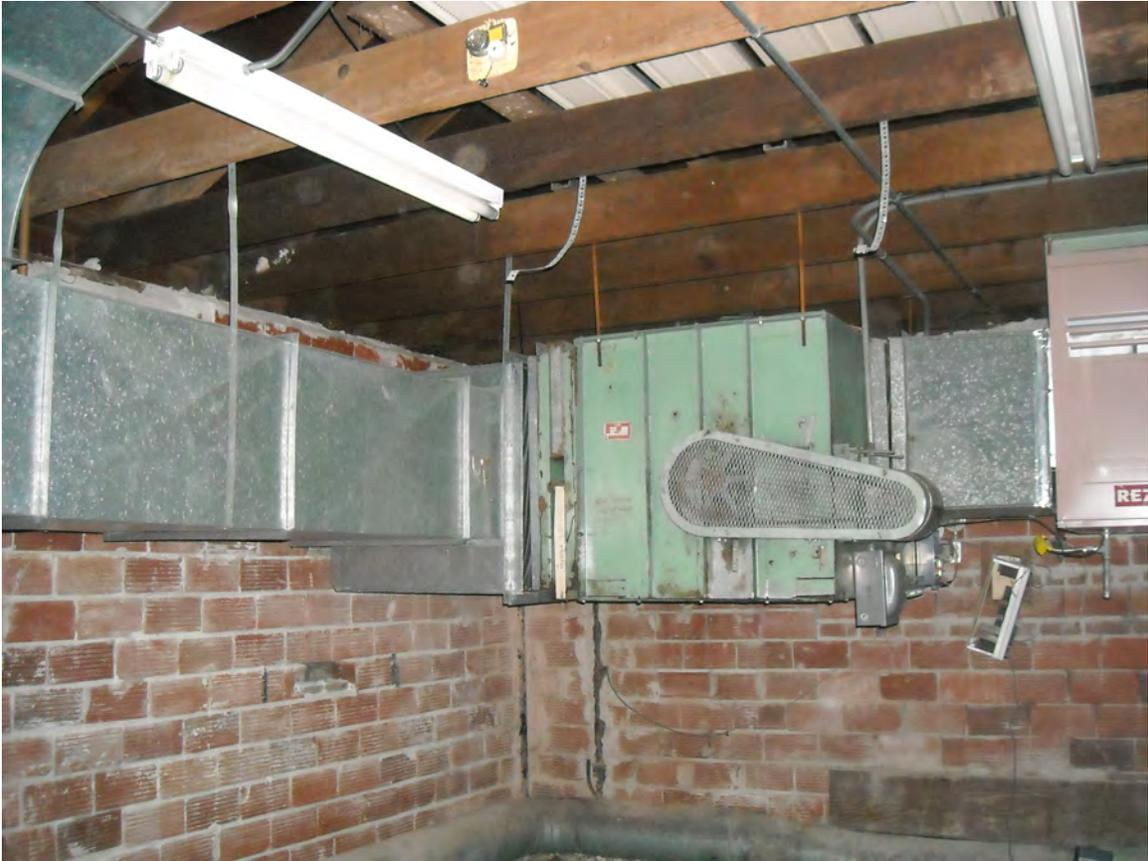
Photo 4.11 Mechanical Equipment with No Seismic Bracing
