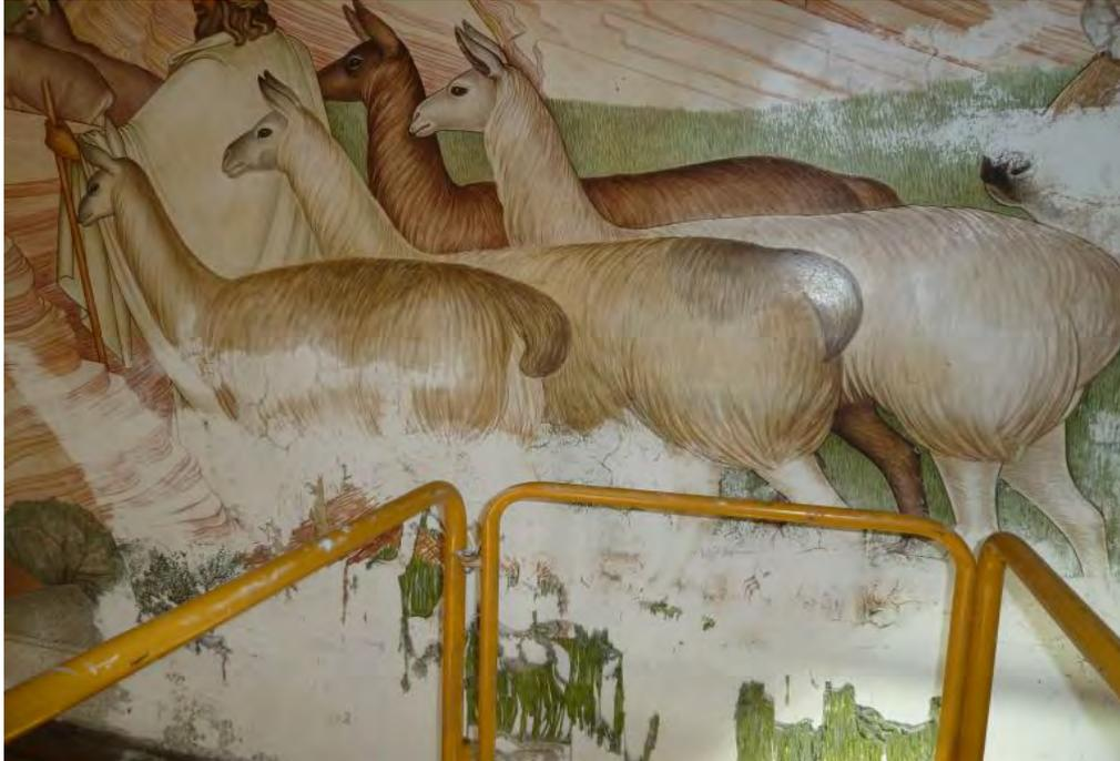
Note: A large expanse of paint loss exists in the lower section of the west wall. Former repairs have failed, indicating that the water damage to this wall is a consistent problem, requiring extensive repair. Preservation of the mural cannot succeed without halting the water penetration and ambient environmental fluctuations.
