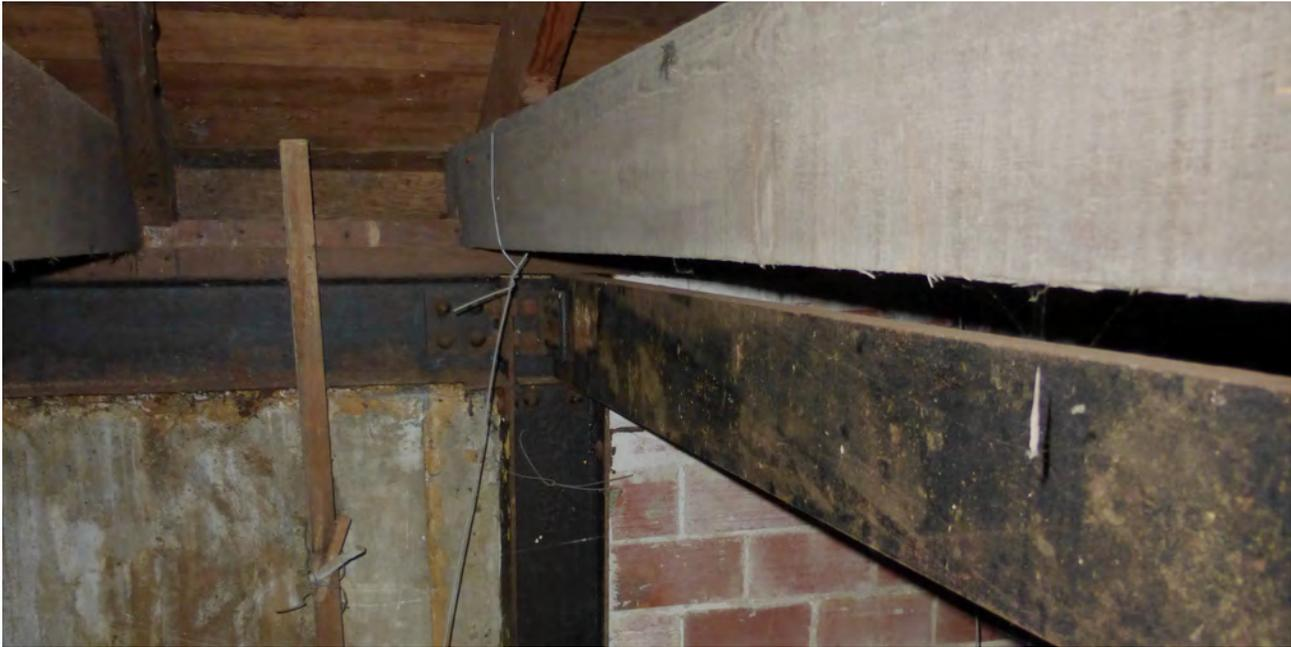
Figure 5.56: Framing above loggia. Note the backside of the precast frieze panel on the back wall.
