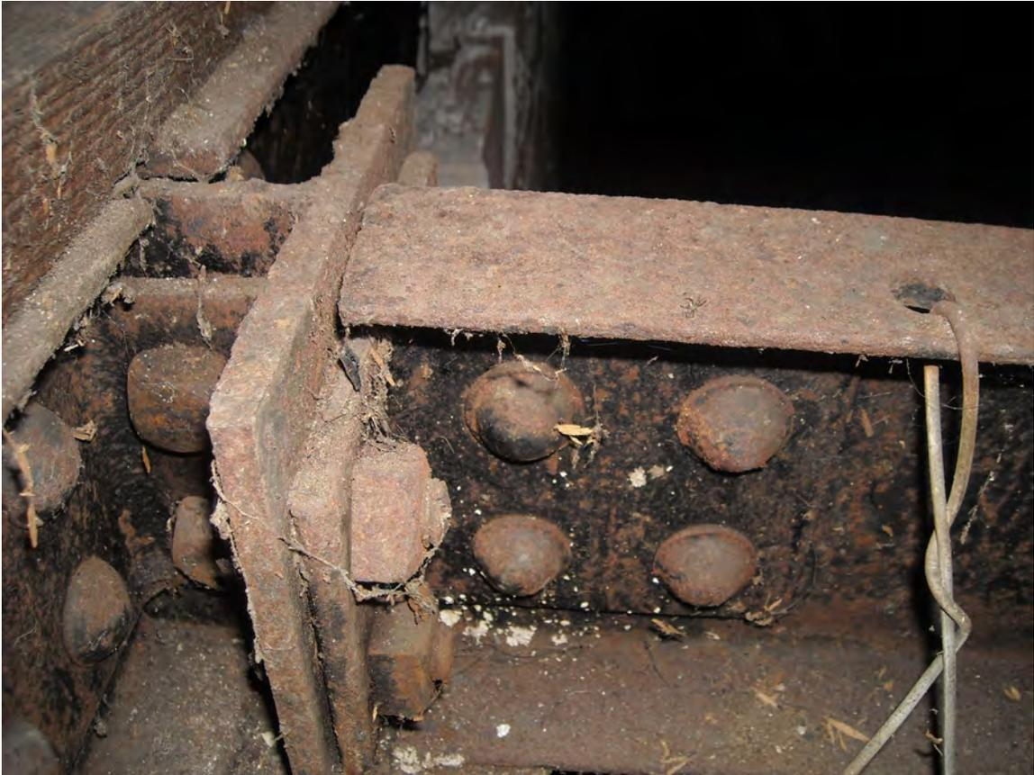
Photo 4.4 Corrosion at Steel Connection
