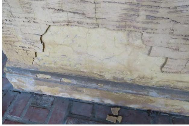
Figure 5.16: Example of stucco exfoliation, east elevation of the loggia.
