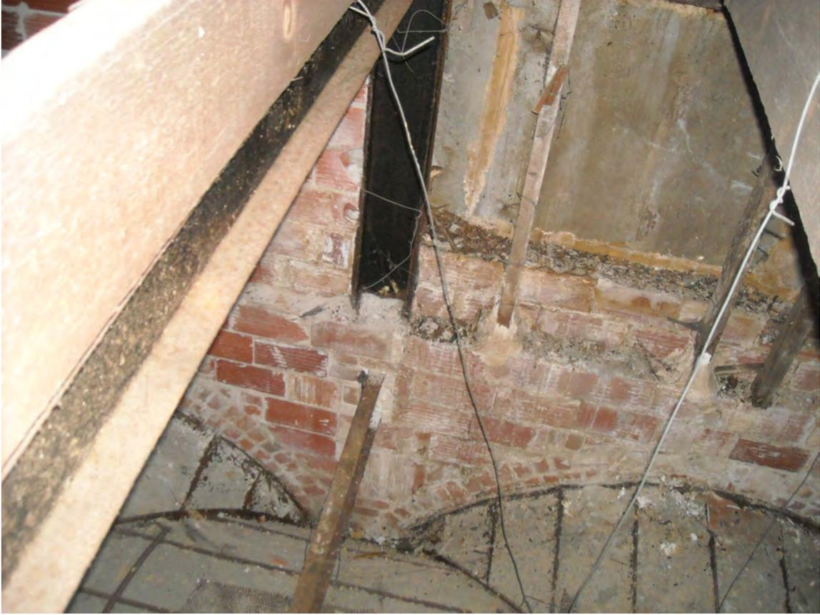
Photo 4.9 Frieze Panels with Inadequate Support
