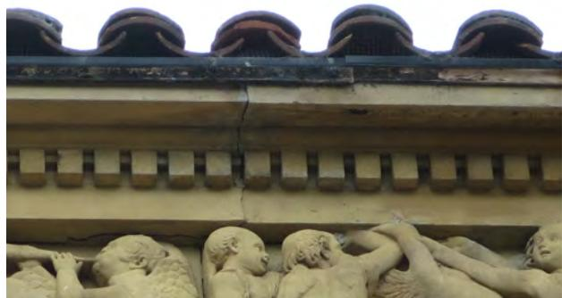
Figure 5.3: Damaged cornice exhibiting wood deterioration and cracked concrete, east elevation.
