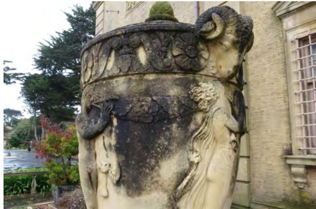
Figure 5.17: Urn covered in general soiling, east elevation.
