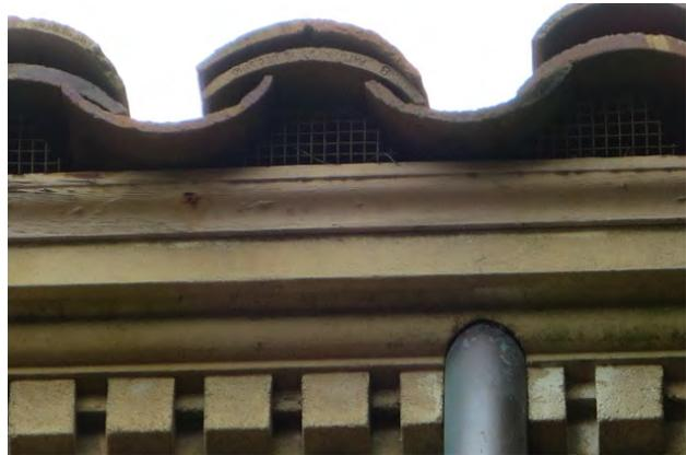
Figure 5.2: Built-in gutter at the roof edge .
