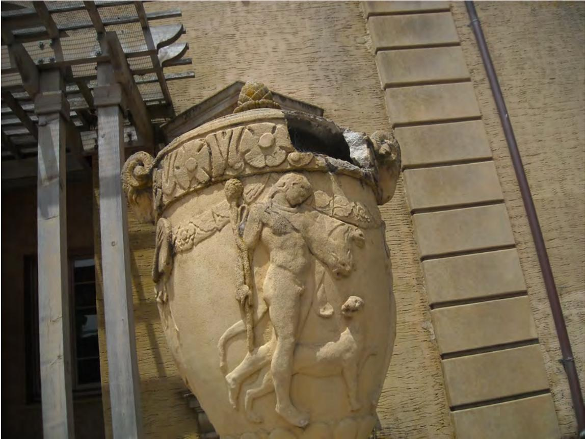
Photo 4.8 Damaged Precast Concrete Urn
