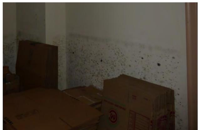
Figure 5.42: Mold on wall surfaces, Room 108.
