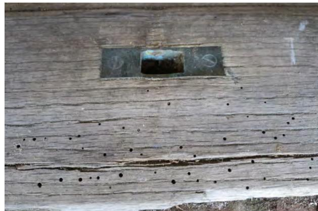
Figure 5.26: Main entrance door threshold infested with beetles or drywood termites.
