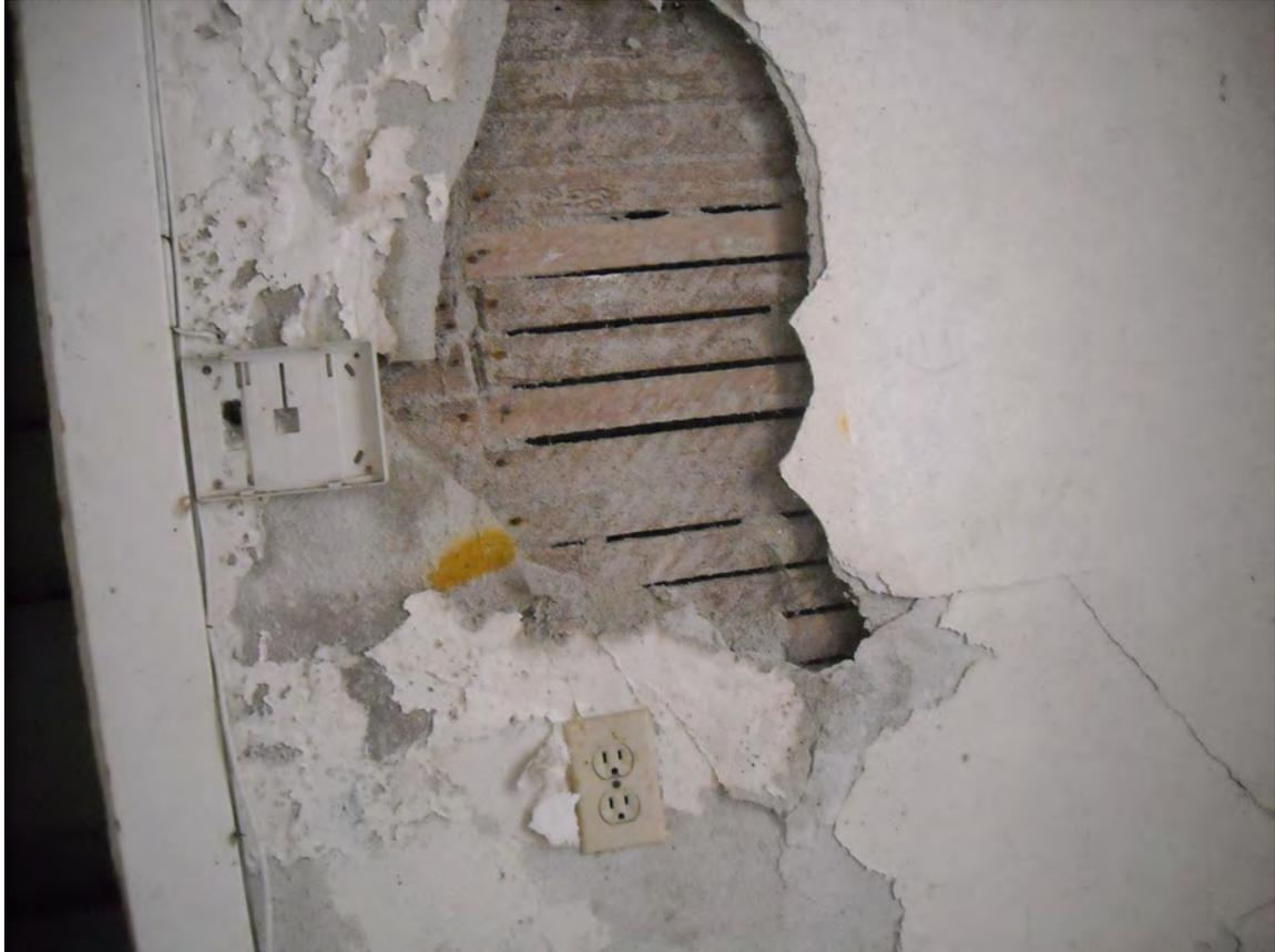
Photo 4.10 Damaged Lath and Plaster
