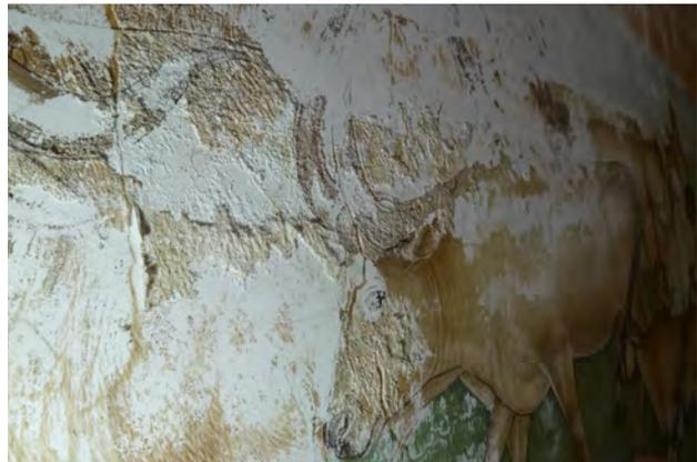
Figure 5.53: West wall detail showing the extent of deterioration of the plaster and paint, main lounge (100). (Source: Anne Rosenthal)
