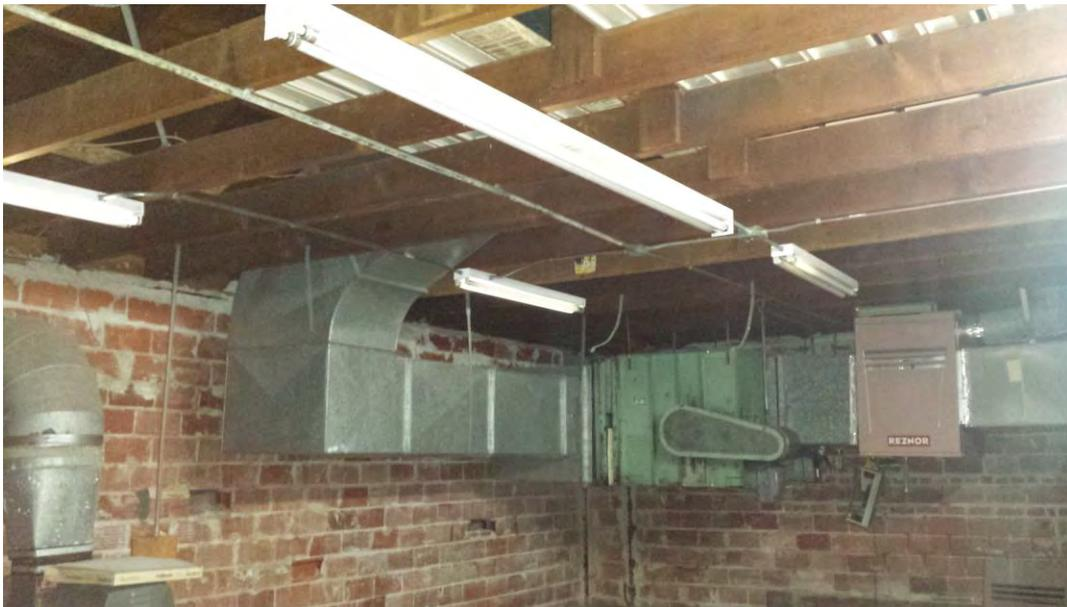
Existing furnace and associated ductwork in second floor mechanical room.
