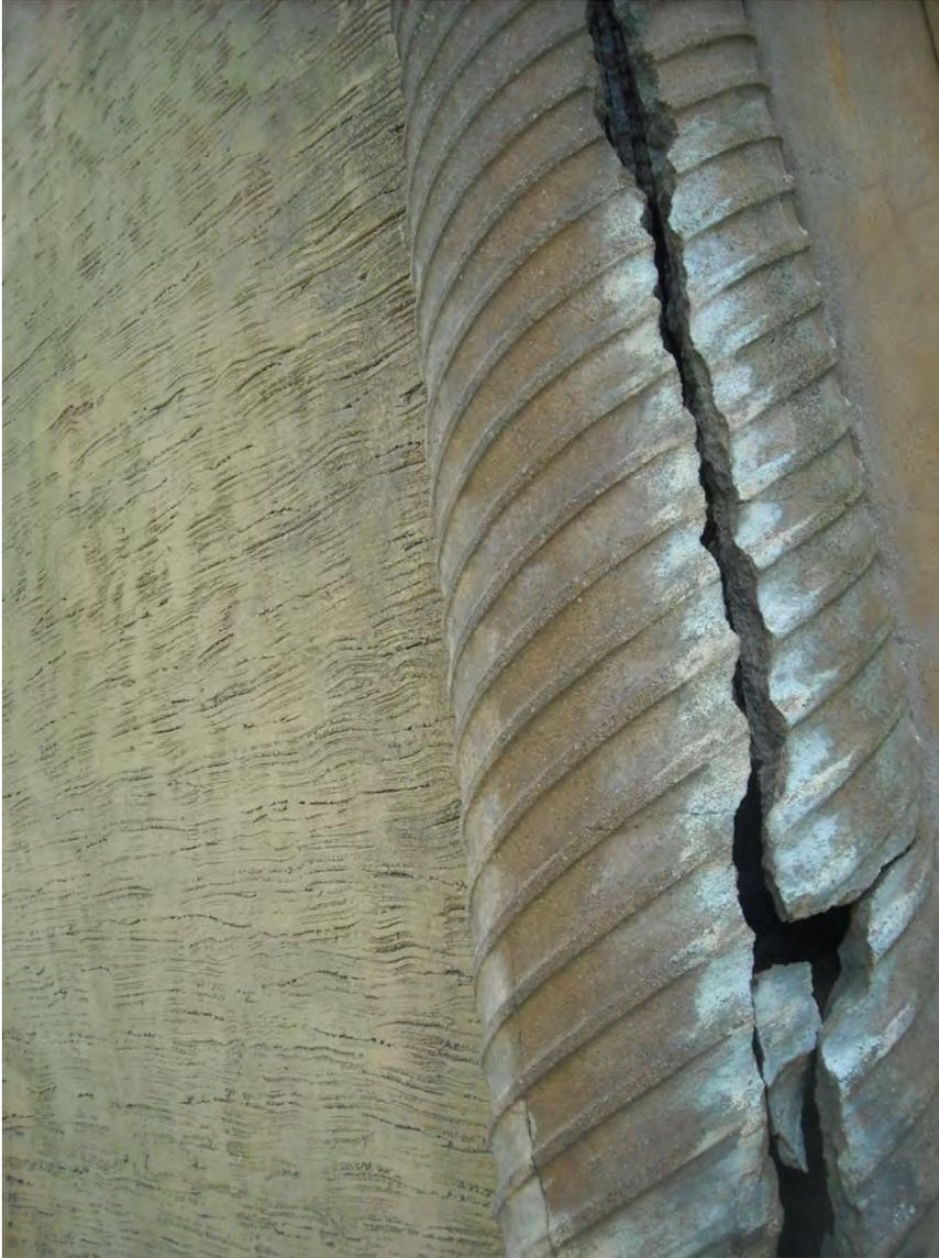
Photo 4.7 Damaged Precast Door Surrounding
