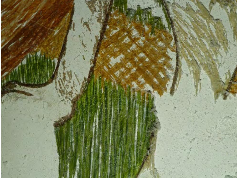
**Note:** Another detail of a restored area on the west wall, consisting of acrylic emulsion paints. These paints are film-forming and do not allow the plaster to breathe. The paint is pushed from the wall by moisture and/or salts. Acrylic emulsion paints fall away in sheets, unlike the crumbling of the original (thinner) egg tempera.
