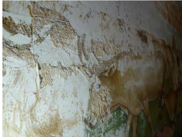
**Note:** Details of other areas showing the extent of deterioration of the plaster and paint.
