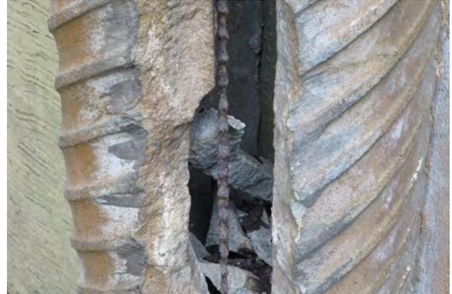
Figure 5.15: North elevation entrance column deterioration.
