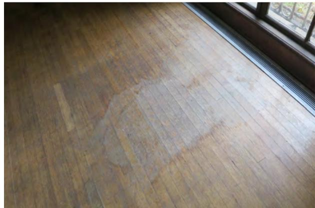
Figure 5.44: Weathered finish from water damage near the large, central window on the west wall, main lounge (100).
