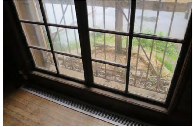
Figure 5.23: Missing mullion at the 16-lite paired casement sash window, east elevation.
