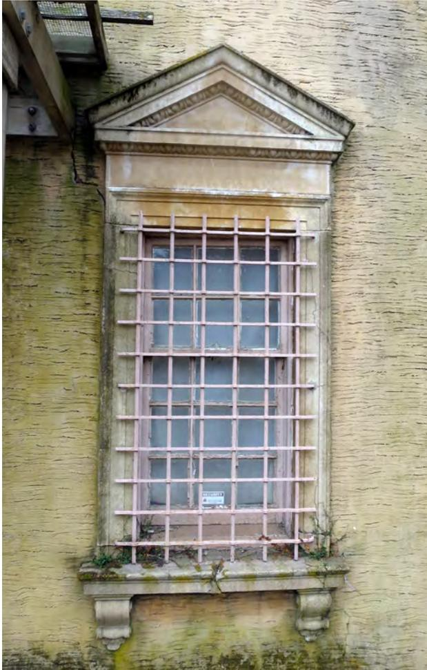
Figure 5.21: 6 over 9 double-hung window at east elevation.
