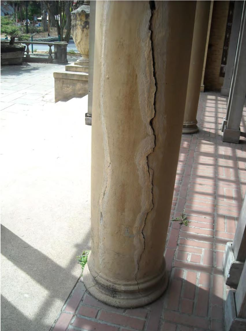
Photo 4.6 Large Cracks at Precast Steel Column Surrounding
