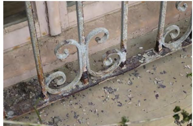
Figure 5.24: Corrosion of the metal grille at the large, 16-lite paired casement sash window, east elevation.
