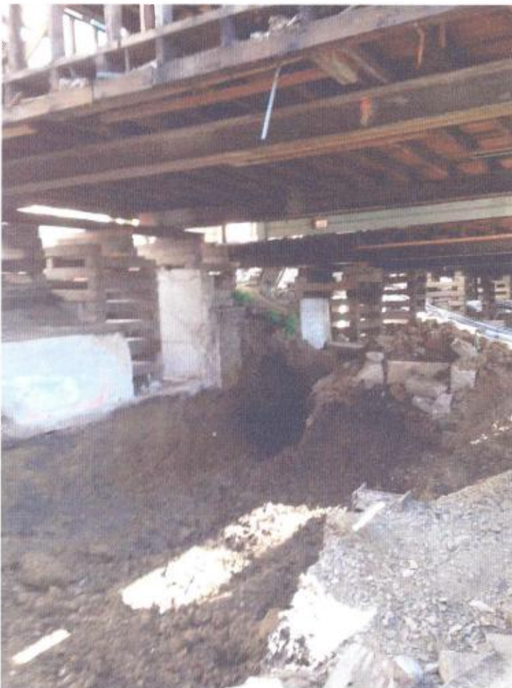
Cottages shored and cribbed during Rehabilitation
