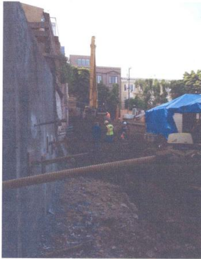
Ties Backs in Consolidated Larkin Retaining Walls
