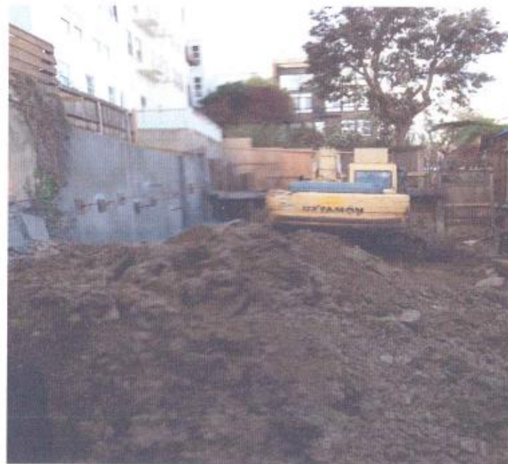
Ties Backs in Consolidated Larkin Retaining Walls
