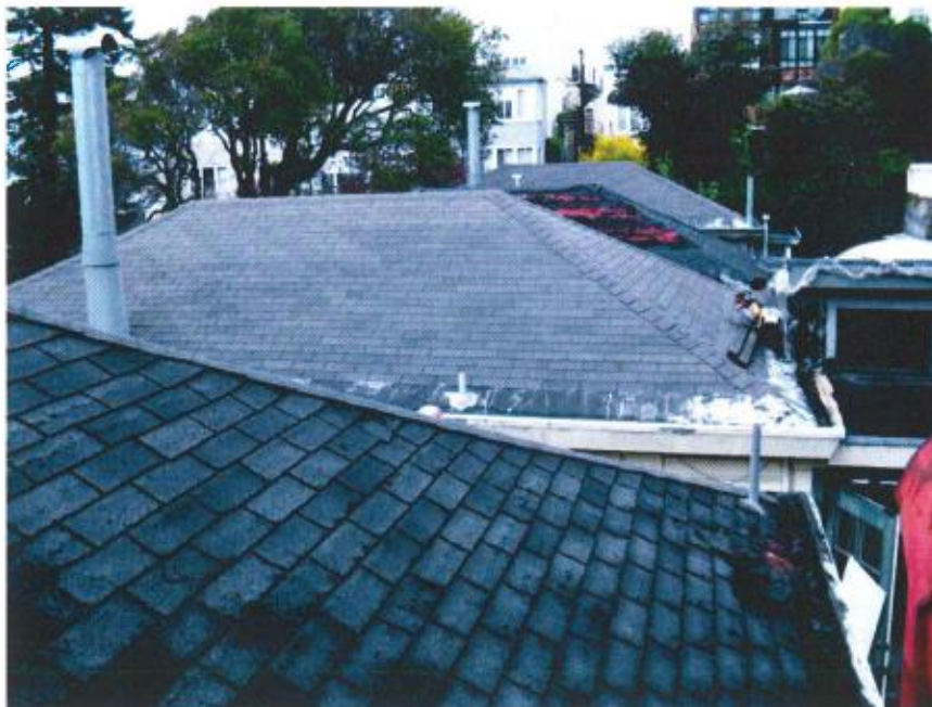
Figure 5. Detail of cottage roofs. Note the round metal flues on the cottages.
