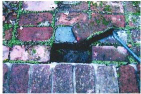
Figure 3: Bedding is a soil/sand mixture
