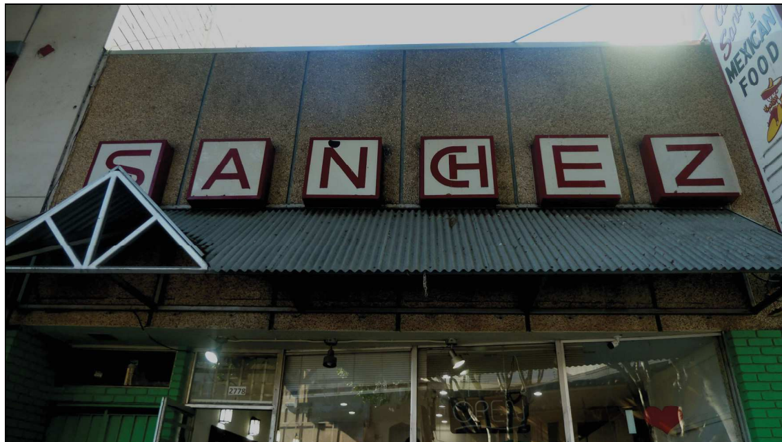
6 of 15. Sanchez sign above awning on primary façade, north view from 24 th Street
