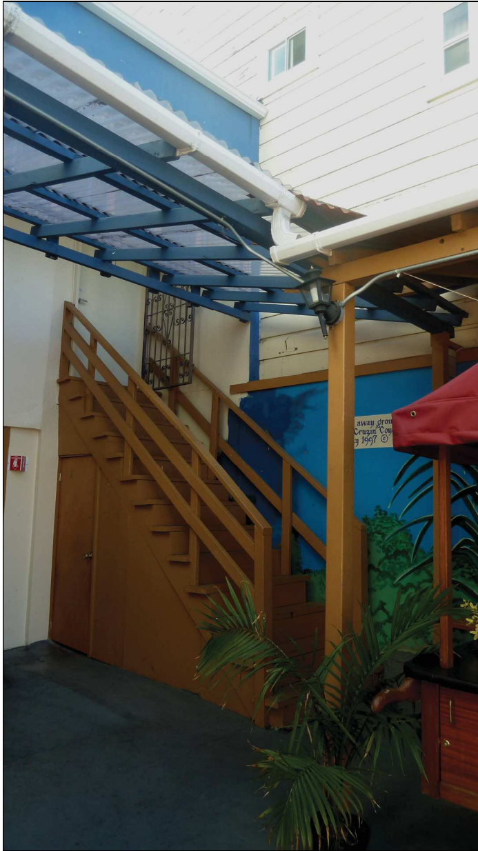
14 of 15. Stairs rear façade
