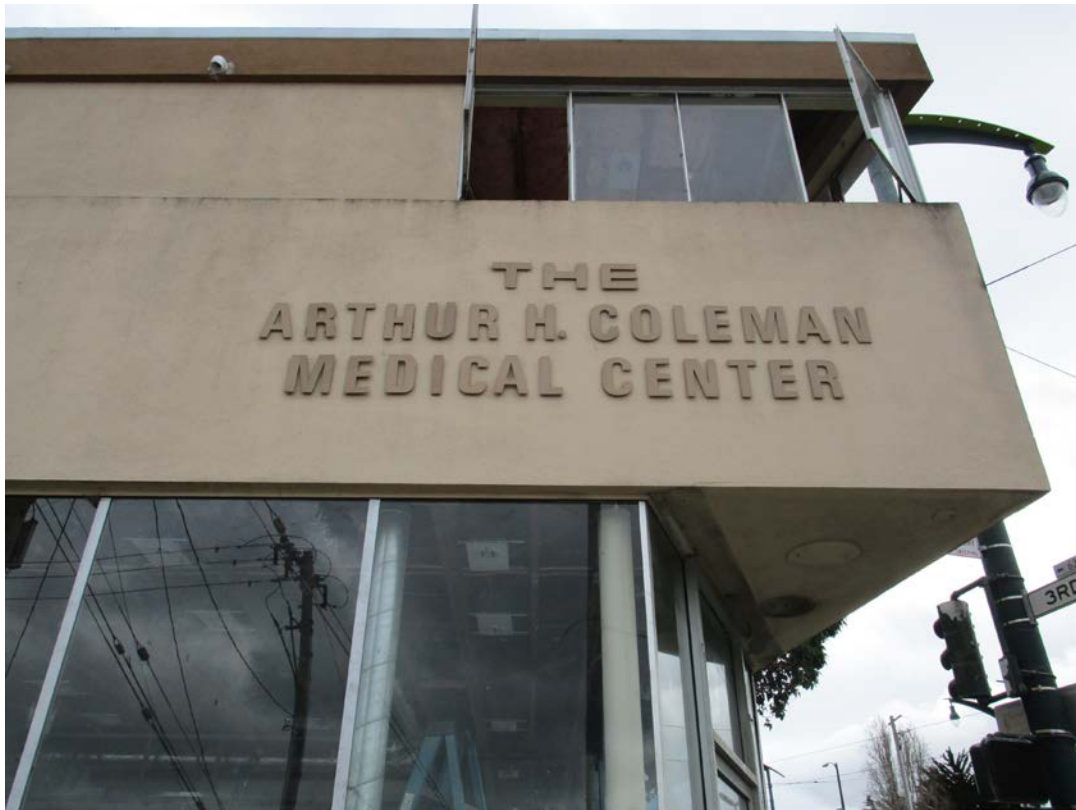
Detail of sign on north (Ingerson Avenue) elevation, view south.
