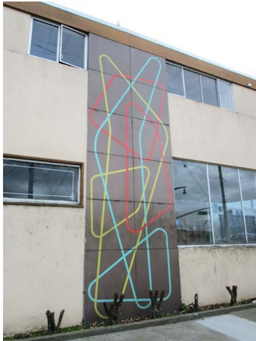
Detail of Porcelain enameled steel panel on north (Ingerson Avenue) elevation, view south.
