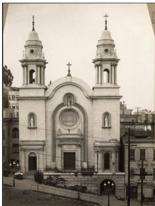
Our Lady of Guadalupe Church exterior showing original round window, circa 1912-1923. (Anne Cervantes/The Art Institute of Chicago, Archival Image Collection)
