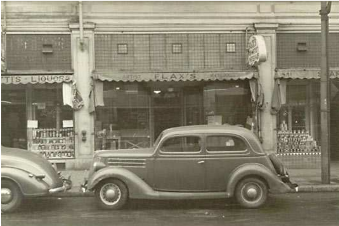
437 Kearny Street, the first FLAX location, 1938
