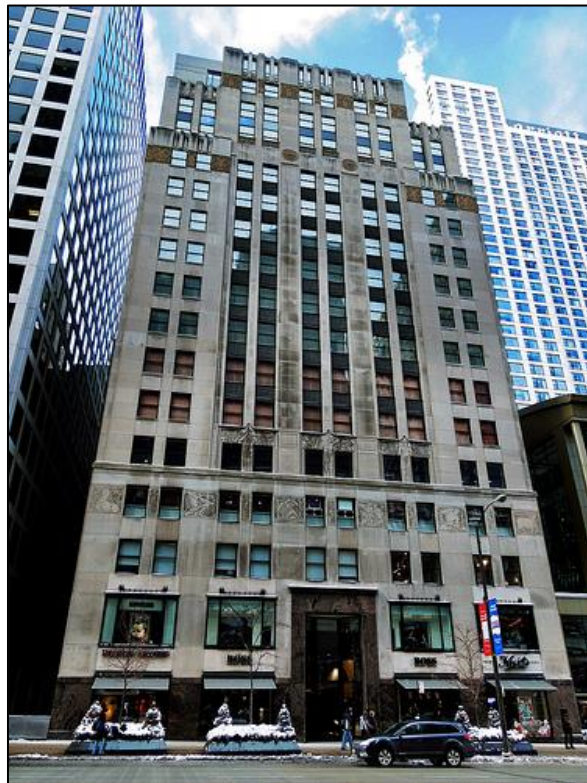
13. McGraw Hill Building, 520 N Michigan Avenue, Chicago II. Constructed 1929, altered 2000. (Image credit: https://www.flickr.com/photos/anomalous_a/6746339749 )
