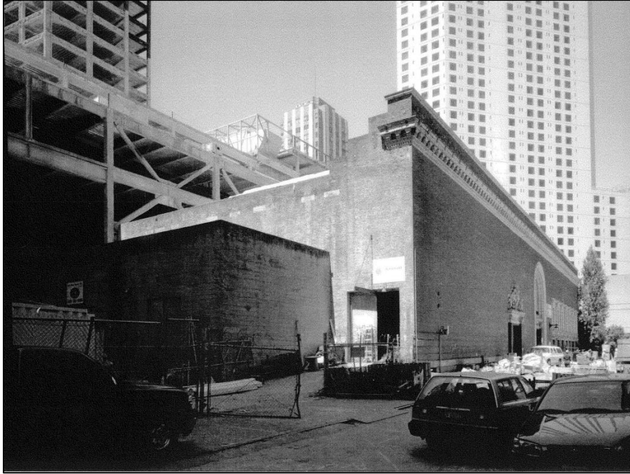
9. 736 Mission Street, before alterations (Image credit: SF Planning Department files)
