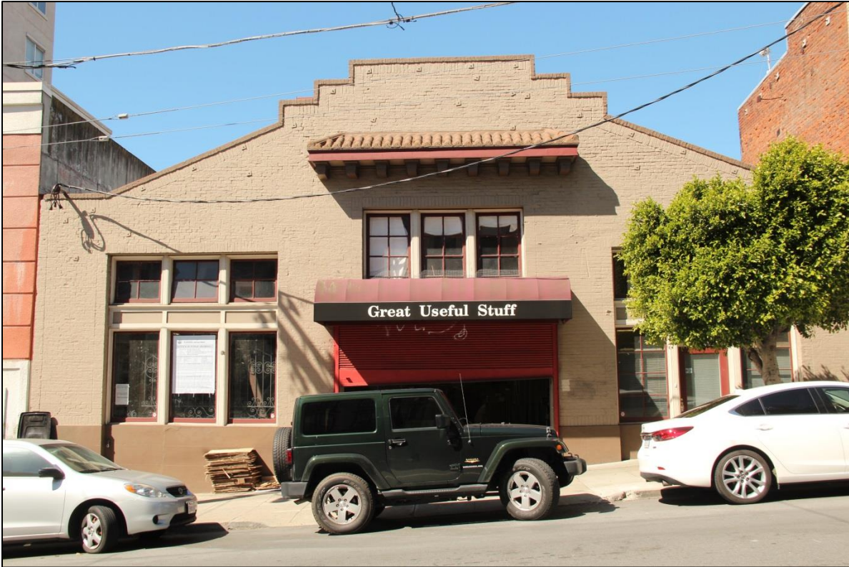
17. 1335 Larkin Street, current photo (Image credit: SF Planning Department)
