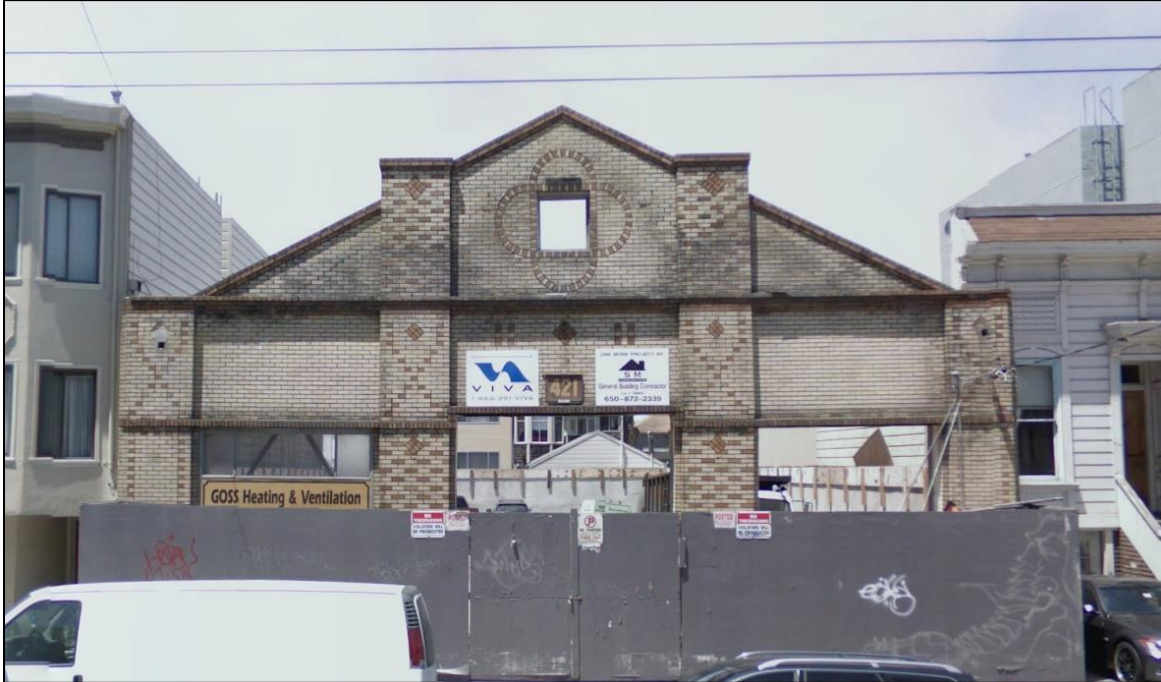
15. 421 Arguello Street, under construction (Image credit: Google street view)
