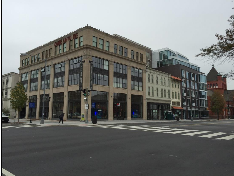
12. The Mission, 1625 14 th Street, NW, Washington D.C. Constructed late-nineteenth and early twentieth century, altered 2014. (Image credit: Tim Frye, SF Planning Department)
