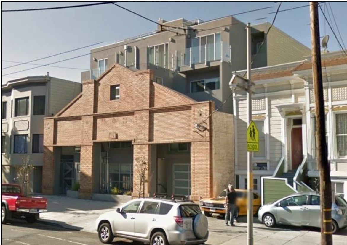
16. 421 Arguello Street, current photo (Image credit: Google street view)
