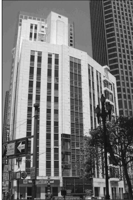
7. 690 Market Street, before removal of 1960s cladding (Image credit: SF City Guides)
