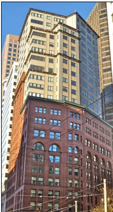
9. Chronicle Building, 690 Market Street, San Francisco, CA. Constructed 1890, altered 2003. (Image credit: https://en.wikipedia.org/wiki/Ritz-Carlton_Club_and_Residences#/media/File:Ritz-Carlton_Club_and_Residences,_San_Francisco.jpg )
