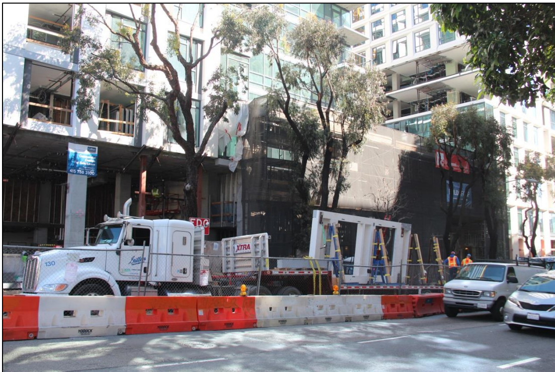
4. 1634 Pine Street, under construction (Image credit: SF Planning Department)
