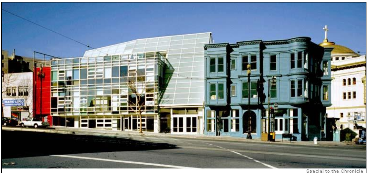
12. 1800 Market Street, after renovation (Image credit: http://imgs.sfgate.com/inline/c/pxs/2004/04/11/cm_lgbt-3.jpg )
