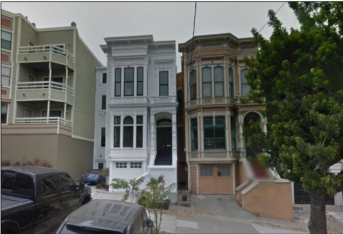
21. 15 Baker Street, current photo (Image credit: Google street view)
