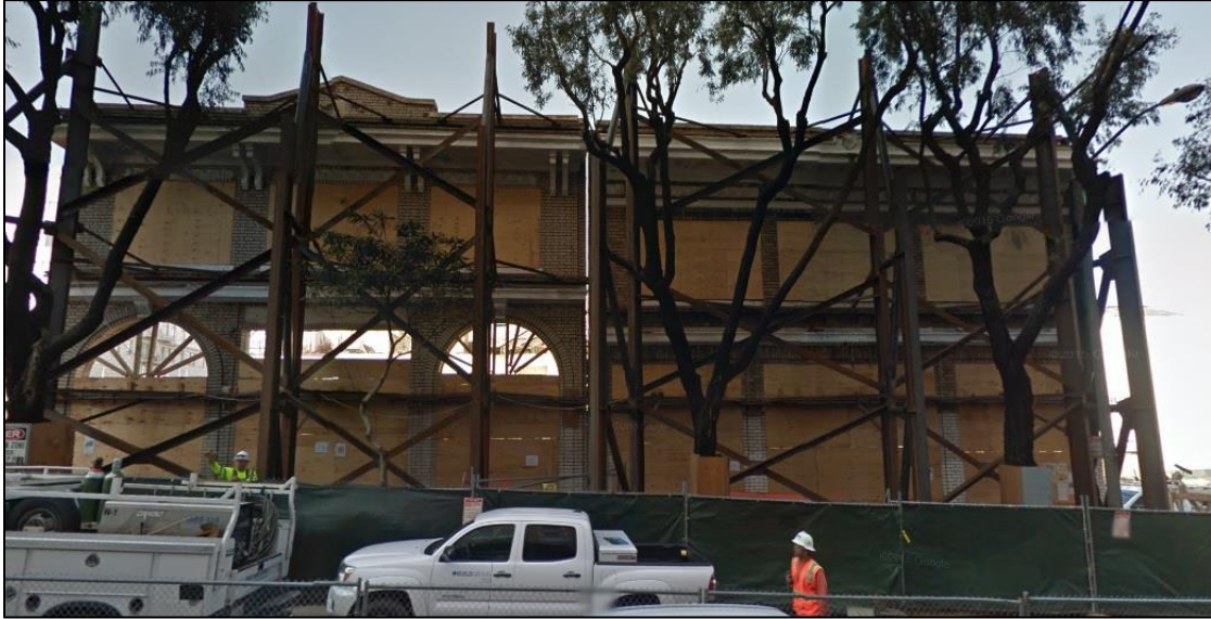
3. 1634 Pine Street, under construction (Image credit: Google street view)
