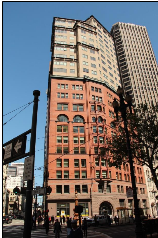
8. 690 Market Street, current photo (Image Credit: SF Planning Department)
