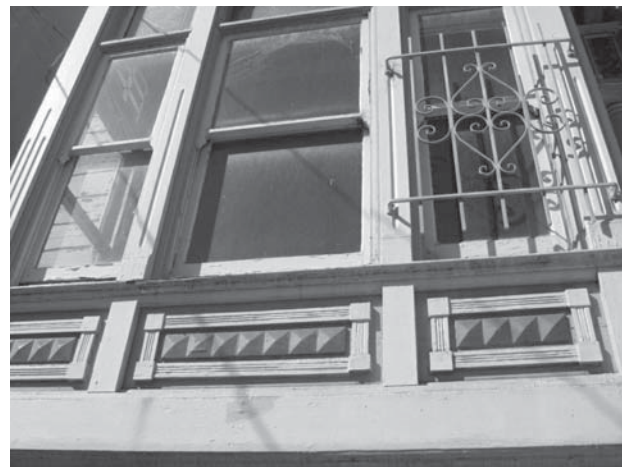
EXISTING WINDOW TRIM
