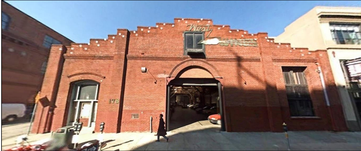
13. 178 Townsend Street, before alterations (Image credit: Google street view)
