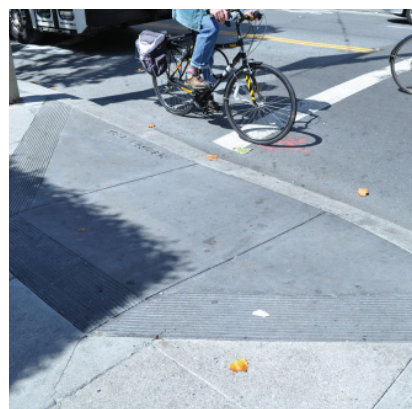
Curb ramp at McAllister and Hyde Streets
