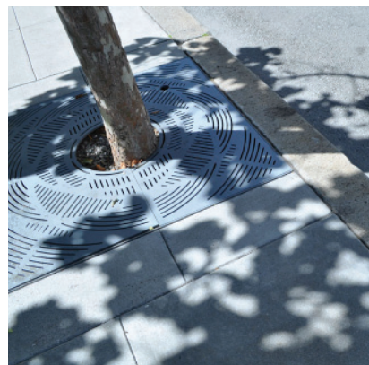
Square metal tree grate along McAllister St
