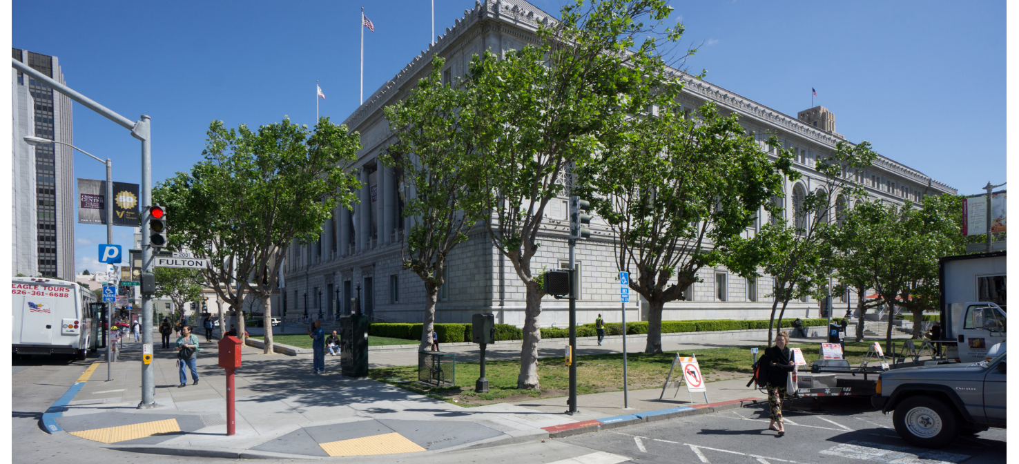
VIEW OF SITE LOOKING NORTHEAST
