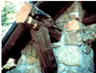
An inert material was injected into the hollow outrigger, permitting the outer wood to be retained and preserved.
