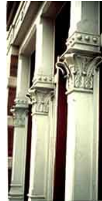
Cast aluminum has been used as a replacement material for cast iron. Photo: NPS files.
