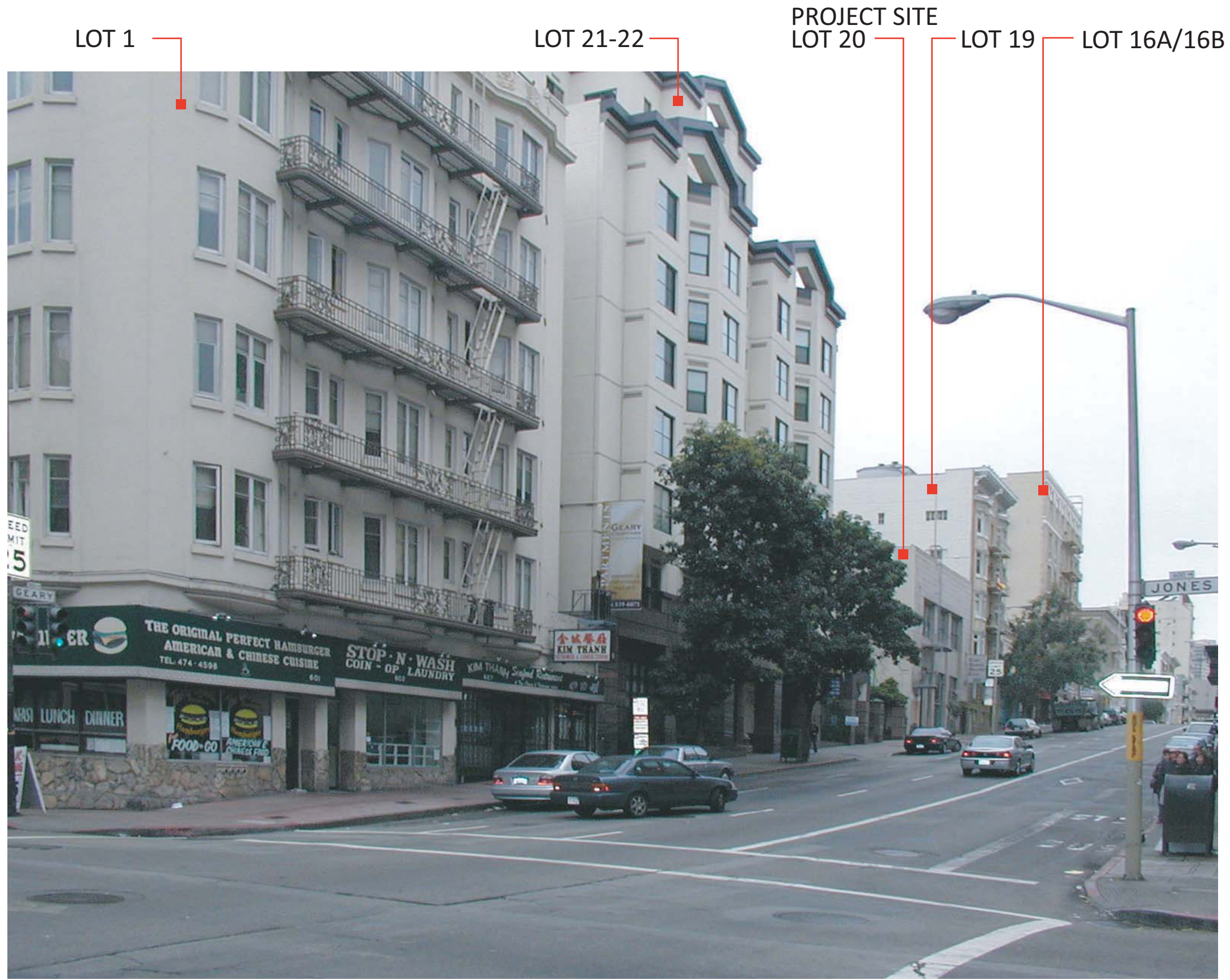
GEARY STREET FRONTAGE - LOOKING SOUTHWEST BLOCK 318
