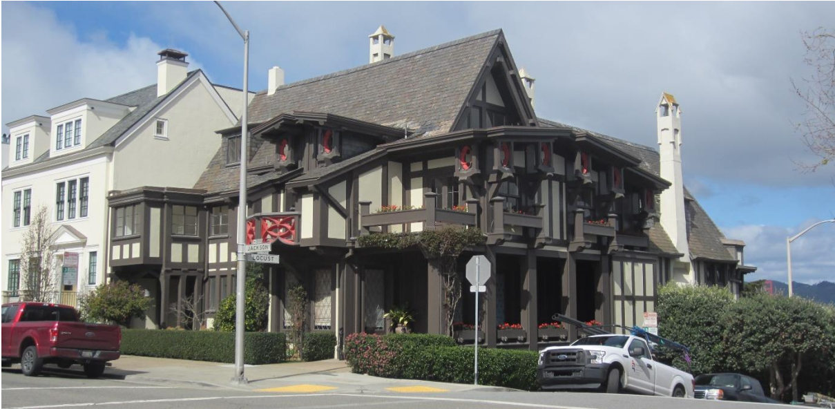
Photo 1. 3500 Jackson Street, view northwest.
