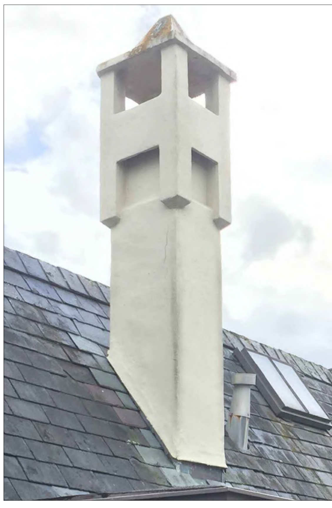
6 EXISTING CHIMNEY PHOTO SCALE: NTS
