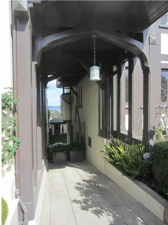
Photo 3. Detail of carriageway, view north.
