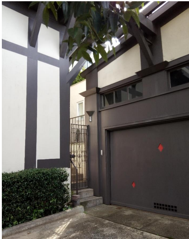
Photo 6. Detail of northwest corner of house and garage, view southwest.
