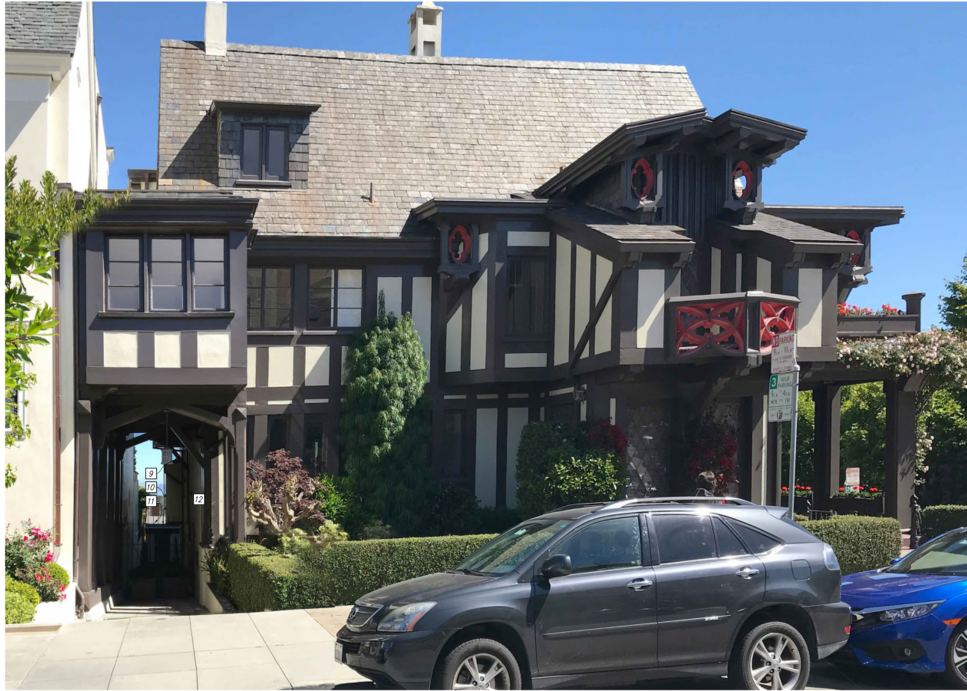
5 PHOTO: EXISTING CARRIAGEWAY SCALE: N/S
