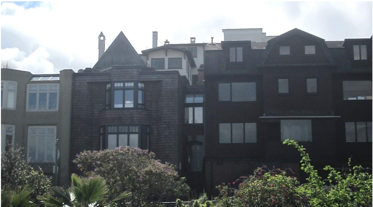
Photo 8. North elevation, view south from the Presidio.
