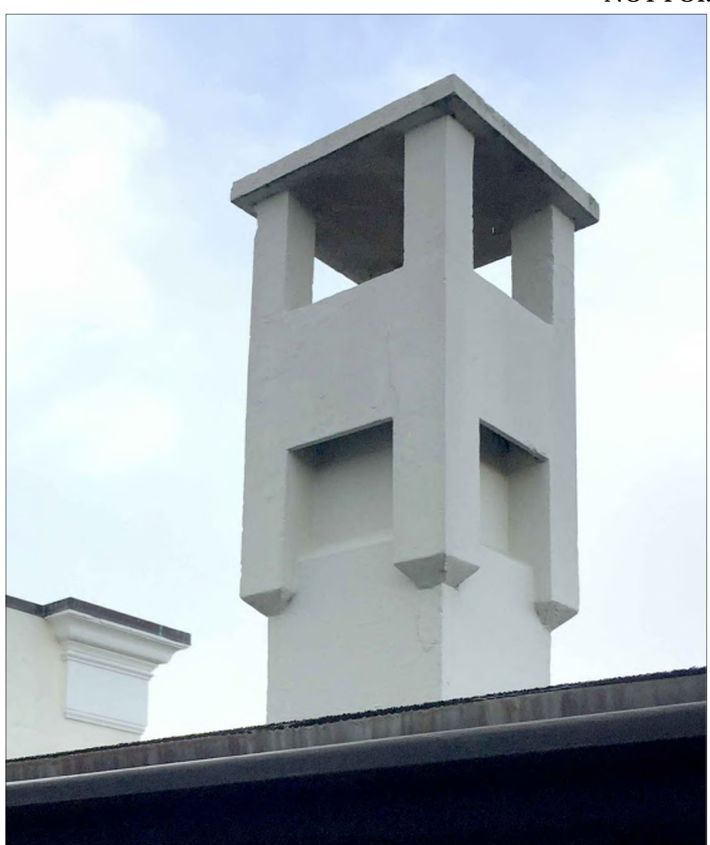
6 EXISTING CHIMNEY PHOTO SCALE: NTS
