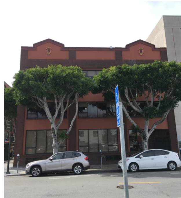
FRAME AND INFILL WITHIN DISTRICT 100-120 Broadway
