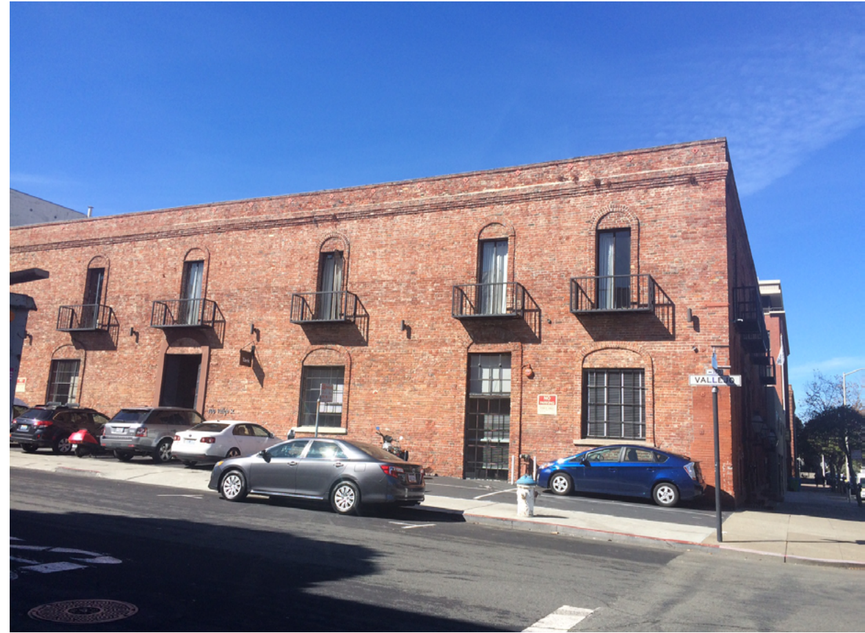
BALCONIES EXAMPLE WITHIN DISTRICT 915 Front Street (Balconies later addition)
