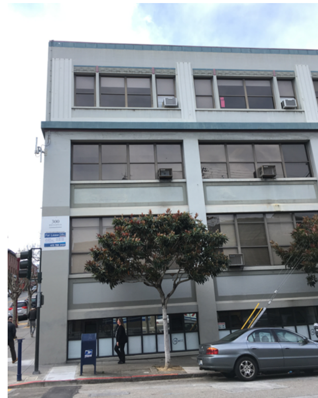
FRAME AND INFILL WITHIN DISTRICT 300 Broadway
