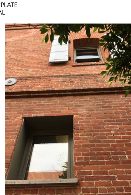
WINDOW OFFSETS WITHIN DISTRICT 1 Union Street
