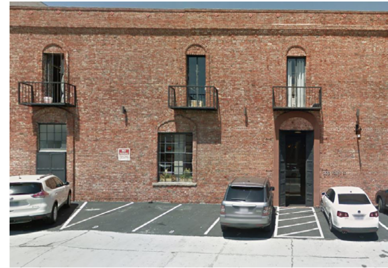
OFFSET WINDOWS EXAMPLE WITHIN DISTRICT 915 Front St
