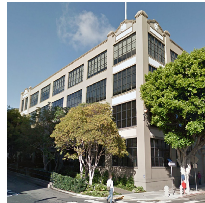
FRAME AND INFILL WITHIN DISTRICT 901 Battery St.
