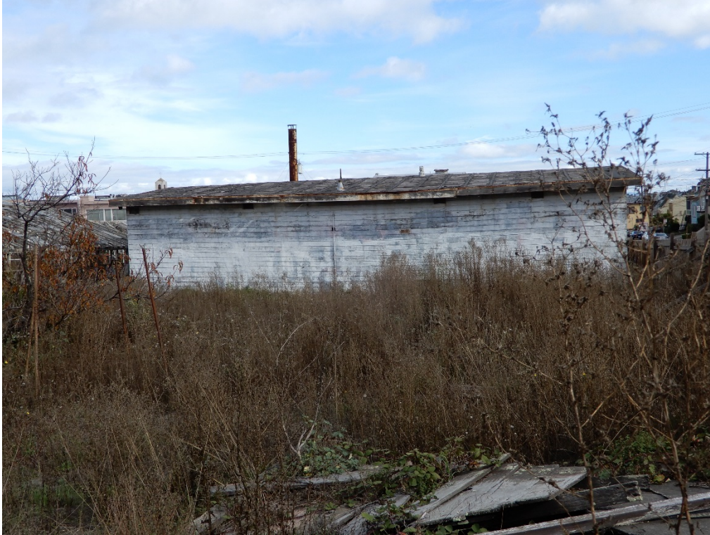
Figure 14. Office building, west façade, view facing east.
