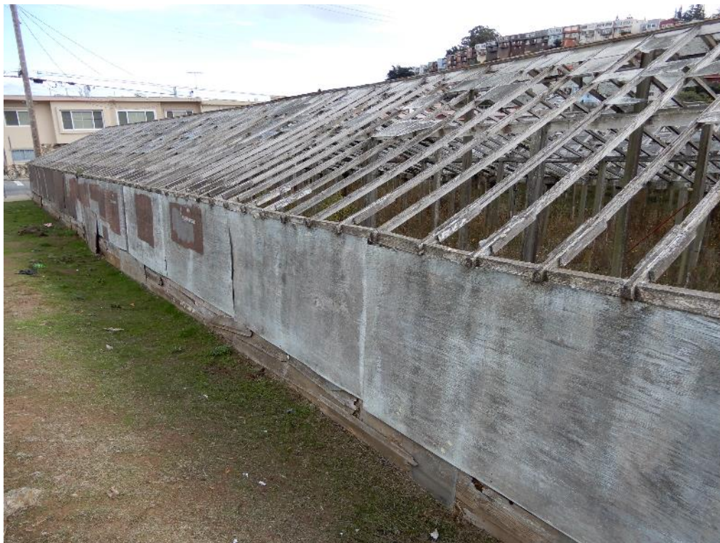
Figure 10. North side of greenhouse at Wayland Street, view facing southeast.
