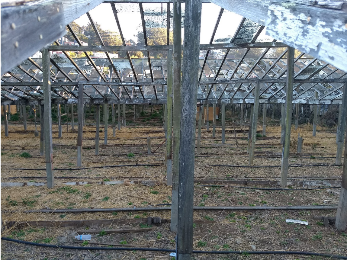
Figure 7. Typical interior of ridge-and-furrow style greenhouses, showing planting beds.
