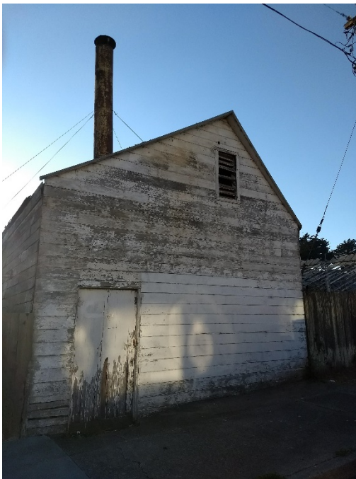
Figure 11. Boiler house, primary (east) façade, view facing northwest.
