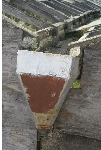
Figure 9. Box gutter and cap.
