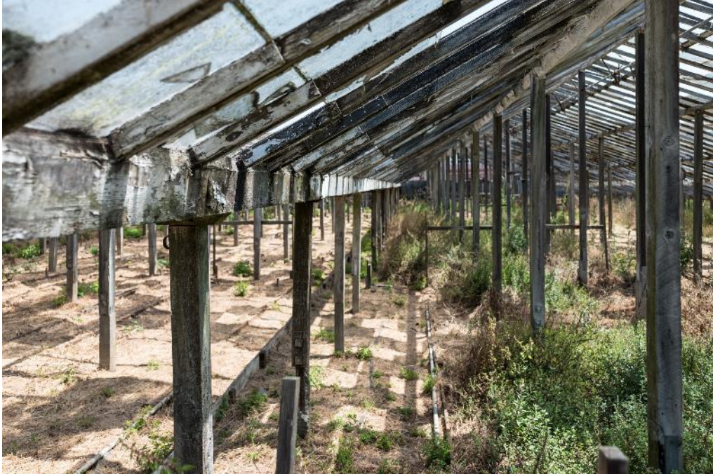
Figure 5. Ridge-and-furrow-style greenhouse, typical interior. Courtesy of Christopher Michel Photography.
