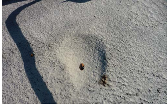
Figure 5. Hole at one bubble near northwest corner.
