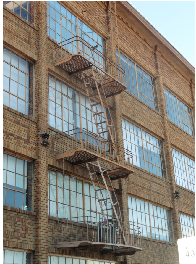
Figure 1. Metal fire escape at south elevation.
