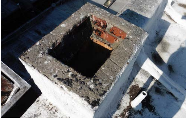
Figure 2. Open ventilation stack on north wall; cover with sheet metal as needed.
