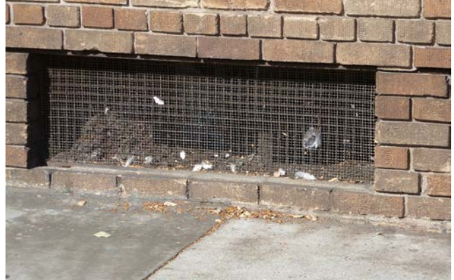
Figure 1. Ventilation grilles; note 1"x 1" historic iron grille.
