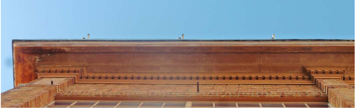
Figure 2. Cornice along west; note discoloration and localized corrosion, conditions are considered typical.
