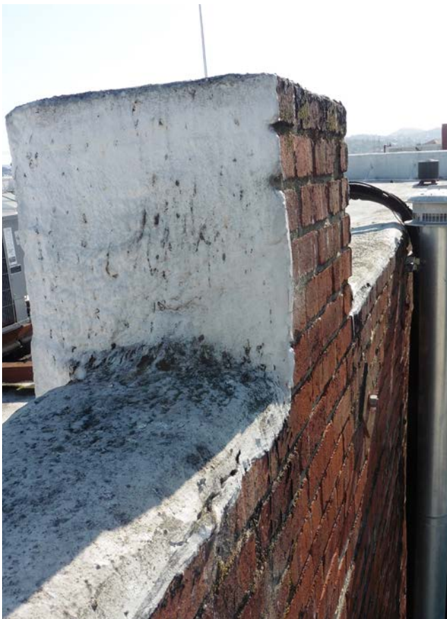
Figure 3. Unbraced ventilation stack at north wall.
