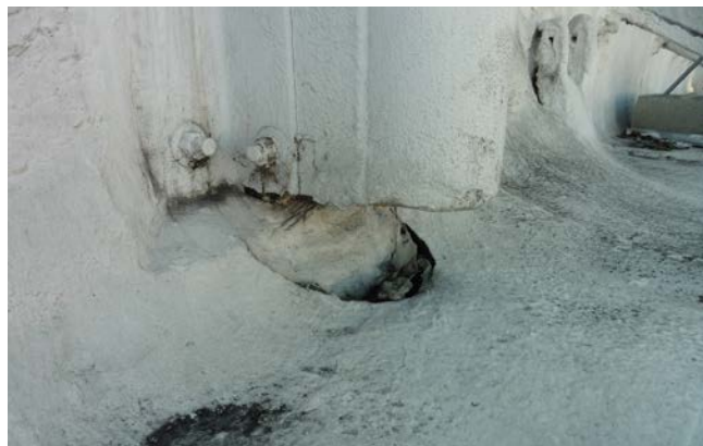
Figure 3. Detail of flagpole anchor; note corrosion and damage to roofing, even after re-roofing.
