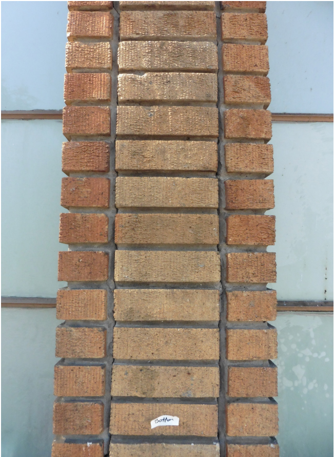
Figure 1. Typical brick pier; note mortar coloring and condition; deep recessed joint to be maintained.
