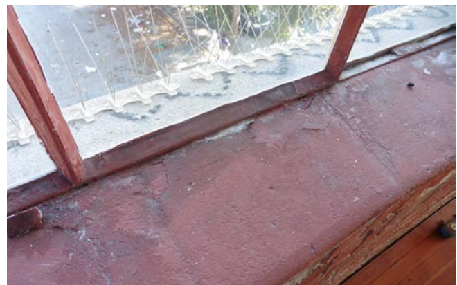
Figure 2: Concrete parge at south window sills, typical. Note level of localized cracking and paint deterioration.
