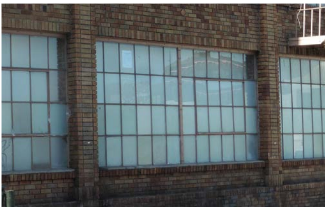
Figure 4. Typical multi-light steel windows at grade.
