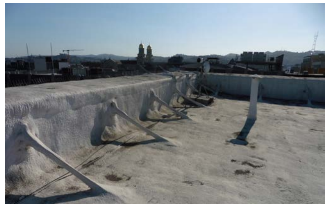
Figure 3. Parapet with bracing, typical.
