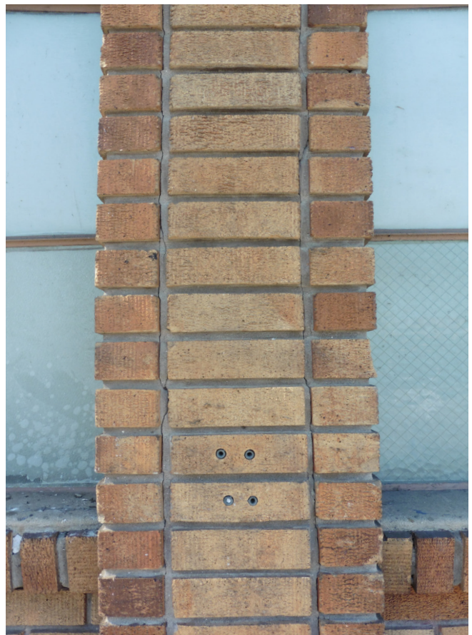
Figure 5. Typical condition of brick at south & west walls, clean all surfaces prior to further rehabilitation work.
