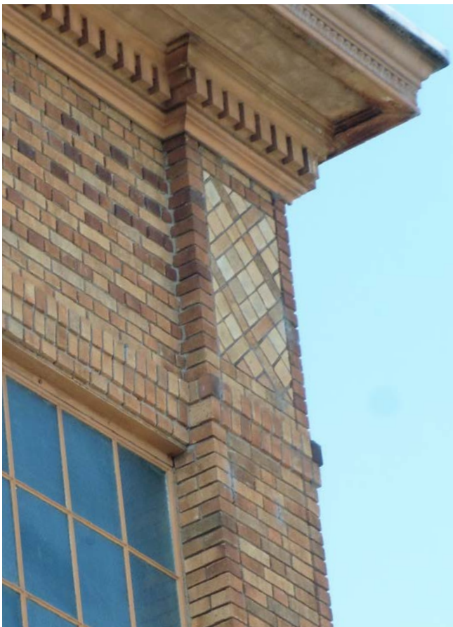
Figure 3. Southeast Corner; note decorative patterning and general brick pattern of elevation.
