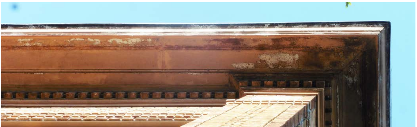
Figure 3. Cornice at southwest corner; localized areas of severe damage observed & requiring immediate repair.
