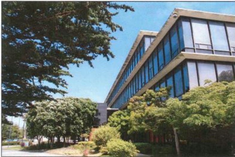
Continuous full-height, slightly recessed curtain wall glazing on most sides and along all levels of the building
