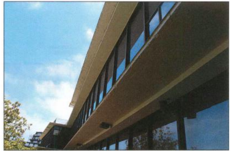
Flat, cantilevered roof with projecting eaves
