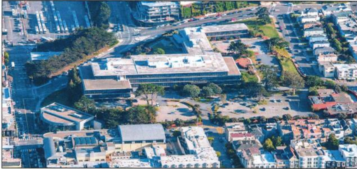
Corporate campus setting featuring an office building located on a large, open landscaped site across 10.25 acres
