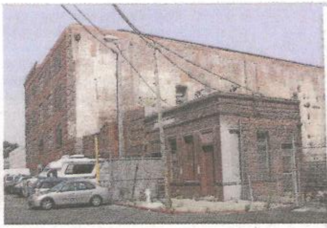
Station A, south end, west wall as seen from 23rd Street. The south portion is more structurally sound than the north.
