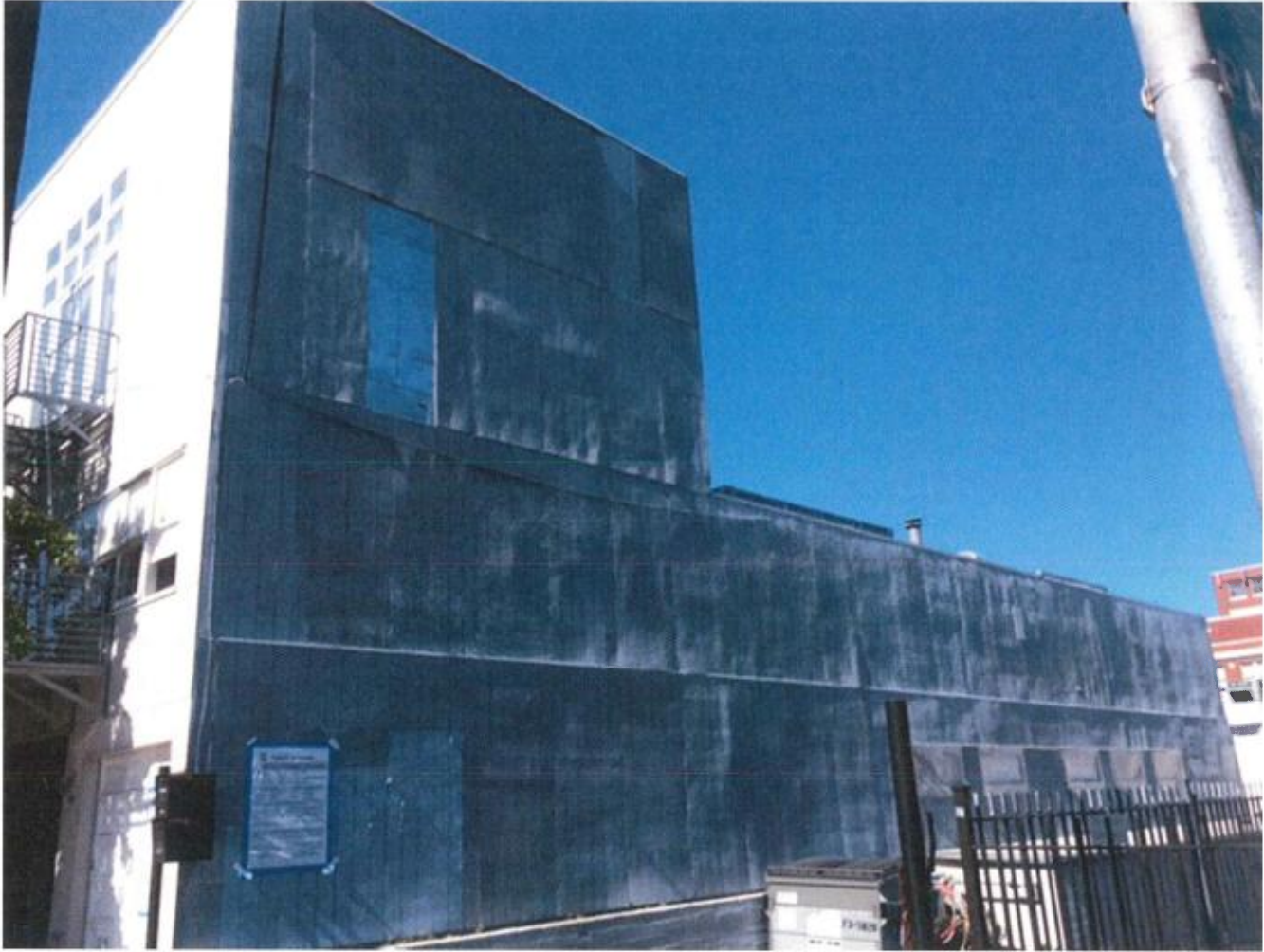
(1) South wall 1001 Tennessee Street.
