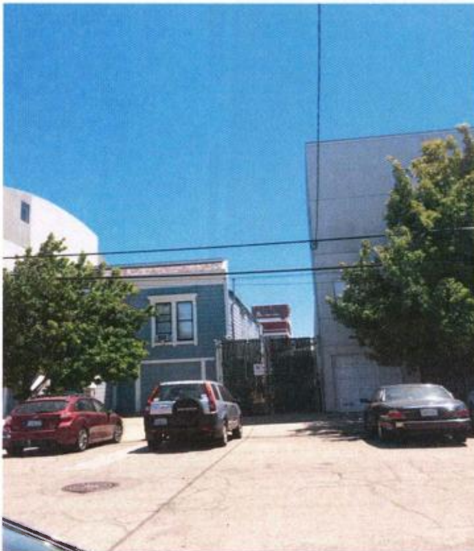
997-999 Tennessee Street with adjacent buildings that were built or modified prior to the enactment of the Dogpatch Historic District.
