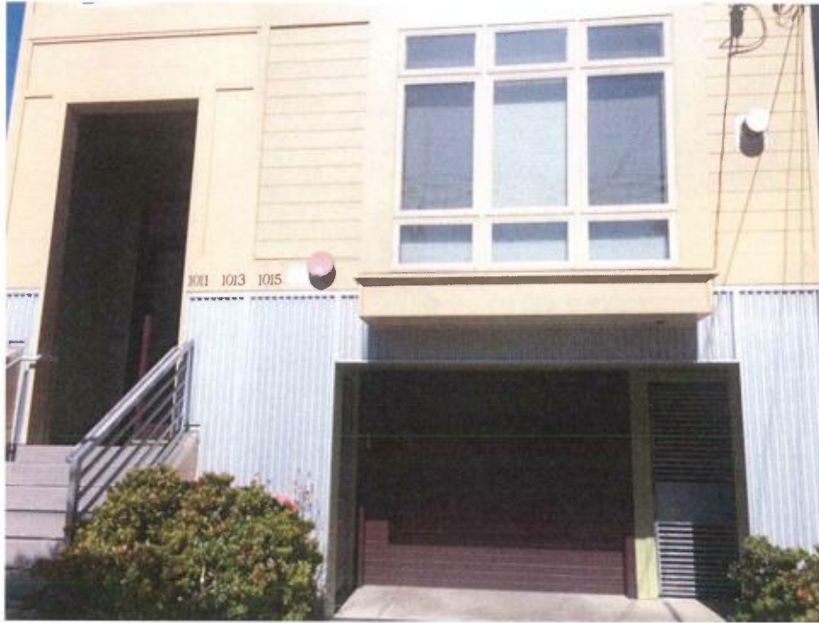
1011 Tennessee Street Façade
