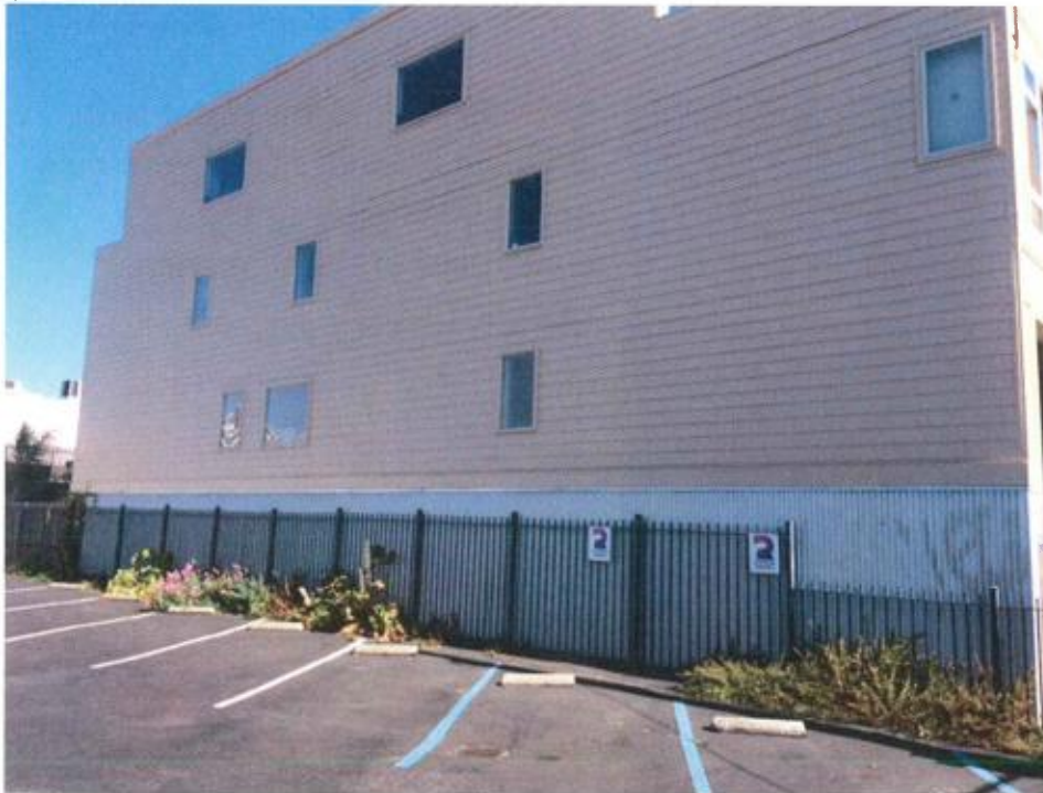
1011 Tennessee Street North Wall.
