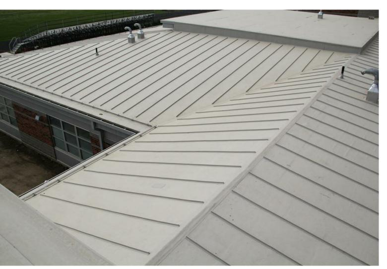
PVC ROOFING WITH CONTOUR RIBS
