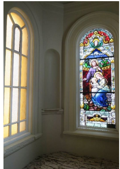
Entry room at southeast corner. (Page & Turnbull)
