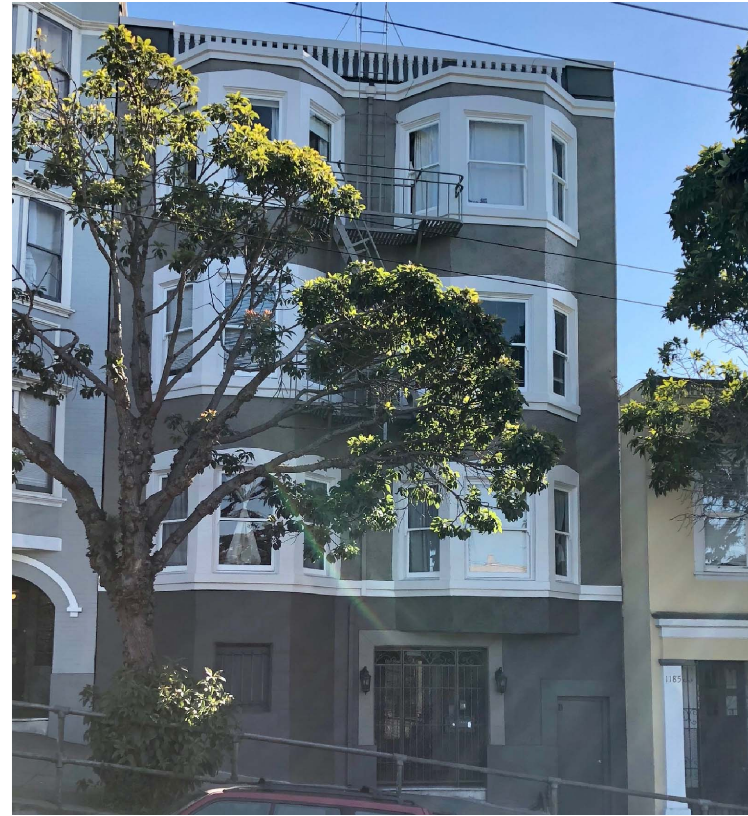
4 Existing Building Front Elevation
