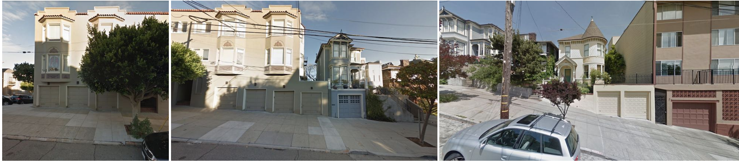
STREET LEVEL VIEW OF BUILDINGS ON EAST SIDE OF FAIR OAKS ST
