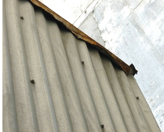
(Left) Figure 9. Older metal panels encapsulated by newer panels, visible from the building interior, are severely deteriorated. (Right) Figure 10. Existing flashing showing severe corrosion and deformation.
