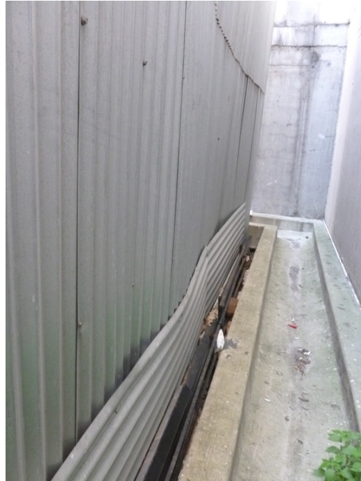
(Left) Figure 13. First area of deformation with gap up to 2" in depth. (Right) Figure 14. Second area of deformation near south end of wall. Note undulation of metal wall panels.
