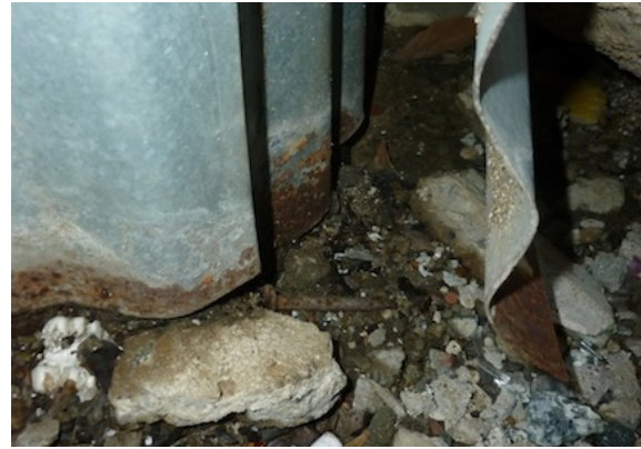
(Left) Figure 15. Puncture at metal panel on west elevation wall. (Right) Figure 16. Base of a metal panel at the southwest corner. Note corrosion caused by contact with grade.
