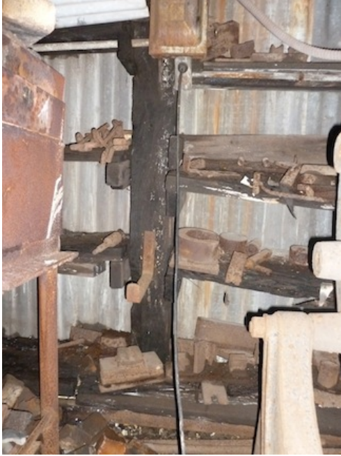
(Left) Figure 39. Grease stains by machine oil at wood post. (Right) Figure 40. Missing areas at wood post by mechanical removal (cutting).
