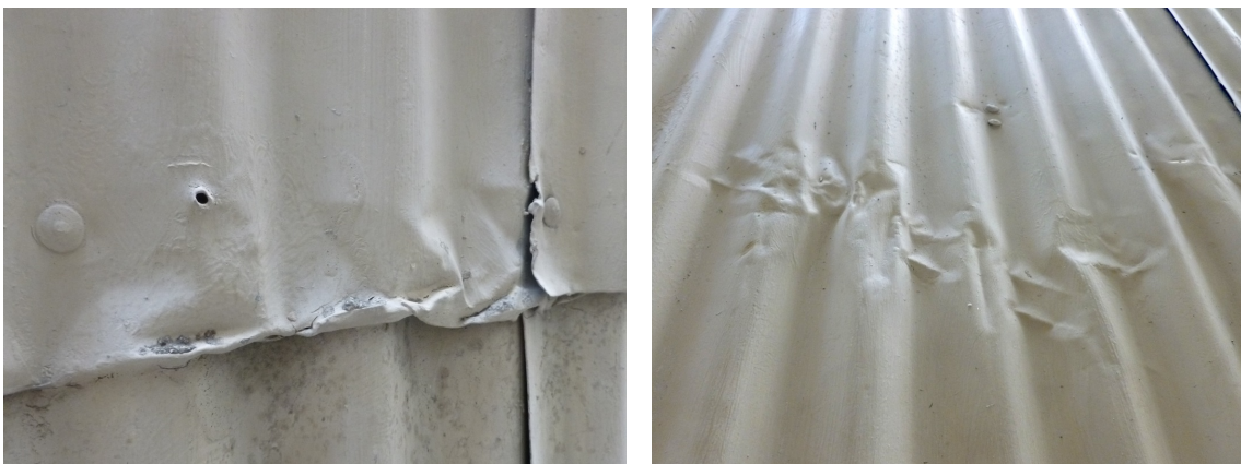
(Left) Figure 23. Example of existing holes from where previous fasteners were installed. (Right) Figure 24. Example of typical damage (dents) found on surface of east elevation wall panels.
