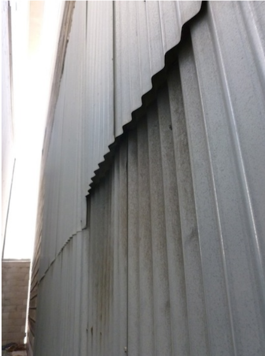
(Left) Figure 13. First area of deformation with gap up to 2" in depth. (Right) Figure 14. Second area of deformation near south end of wall. Note undulation of metal wall panels.
