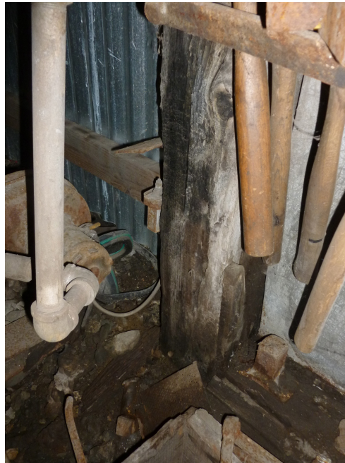
(Left) Figure 37. Wood post with split spanning its entire length. (Right) Figure 38. Wood post with smaller split at its base.
