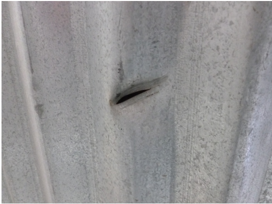
(Left) Figure 15. Puncture at metal panel on west elevation wall. (Right) Figure 16. Base of a metal panel at the southwest corner. Note corrosion caused by contact with grade.
