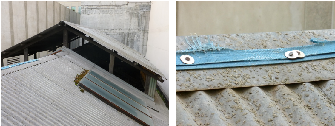
(Left) Figure 30. View of roof and central monitor. Note biological growth above skylight. (Right) Figure 31. Mortar splatter found on metal roof panels, as well as remnants of a blue tarp and fasteners.
