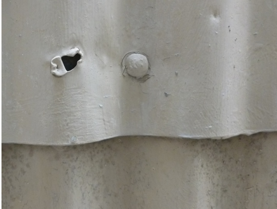
(Left) Figure 5. Example of an older fastener with rounded (cone-shaped) head. (Right) Figure 6. Example of a newer fastener with hexagonal bolt, washer and gasket.
