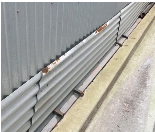
(Left) Figure 11. Smaller (horizontally laid) panels of corrugated metal at base of wall showing visible corrosion at tops of panels. (Right) Figure 12. Severely deteriorated metal track found along base of west elevation wall.
