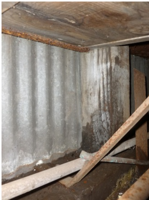
(Left) Figure 41. Staining by moisture infiltration at wood post base and sill plate below. (Right) Figure 42. Biological growth found near base of wood post on east elevation wall.
