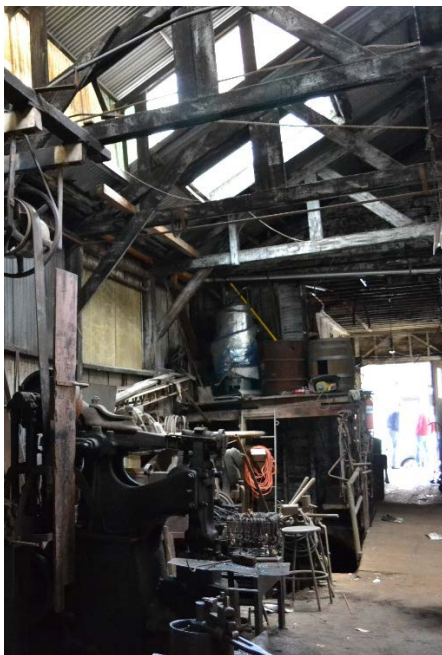
Figure 17. Interior walls and exposed roof trusses within the rear shed
