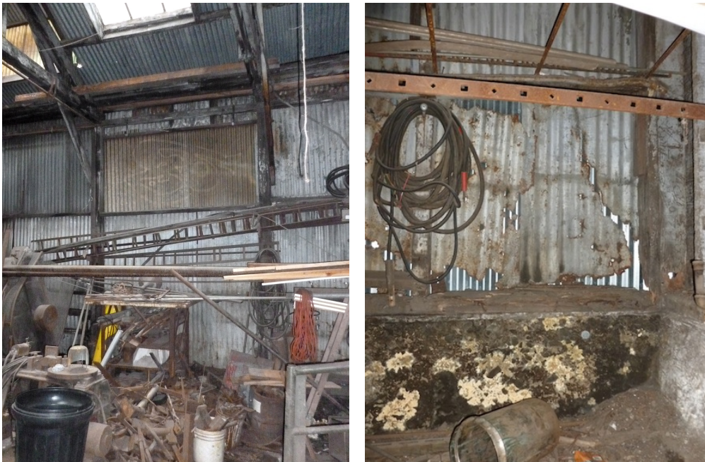
(Left) Figure 43. Equipment and material in front of wood posts made most inaccessible during survey. (Right) Figure 44. Northernmost bay of west wall showing the encapsulated and deteriorated older metal panels, poor condition of wood sill plate, and severe extent of biological growth at concrete foundation.
