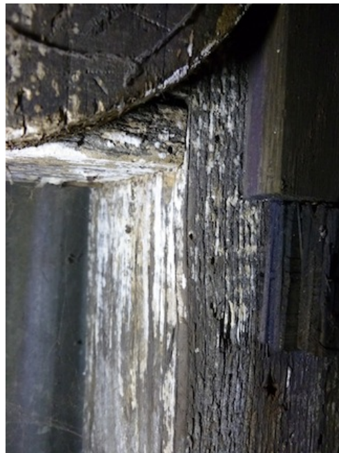
(Left) Figure 41. Staining by moisture infiltration at wood post base and sill plate below. (Right) Figure 42. Biological growth found near base of wood post on east elevation wall.
