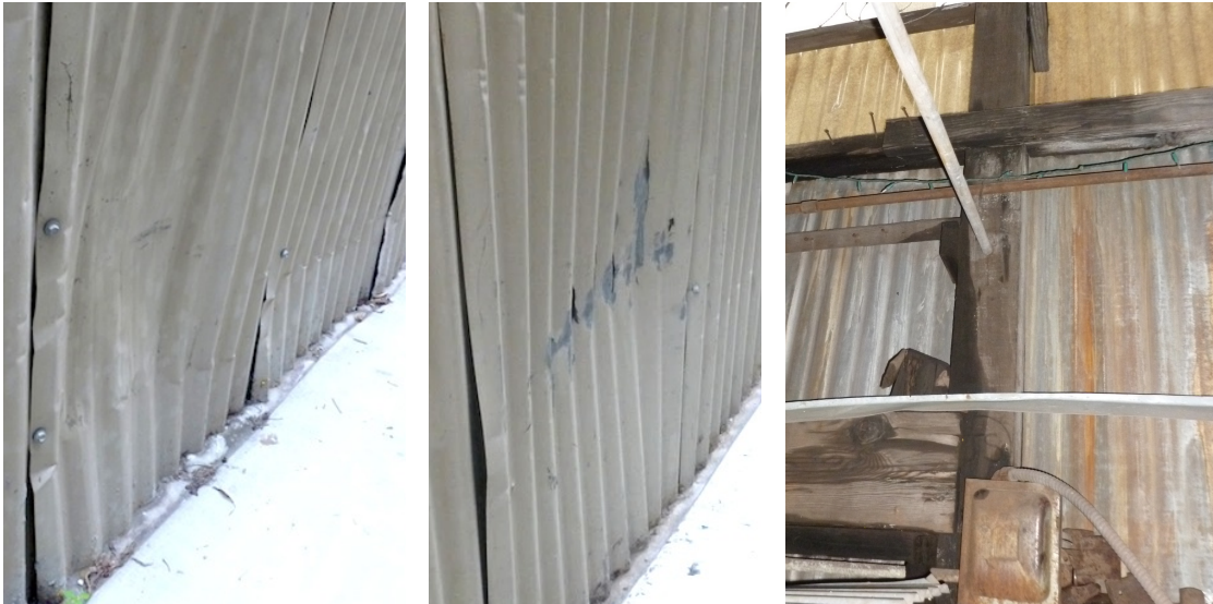
(Left and Center) Figures 25 & 26. Example of typical deformation (depression) and paint loss found along base of east elevation wall. (Right) Figure 27. Corrosion is visible on the backside of a metal panels.
