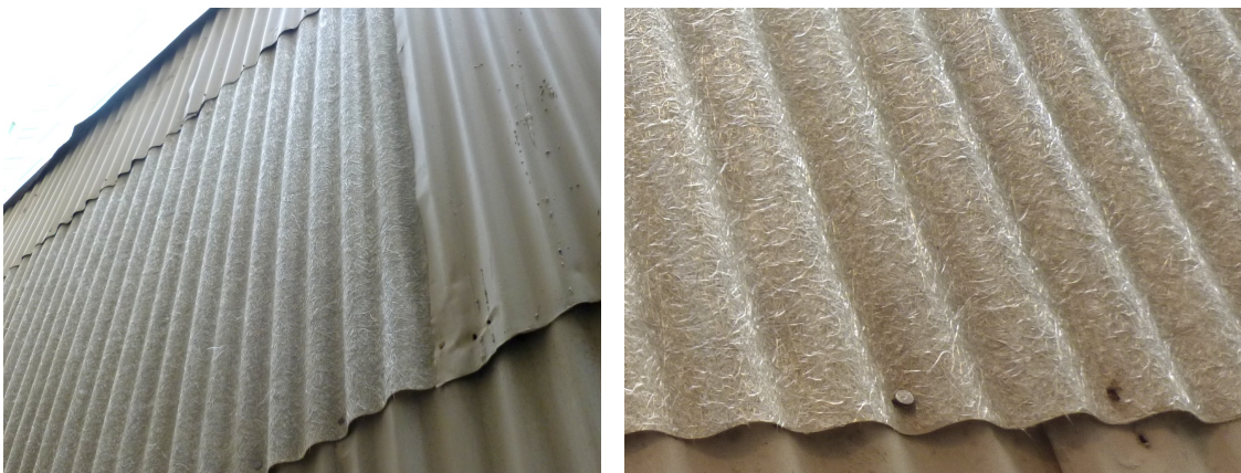
(Left) Figure 28. Example of fiberglass panel on the east elevation. (Right) Figure 29. Exposed glass fibers where resin coating has been lost.
