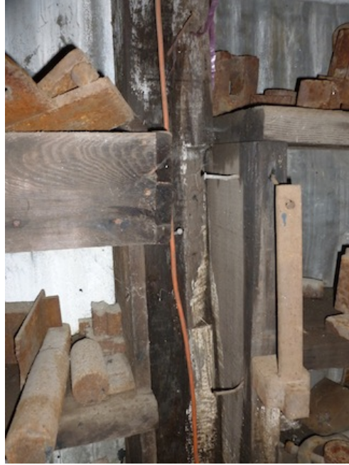
(Left) Figure 39. Grease stains by machine oil at wood post. (Right) Figure 40. Missing areas at wood post by mechanical removal (cutting).
