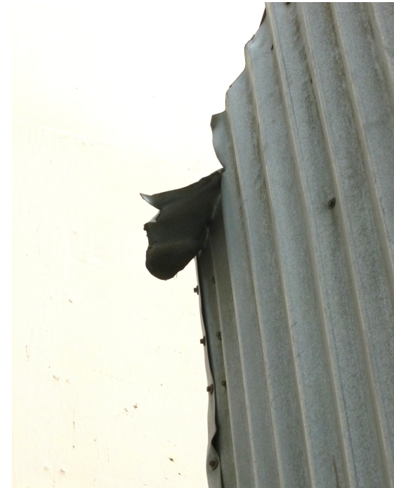
(Left) Figure 17. View of the south elevation gable end wall showing all three rows of corrugated metal panels. (Right) Figure 18. Make-shift scupper at the southwest corner.
