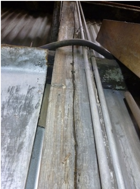
(Left) Figure 37. Wood post with split spanning its entire length. (Right) Figure 38. Wood post with smaller split at its base.
