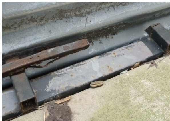
(Left) Figure 11. Smaller (horizontally laid) panels of corrugated metal at base of wall showing visible corrosion at tops of panels. (Right) Figure 12. Severely deteriorated metal track found along base of west elevation wall.
