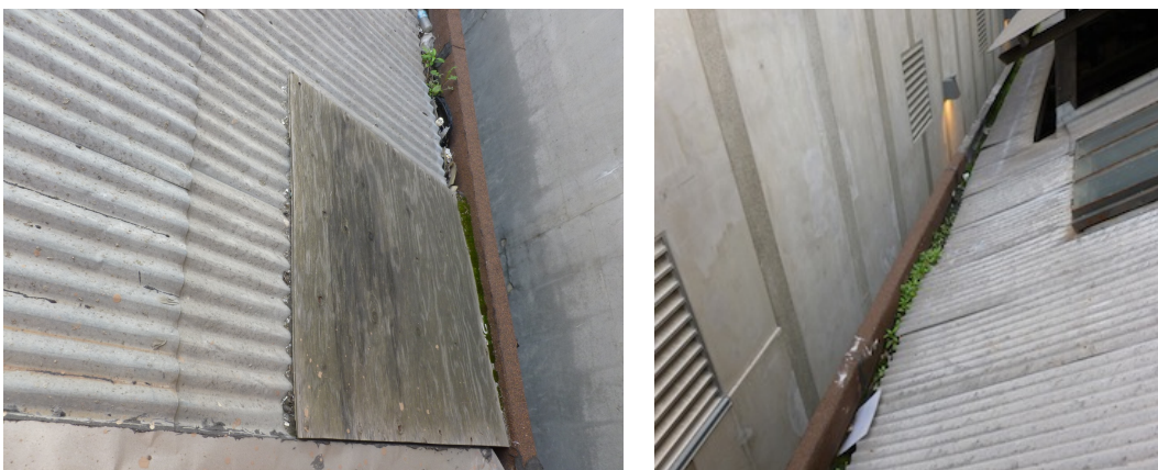
(Left) Figure 32. Plywood panel over metal panel on the northwest corner of roof. (Right) Figure 33. Gutters are filled with debris, plant and biological growth.
