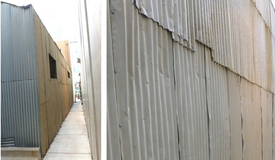
(Left) Figure 21. View of east elevation wall with painted corrugated metal panels. (Right) Figure 22. Photo shows metal and fiberglass panels of varying dimensions.
