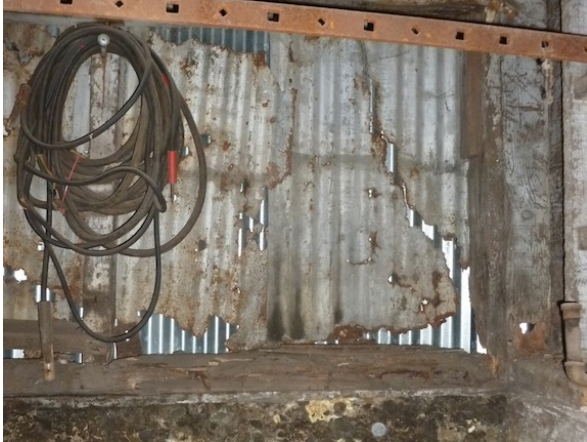
(Left) Figure 9. Older metal panels encapsulated by newer panels, visible from the building interior, are severely deteriorated. (Right) Figure 10. Existing flashing showing severe corrosion and deformation.
