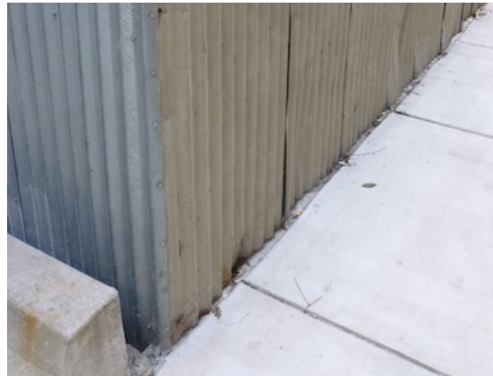
(Left) Figure 7. Concrete drain flanking west and south elevations. (Right) Figure 8. Painted metal panels on the east elevation terminate at concrete walk.
