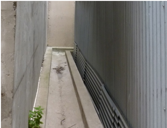
(Left) Figure 7. Concrete drain flanking west and south elevations. (Right) Figure 8. Painted metal panels on the east elevation terminate at concrete walk.
