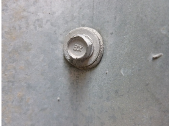
(Left) Figure 5. Example of an older fastener with rounded (cone-shaped) head. (Right) Figure 6. Example of a newer fastener with hexagonal bolt, washer and gasket.
