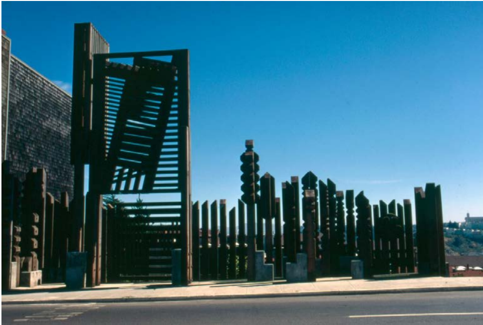
Newly constructed Diamond Heights Safety Wall, c. 1968. [SFPL – AAZ-0854]
