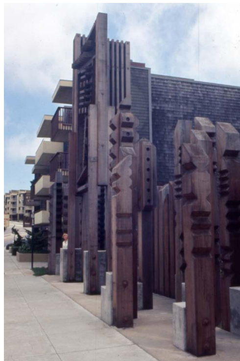
Diamond Heights Safety Wall (looking east) with Cohen & Levorsen-designed Red Rock Hill condominiums behind, c. 1968. [SFPL – AAZ-0856]
