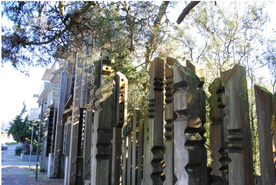
Detail of horizontal "wall" element (looking east).
