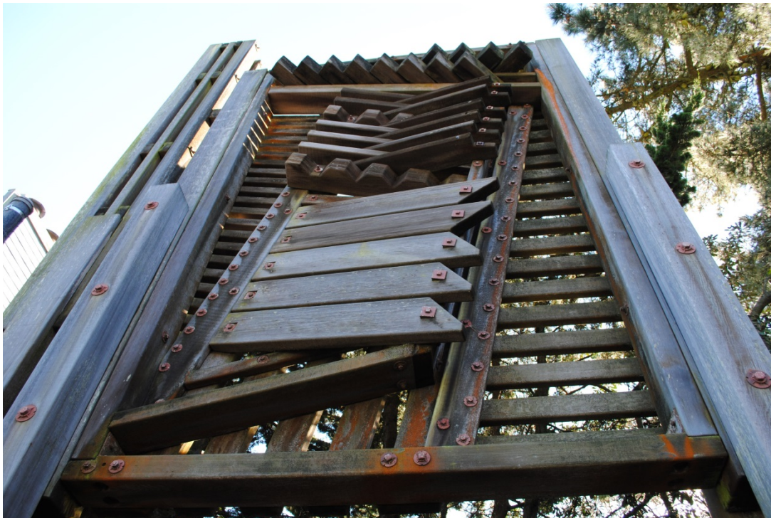
Detail of primary (north) façade.
