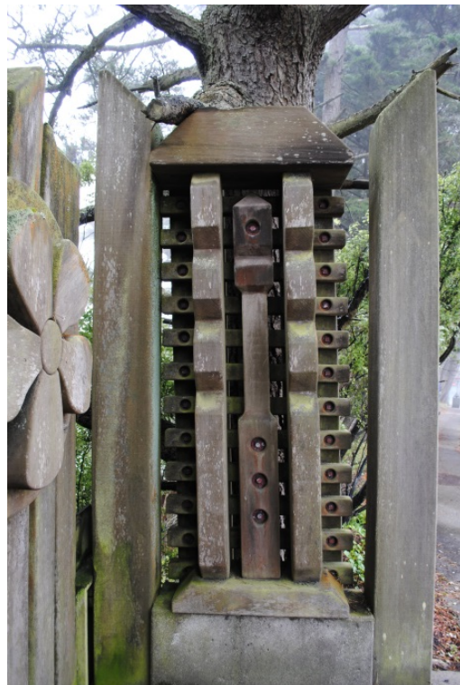
Physical encroachment of adjacent tree (west).
