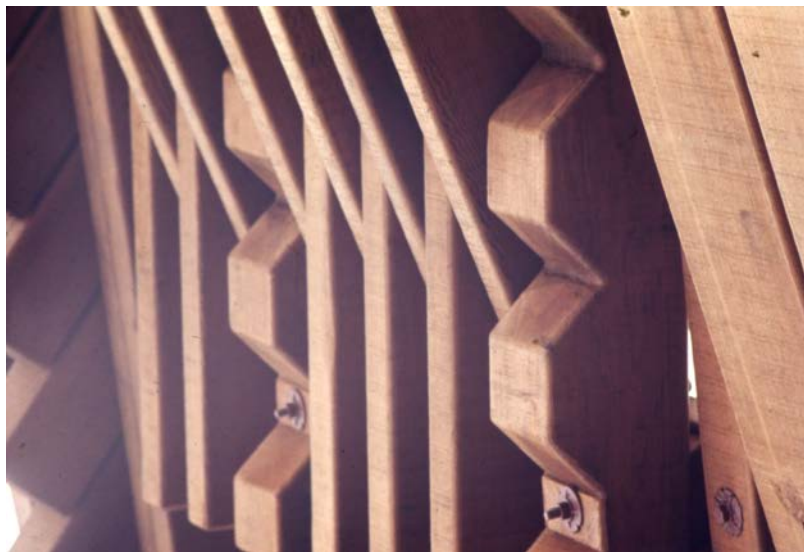
Detail of geometrically notched redwood elements and metal bolts, c. 1968. [SFPL – AAZ-0855]
