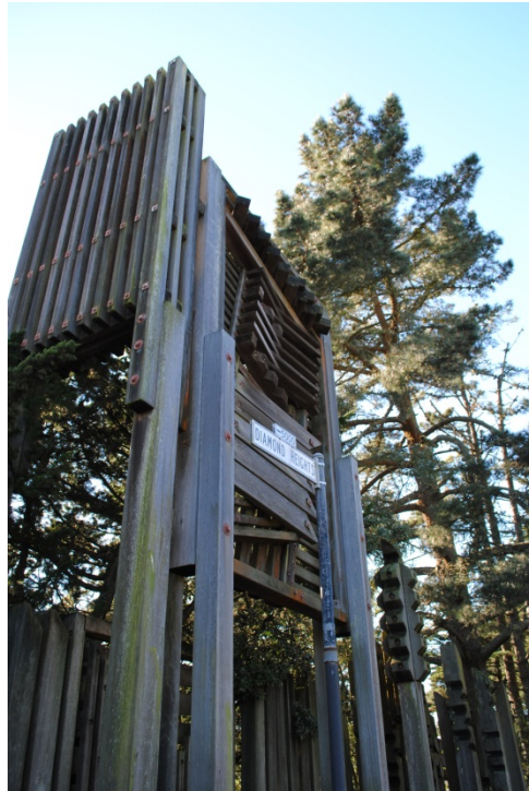
Oblique detail (looking southwest).
