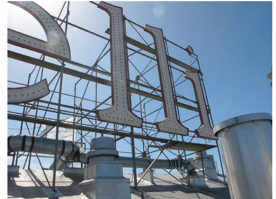
View of Ghirardelli sign, looking southwest
