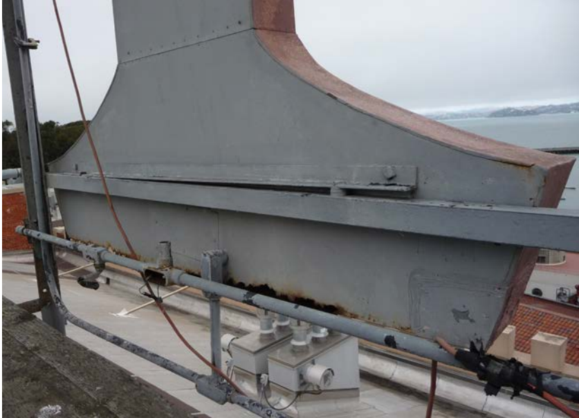
Figure 20 - A steel angle is bolted into the rear of each letter. This angle is then bolted to another steel angle which is bolted to the armature.
