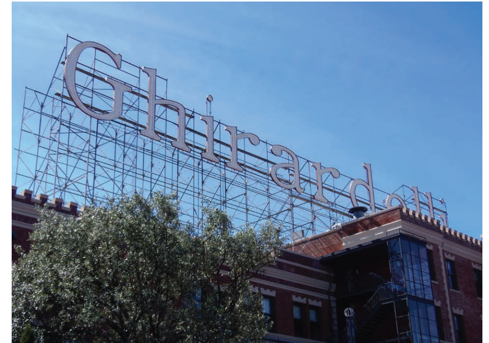
7. View of Ghirardelli Square facade along Polk Street, from the southwest corner of Polk and North Point Streets.
