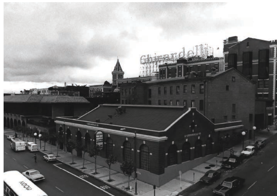
5. View of Beach Street and Polk Street facades, looking northwest, circa 1975 (Ghirardelli Square archives)
