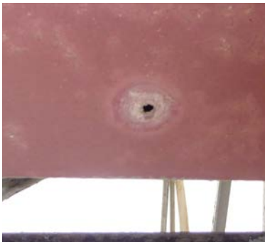
Figure 6 - Still operable weep hole with little deterioration
