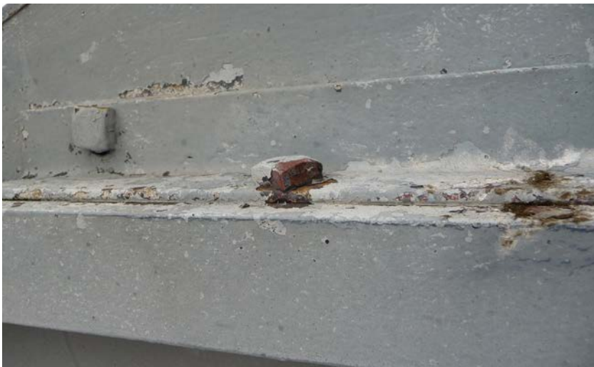
Figure 25 - The paint sample for the back of the letter came from the armature connection point at the rear of the last "i"
