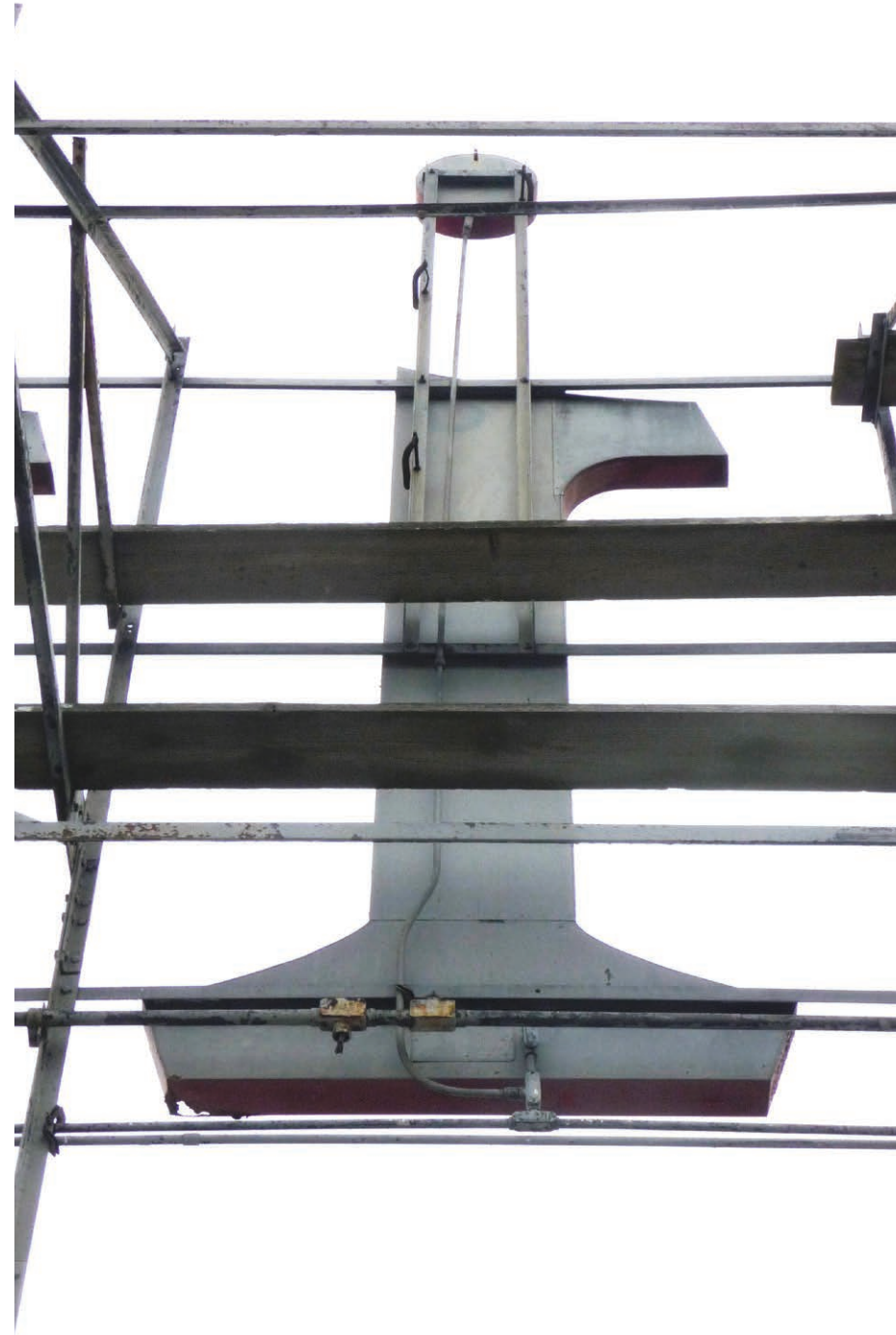
View of letter "i" mounted to steel truss frame, with scaffolding
