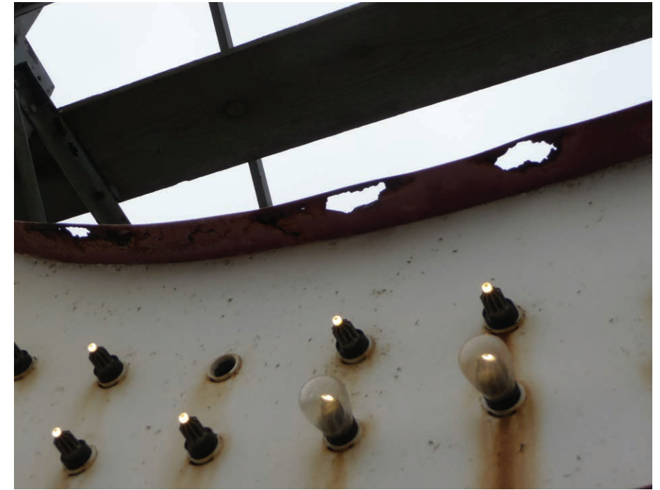
Close up of front side of letter showing corrosion and missing glass bulbs
