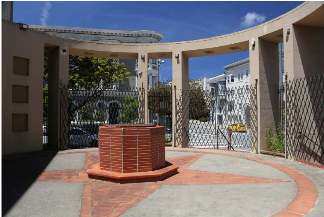
Octagonal baptismal font clad in long, narrow terracotta tile, and terracotta star inlaid in concrete platform at the main entrance. View northwest.
