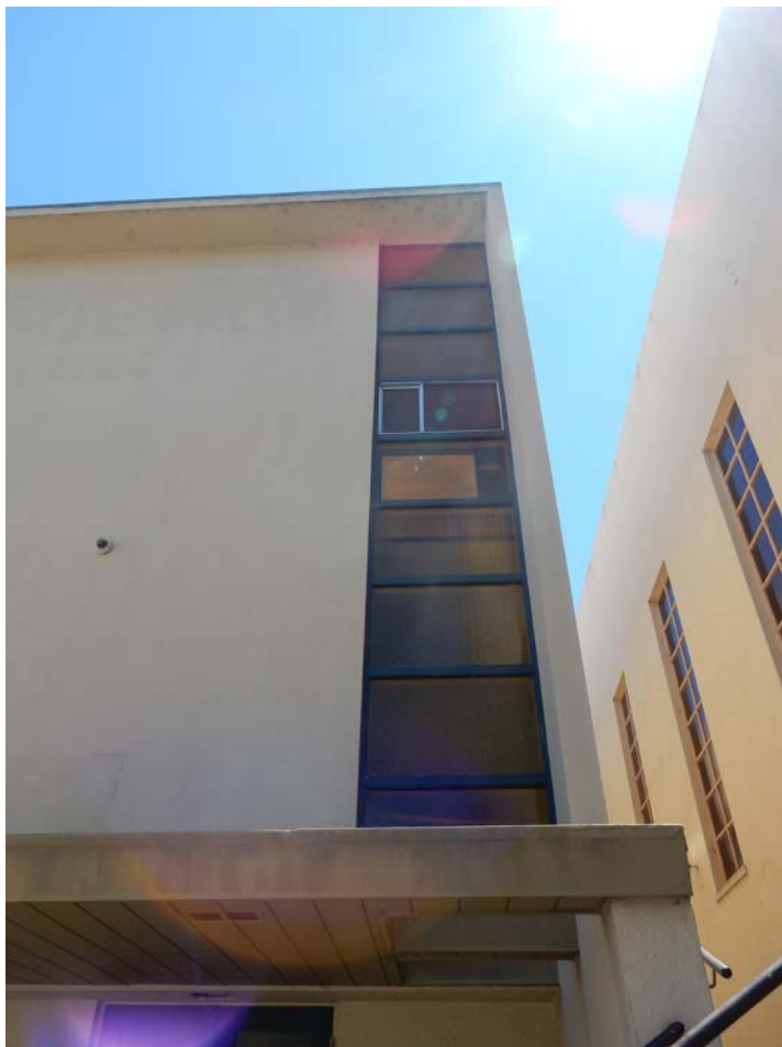
Vertical wood ribbon windows with textured yellow glass on north elevation of youth and classroom building, view south.
