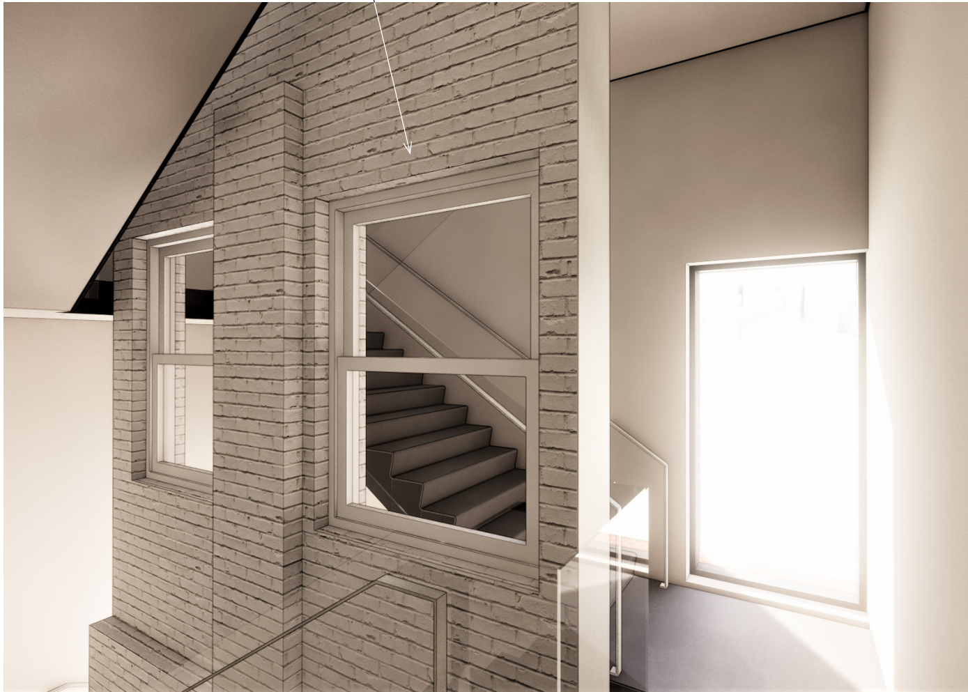
WEST STAIR THE EXISTING BRICK WALL AT THE WEST FACADE RE-MAINS IN-PLACE AND IS INTEGRATED INTO THE NEW WEST STAIR.
