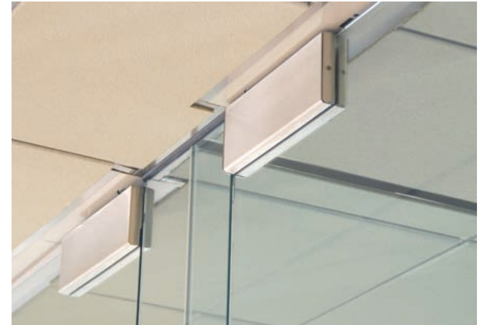
Patch fittings at top of proposed doors. Finish to match matte dark gray finish of metal canopy and cap
