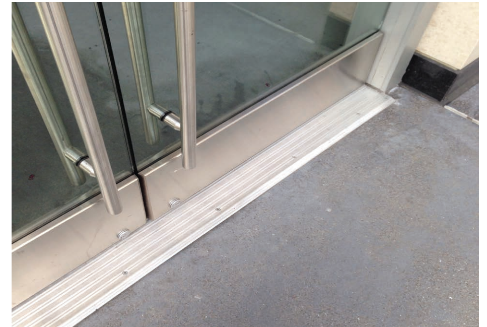
Brushed stainless steel door handle. Bottom door rail finish to match matte dark gray finish of metal canopy and cap
