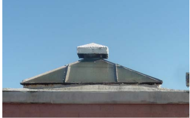
Figure 1. Roof & ventilator at penthouse.
