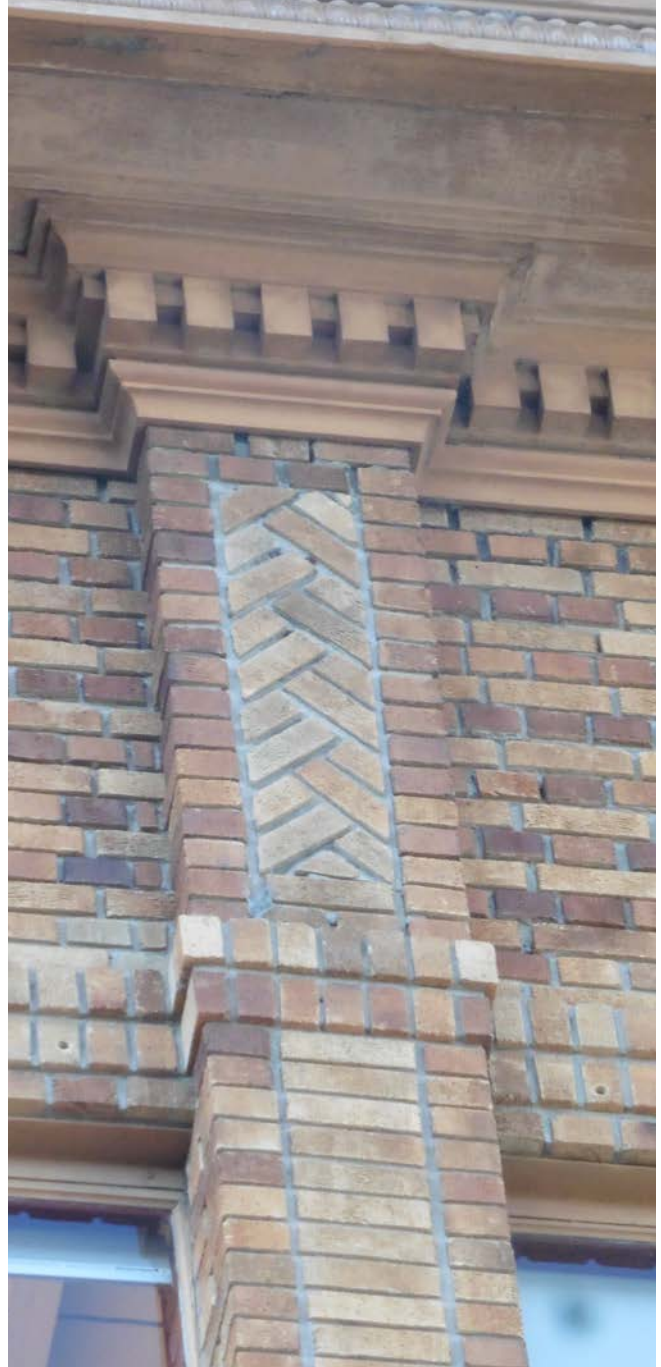
Figure 4. Detail of decorative brickwork at piers.
