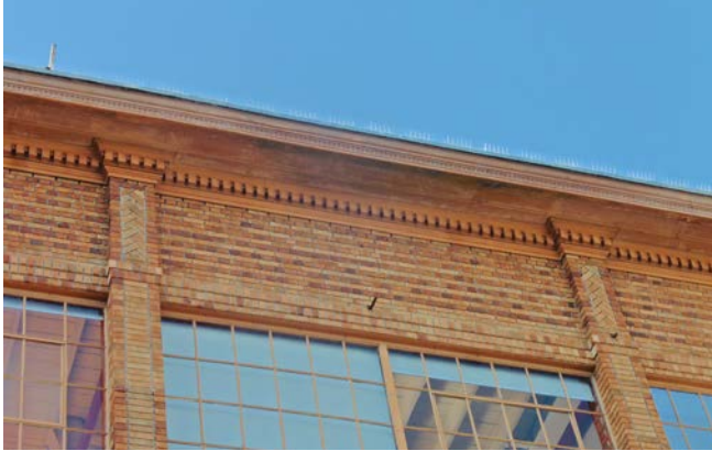
Figure 2. South Elevation; note dentils and decorative piers.
