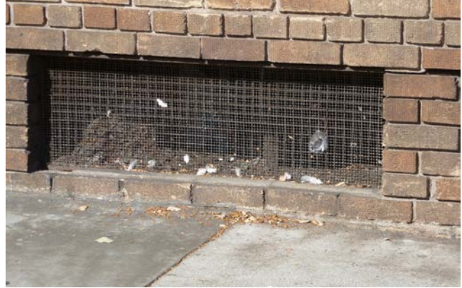
Figure 1. Ventilation grilles; note 1”x 1” historic iron grille.
