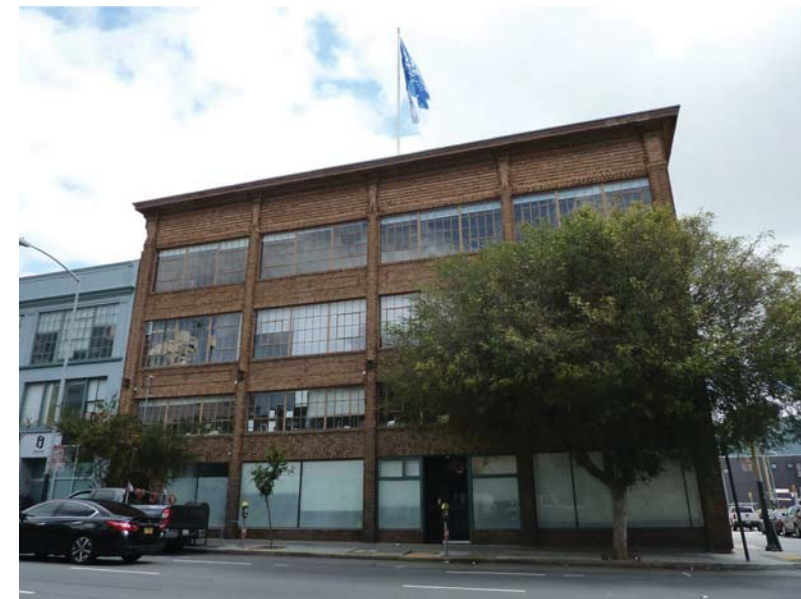
9TH STREET FACADE
