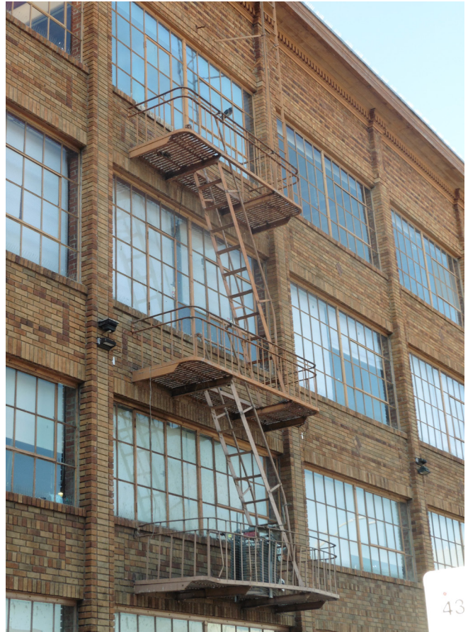
Figure 1. Metal fire escape at south elevation.
