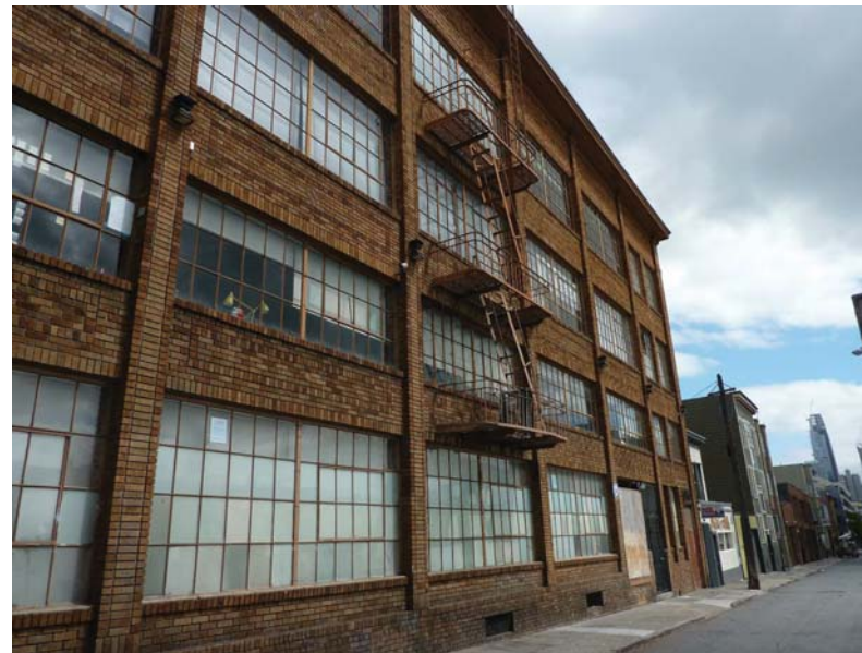
NATOMA STREET FACADE
