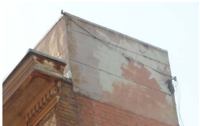
Figure 2. Penthouse from grade (east elevation).
