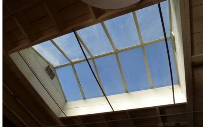
Figure 5. Skylight from interior.
