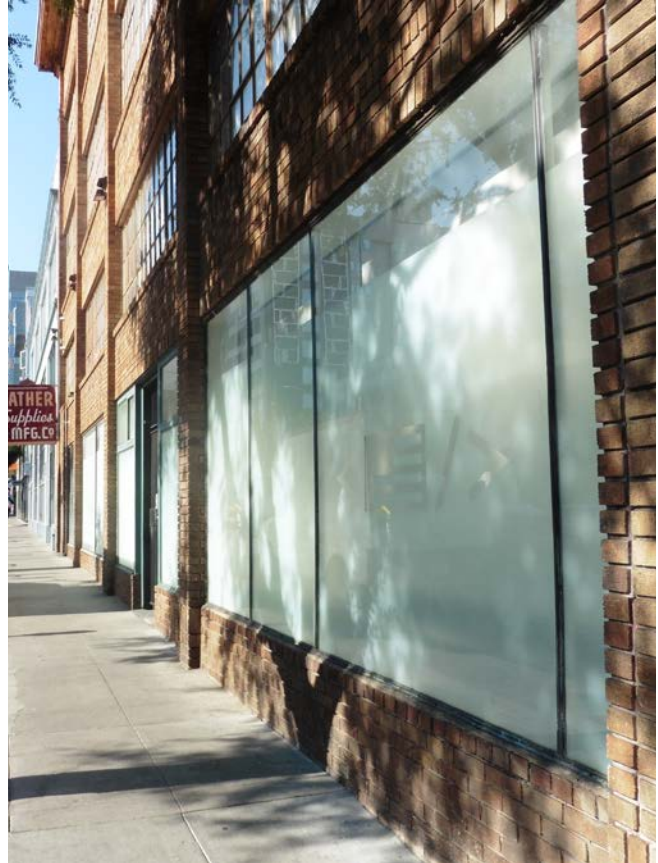
Figure 1. Typical Storefront at west elevation.
