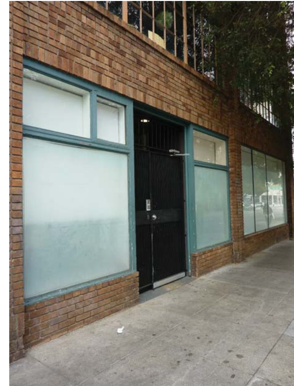
9TH STREET WINDOW DETAIL
