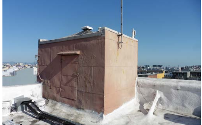
Figure 1. Penthouse from roof, typical.
