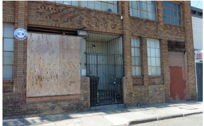
Figure 1. Service doors along south elevation.
