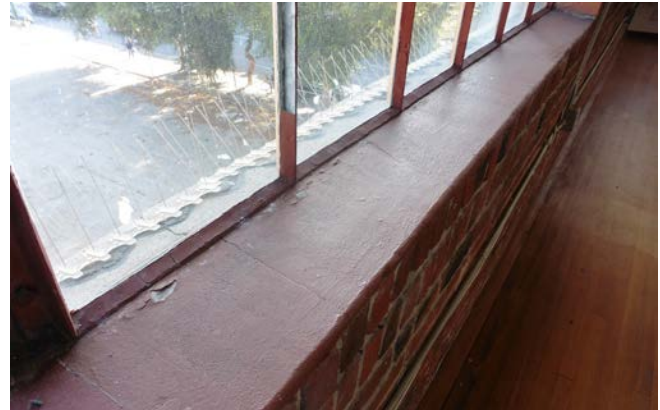
Figure 1: Window sills with concrete parge, typical.
