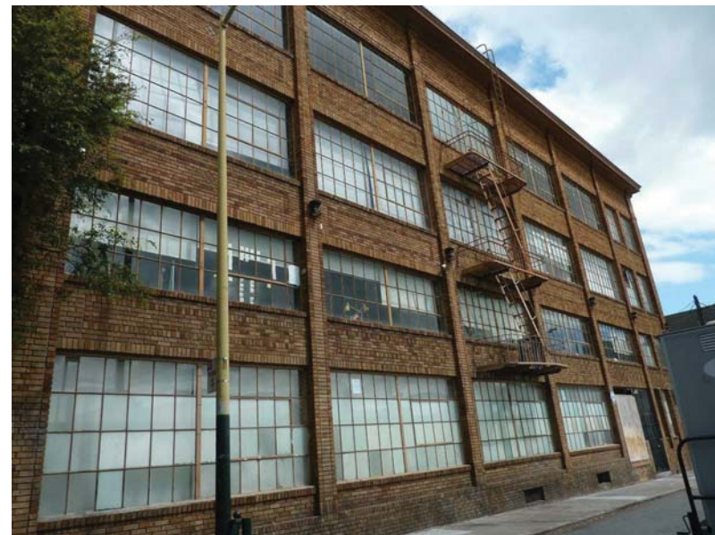
NATOMA STREET FACADE
