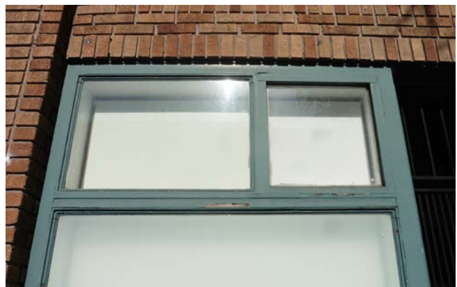
Figure 2. Non-historic split transom at storefront.
