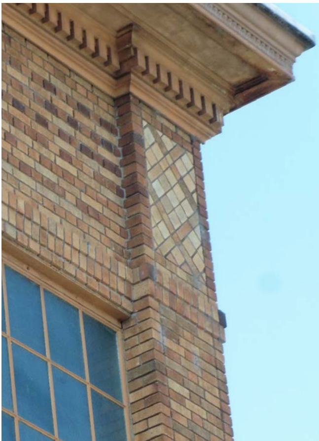
Figure 3. Southeast Corner; note decorative patterning and general brick pattern of elevation.
