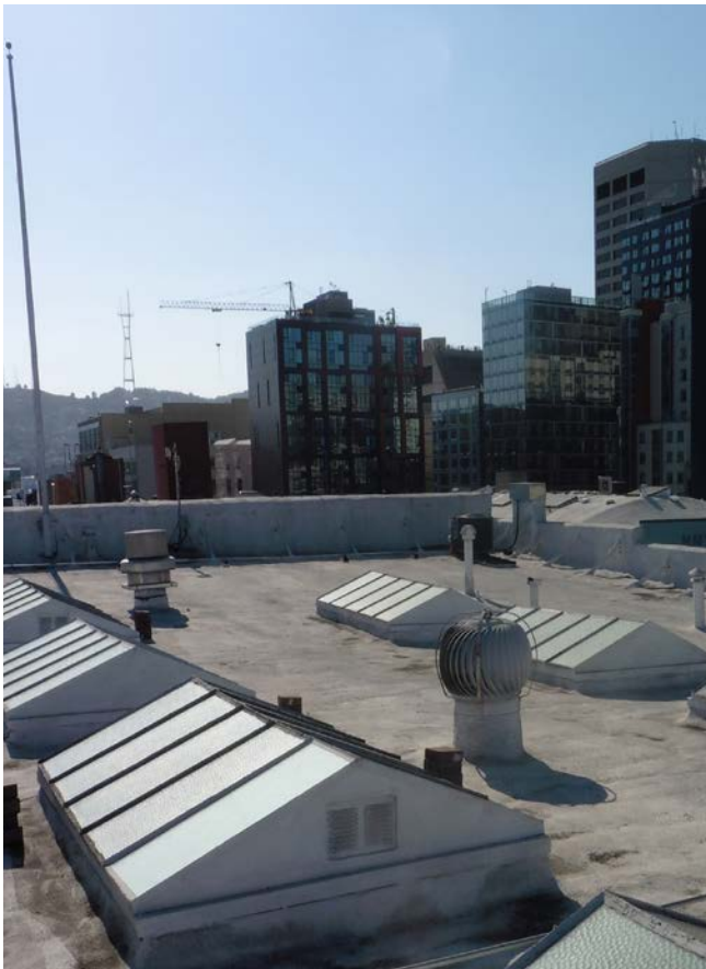
Figure 4. Skylights; note covered ventilation grilles.
