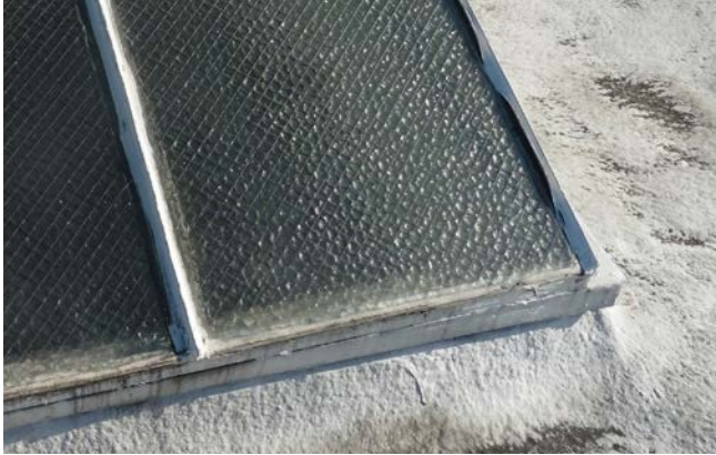
Figure 3. Skylight typical frame conditions.
