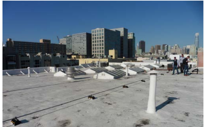
Figure 1. Roof of 149 9th Street, typical.
