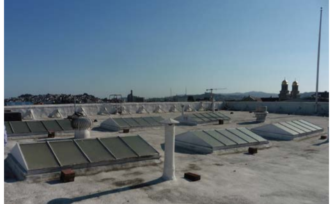
Figure 1. Roof overview; note skylights.
