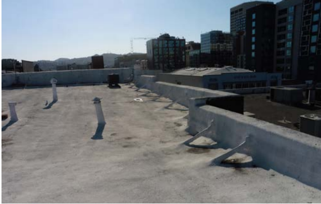
Figure 3. Roof along north elevation, typical.
