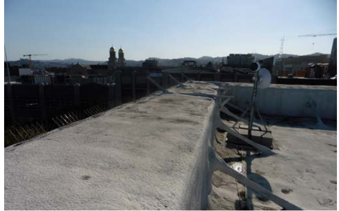
Figure 1. Parapet at southwest corner.
