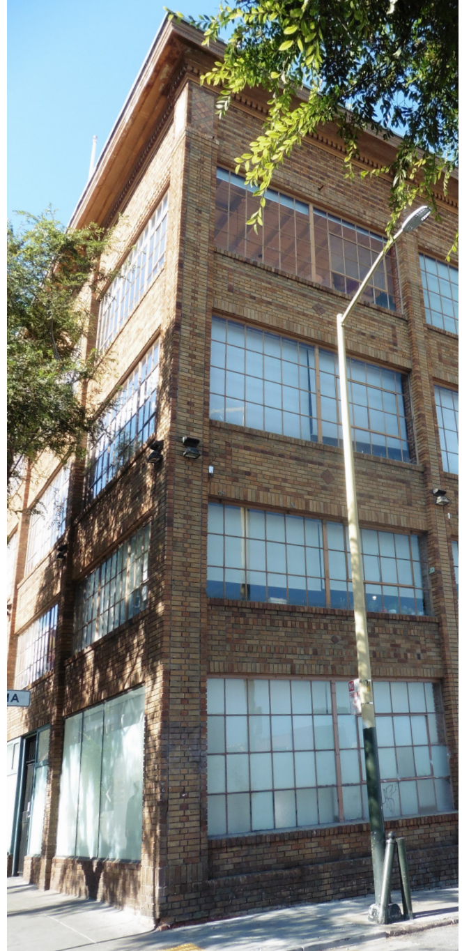
Figure 5. Typical window bay (south elevation)
