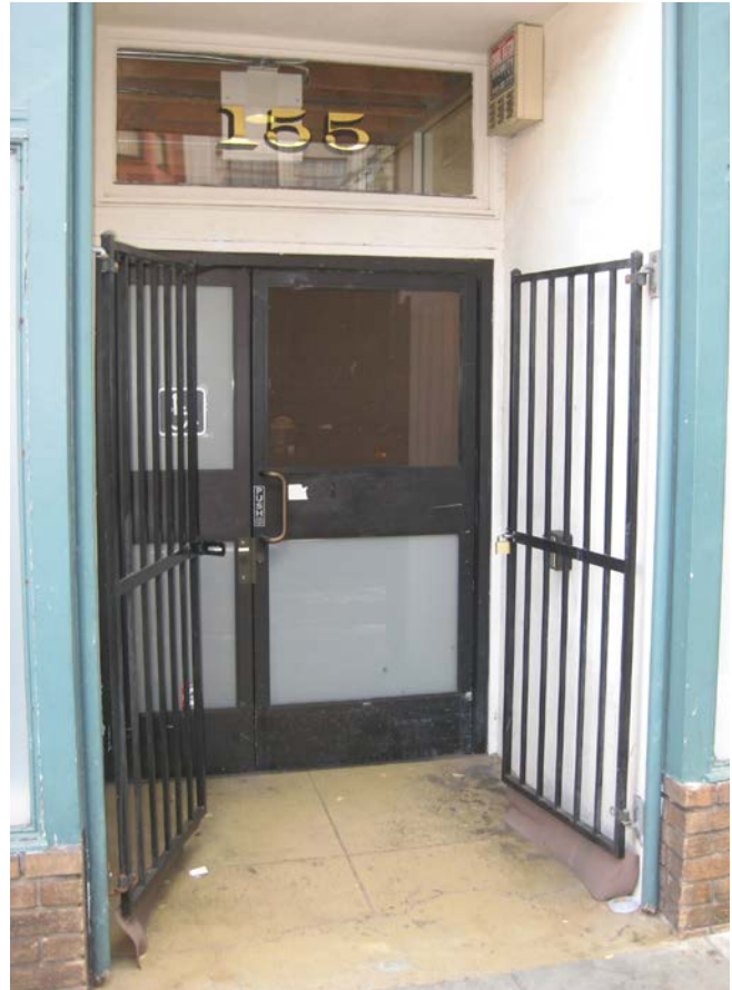
Figure 1. Metal entry door at west elevation.
