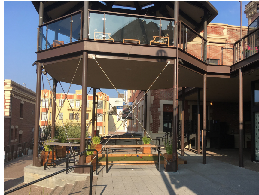
11. View of Carillon Building from Fountain Plaza (looking southeast)
