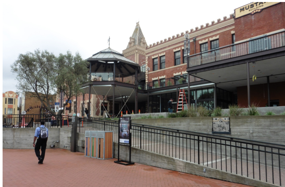
10. View of Carillon Building from Fountain Plaza (looking southeast)
