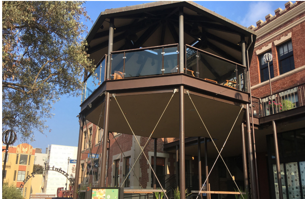
9. View of existing Carillon Building
