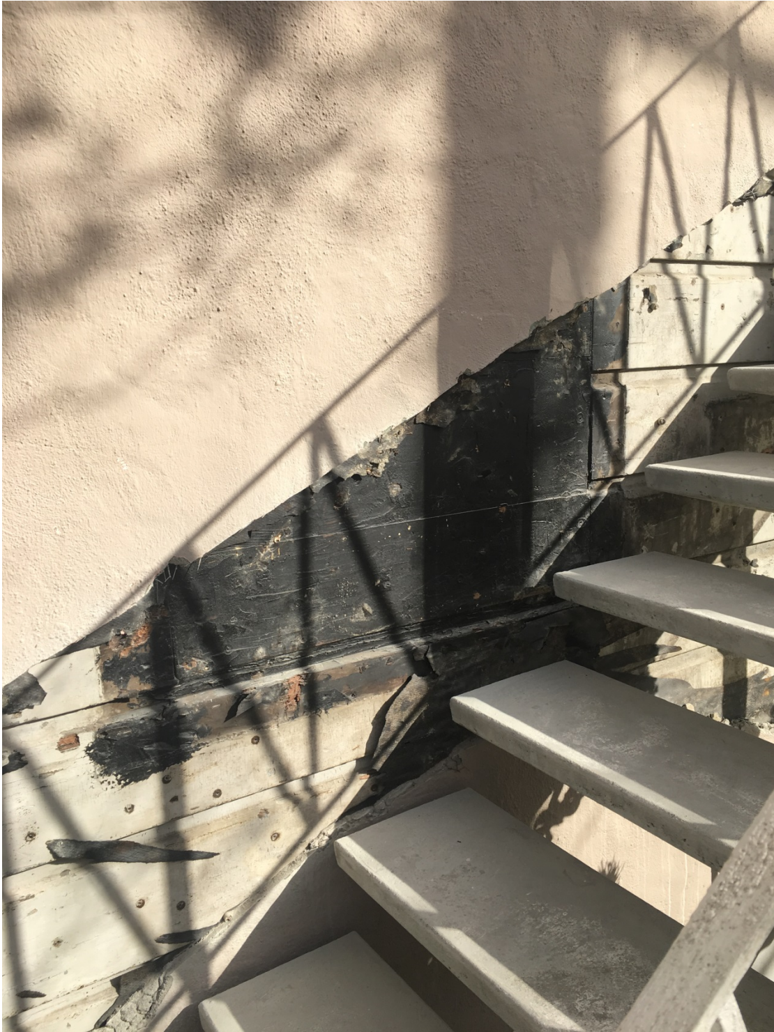
Results of physical investigation revealing historic siding and evidence of historic window and stair locations.
