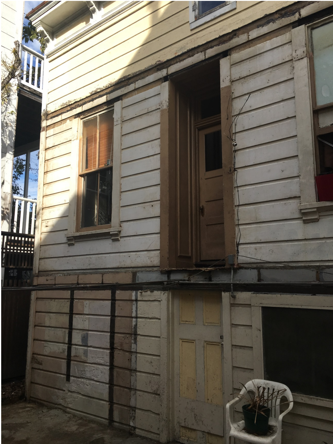
Façade of rear building after non-historic sun porch removal. Scarring at lower left corner indicates historic stair location.
