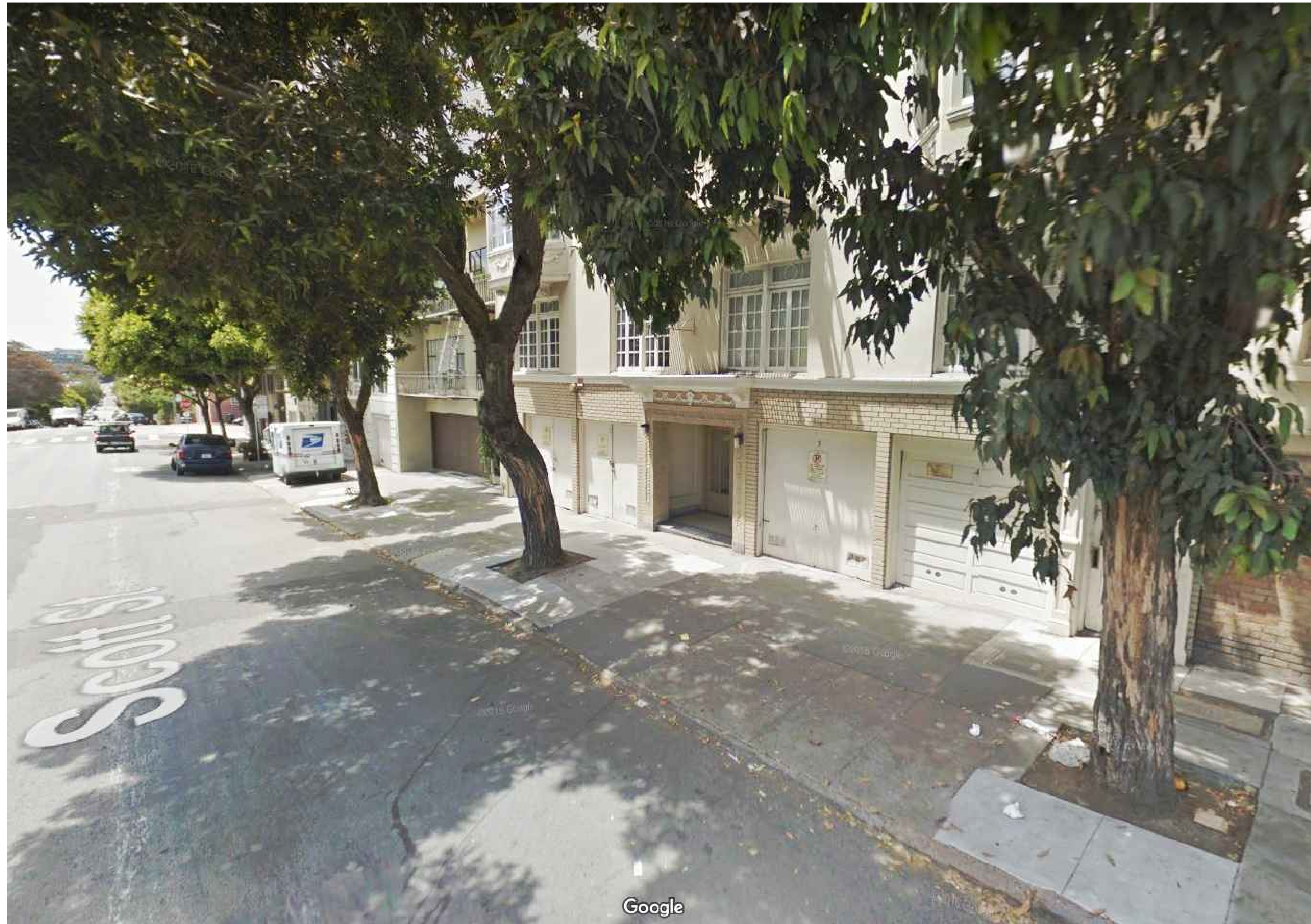
1 EXISTING FRONT FACADE - RIGHT NOT TO SCALE
