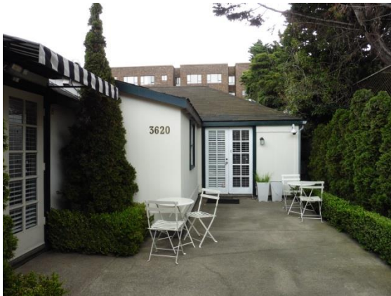
Figure 6: West façade of eastern-most bay, facing east.
