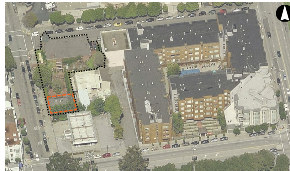
Aerial view of the subject block. Subject property is outlined with black dashes. Current garden house/workshop building at 3620 Buchanan Street is outlined with orange dashes (Microsoft Bing Maps, 2016, edited by Page & Turnbull).
