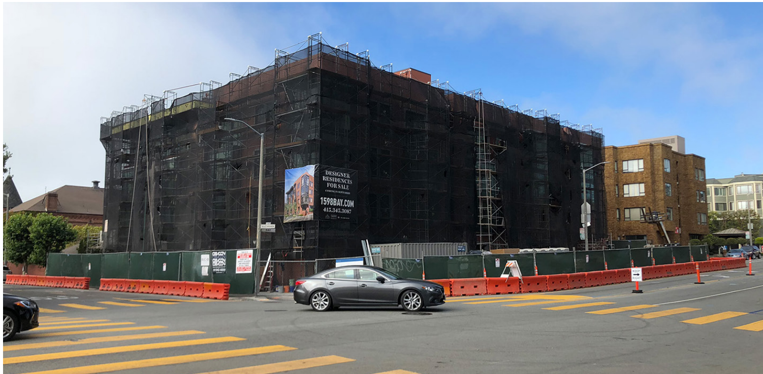
BUCHANAN ST. + BAY ST. - ADJACENT PROPERTY
