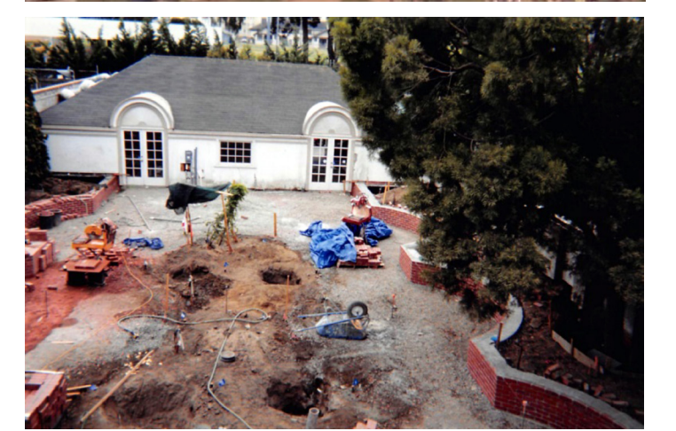
2000 Photo of garden ca. 2000 under construction.
