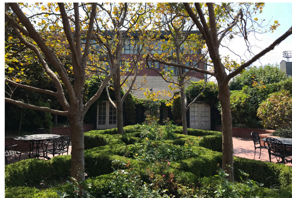
Rear (north) façade of garden house/workshop and courtyard garden, facing south.
