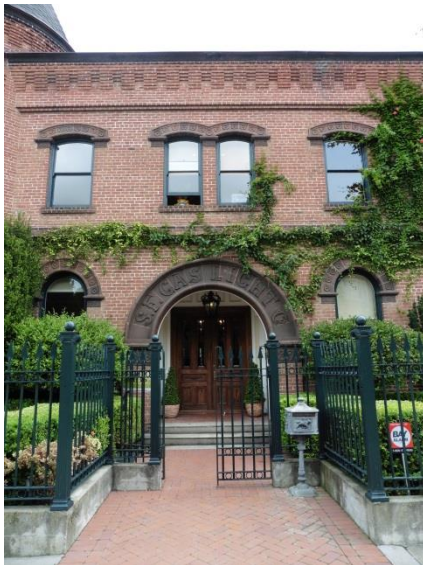
Figure 14: Iron gate and main entrance to Landmark No. 58, facing east.
