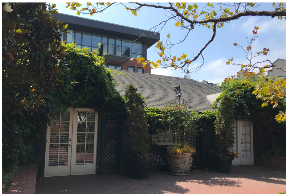
Rear (north) façade of garden house/workshop, facing southwest.
