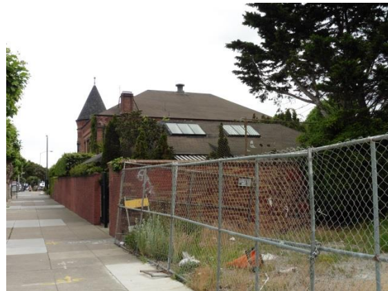
Figure 23: South brick wall of concrete patio with roofs of Landmark No. 58 and subject building in background, facing north.
