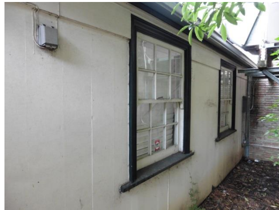
Figure 7: South façade of eastern-most bay, facing northeast.
