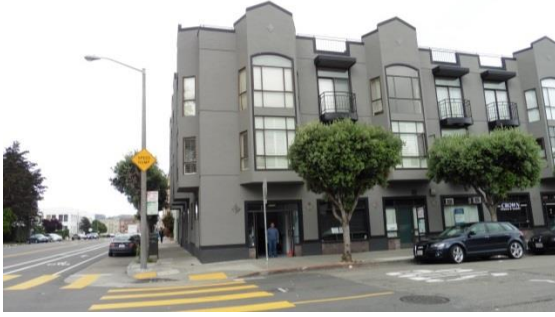
Figure 30: Apartment building with commercial ground floor, west of subject block, facing west.
