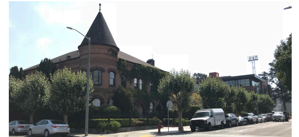
View of subject block face from the northwest corner of Buchanan and North Point streets, facing southeast (Page & Turnbull, September 2018).
