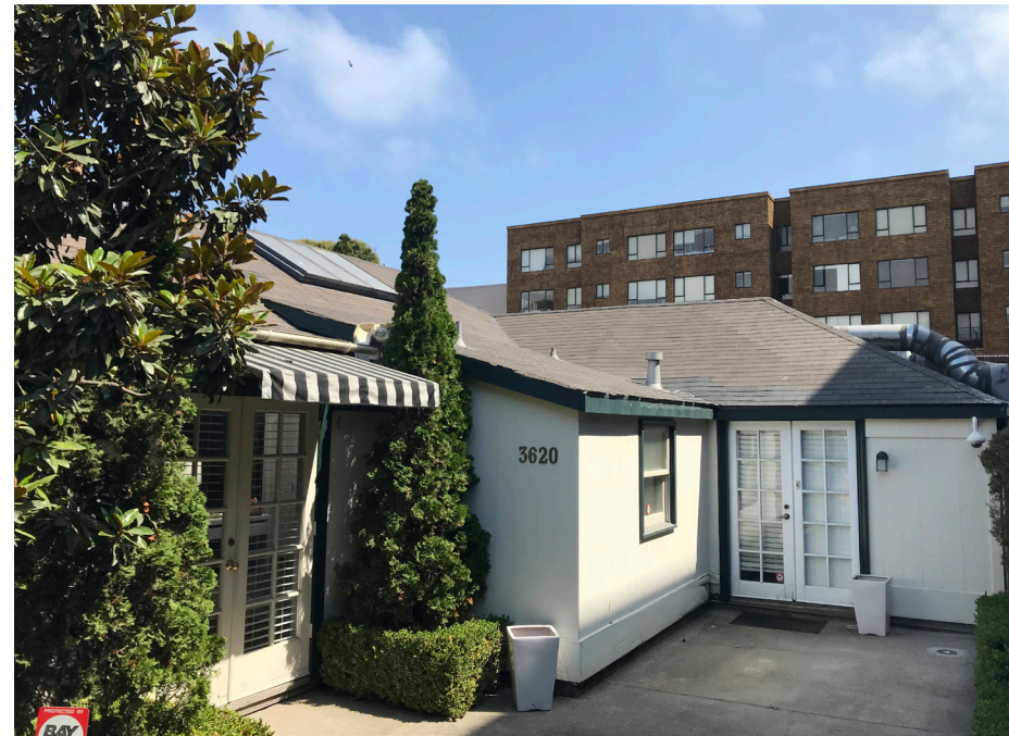
West façade of eastern-most bay of garden house/workshop, facing east.
