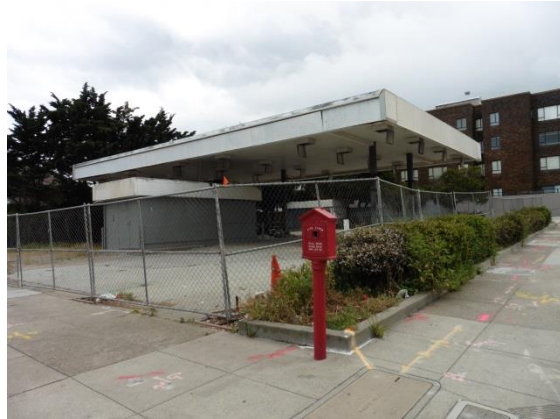
Figure 25: Abandoned gas station, facing northeast.
