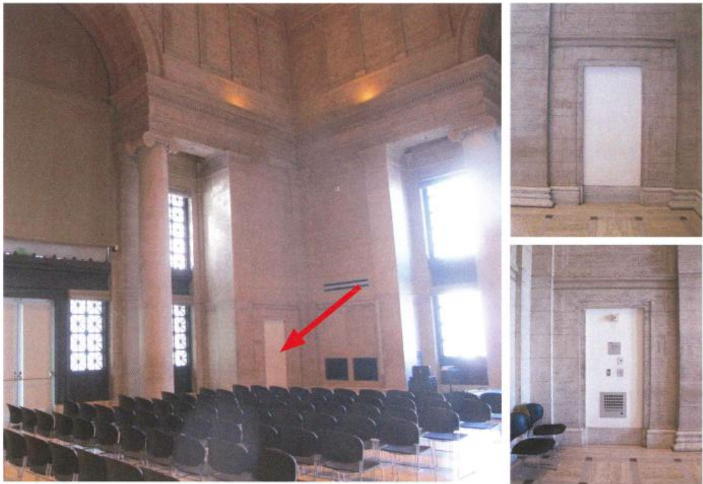
9. (clockwise) Location of proposed 100 amp connection box; 10. Closeup of wall panel; 11. Existing power location in similar panel at northwest corner of the room.
