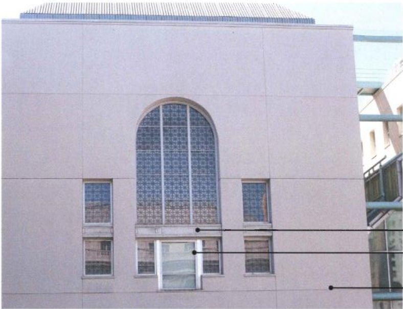
Building facade at Samsung Hall: within the historic window assembly, a non-historic windowframe is proposed to be replaced with a double door
