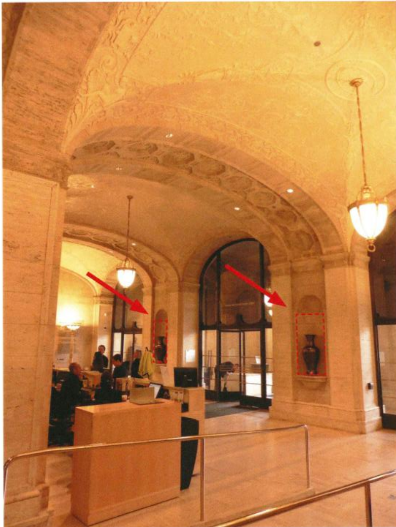
3. View of lobby and main entrance. Arrows and red outlines indicate location of proposed digital display screens to be mounted at existing decorative plaster niches. There will be small penetrations into the plaster to mount new connection clips for the screens, and new conduit whips for power/data.
