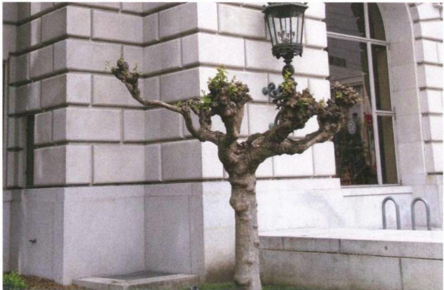
Close-up view of the San Francisco War Memorial Opera House: its historic facades were constructed of terra cotta units with a similar color and texture to Raymond granite.
