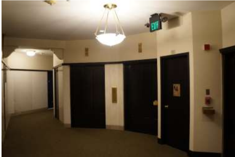
Typical upper floor elevator lobby, Hearst Building. (Knapp Architects photograph.)
