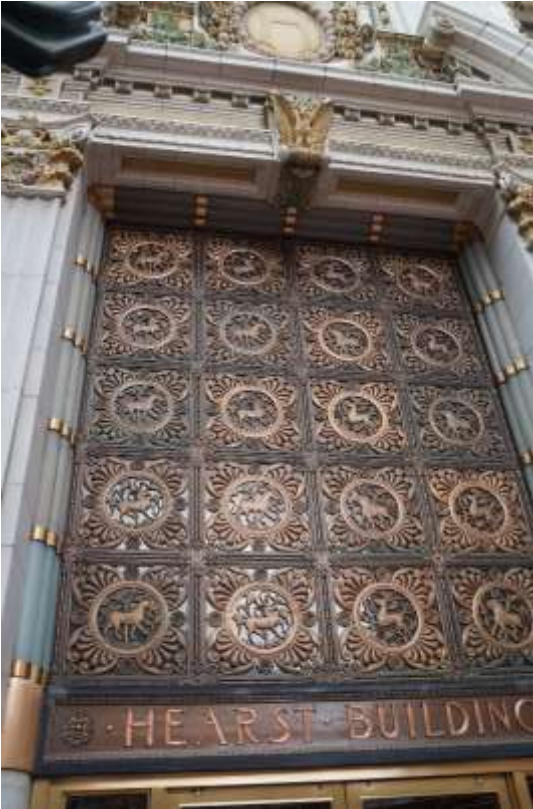
Entry portal detail showing bronze screen. (Knapp Architects photograph.)
