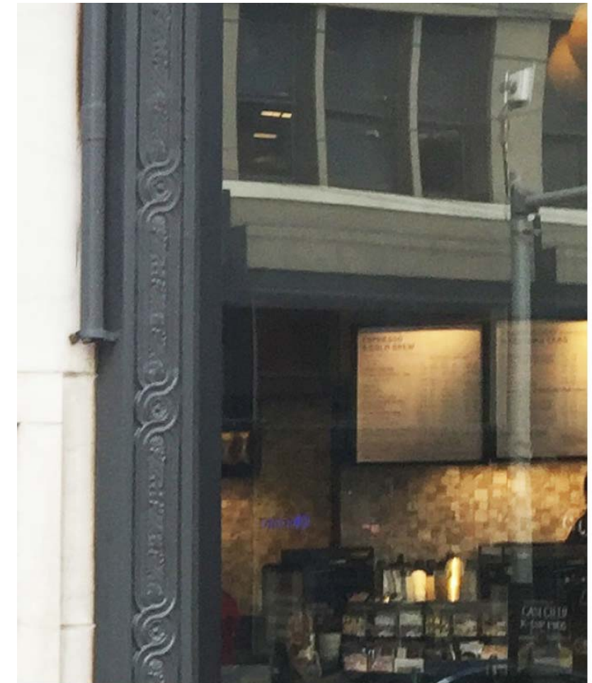
EXISTING ORNAMENTAL SURROUND
