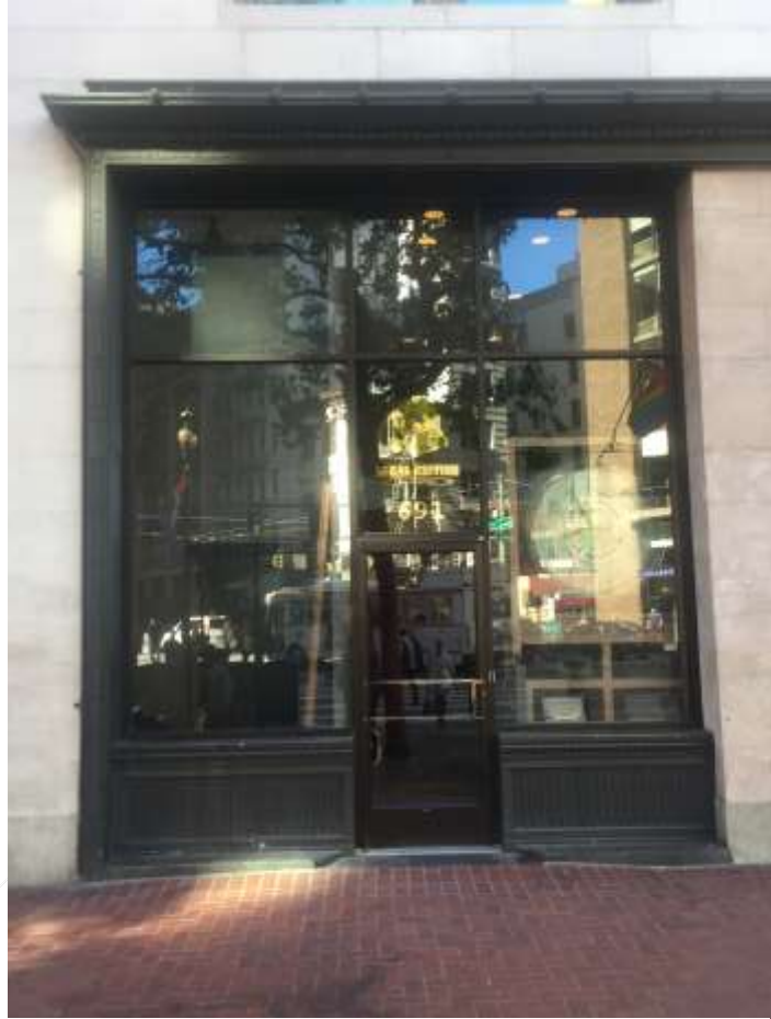
Market Street storefront, easternmost bay (at Local Edition bar). Note original cast iron bulkhead and storefront surround. (Knapp Architects photograph.)
