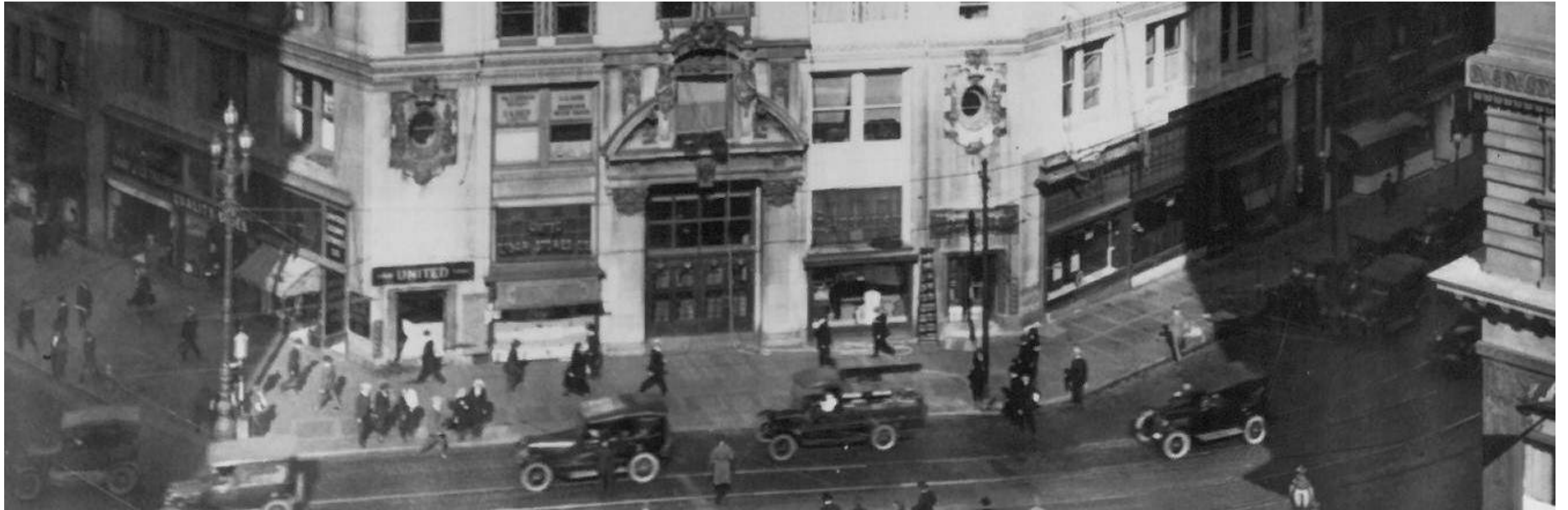
1911 - End of Construction
