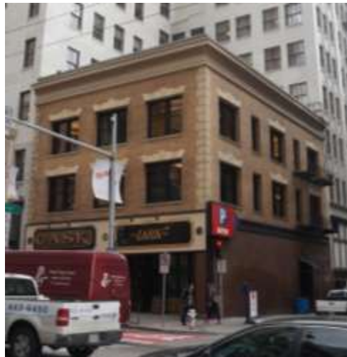
View of 17-29 Third Street, looking northeast. (Knapp Architects photograph.)
