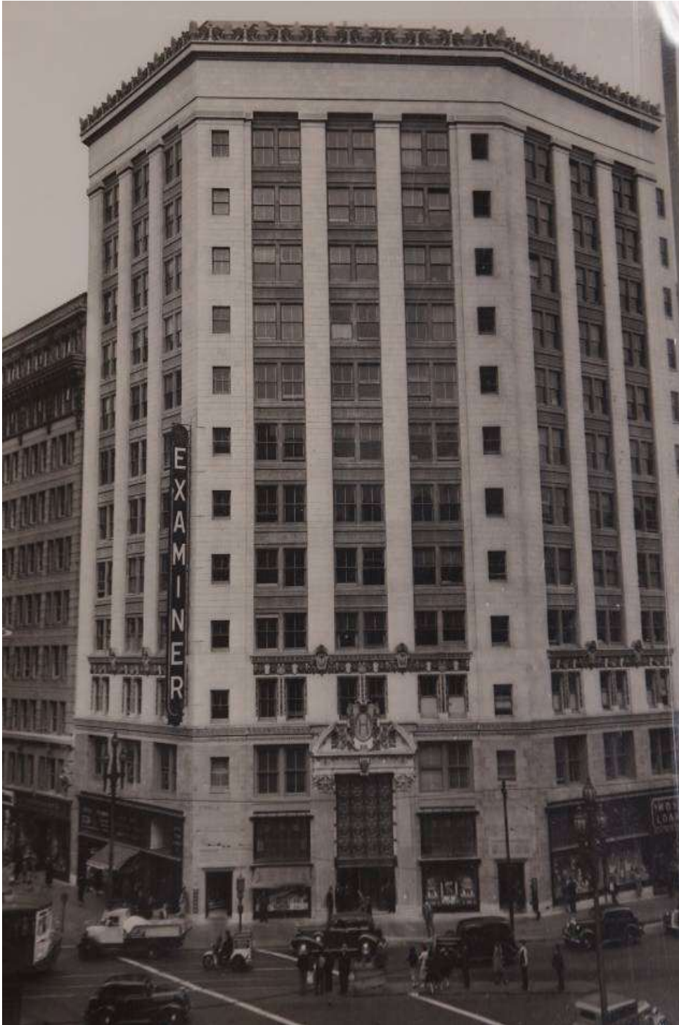
San Francisco Examiner Building, c 1938. (Julia Morgan archives, California Polytechnic University, San Luis Obispo.)
