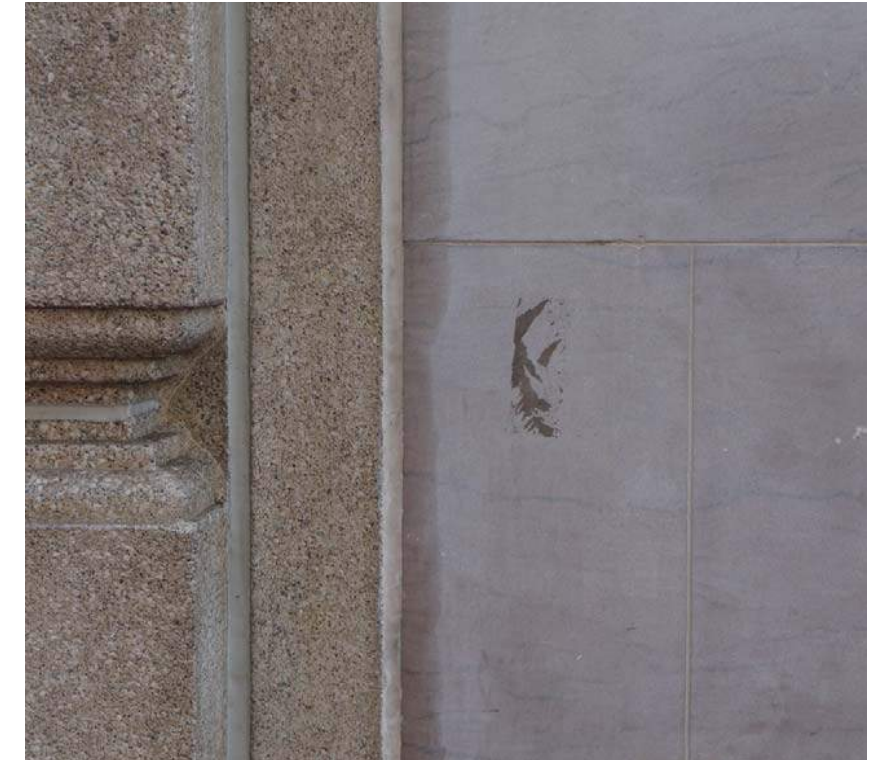
Hearst Building – Minor residue at marble podium
