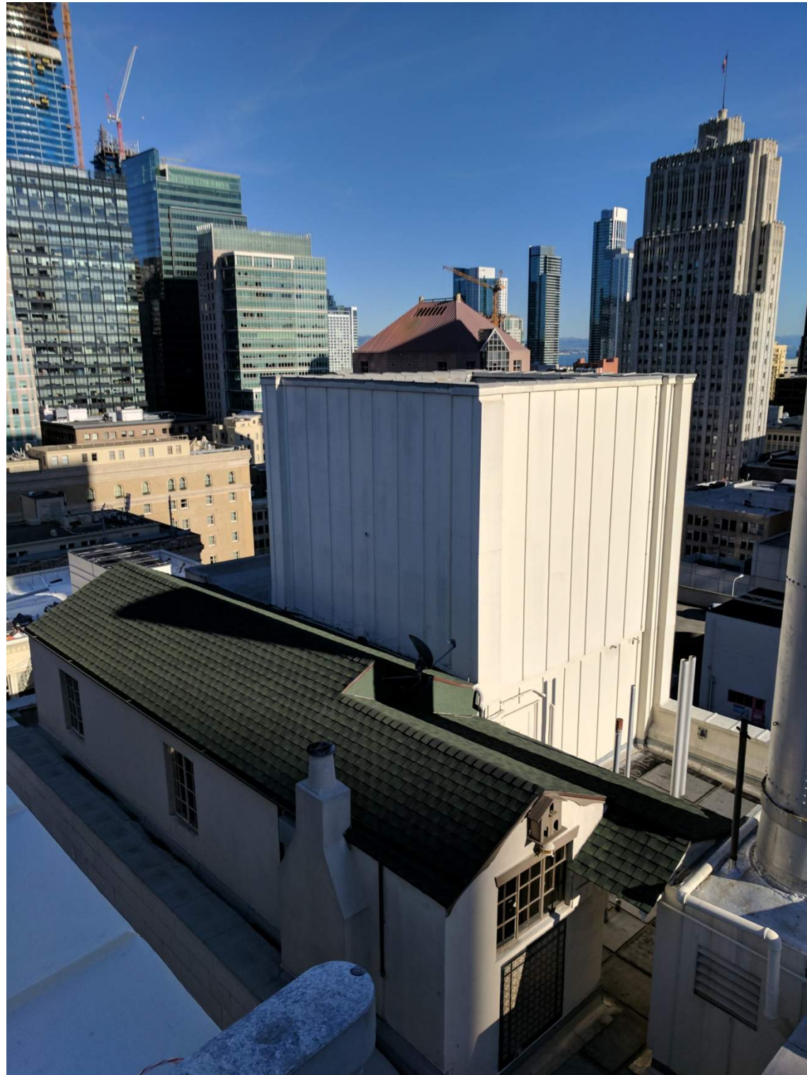
The penthouse as viewed from the upper roof looking southeast.
