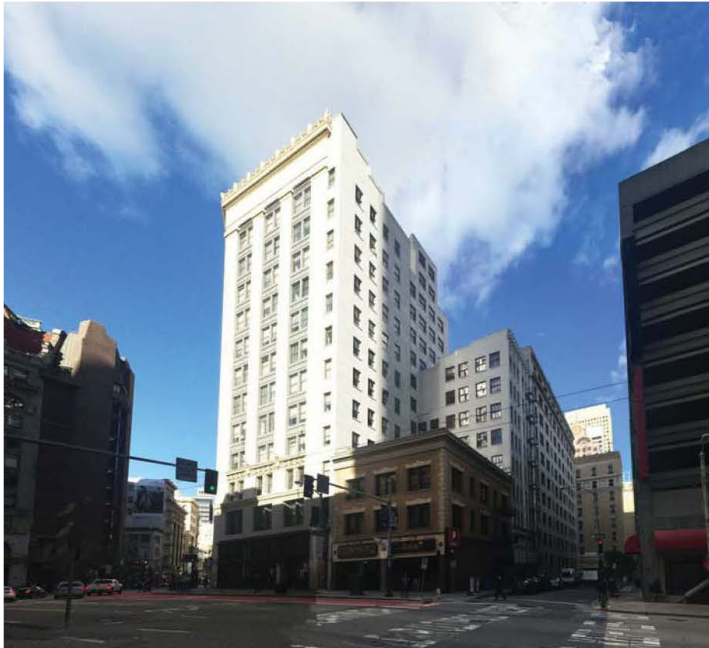
EXISTING view looking east from Third Street at Stevenson Street
