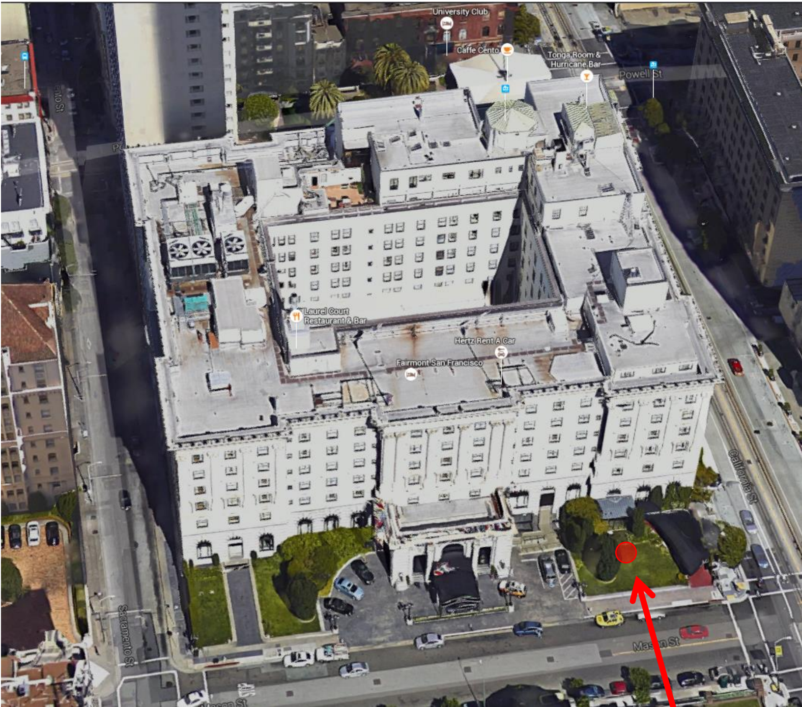
950 Mason Street (looking east)
