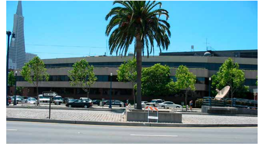
KGO - from The Embarcadero across project park site
