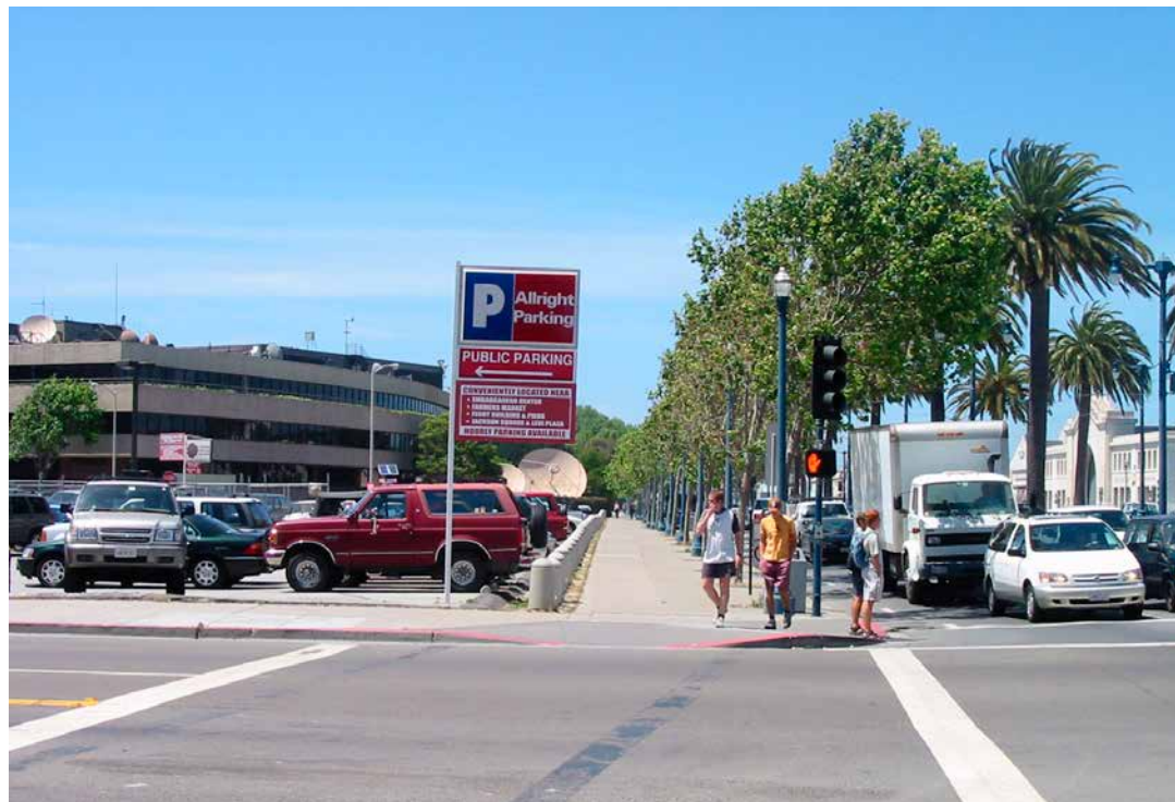
Existing Site Broadway/Embarcadero Corner Looking North
