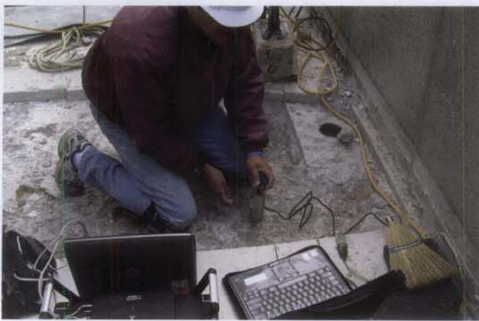
Figure 16. Impact echo testing is performed on a concrete structural slab to help determine depth of deterioration. In this method, a short pulse of energy is introduced into the structure and a transducer mounted on the impacted surface of the structure receives the reflected input waves or echoes. These waves are analyzed to help identify flaws and deterioration within the concrete.
