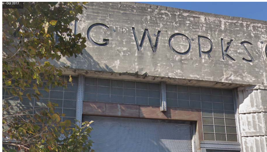
FIGURE 3. EXISTING 'SAN FRANCISCO GALVANIZING WORKS' FACADE LETTERING
