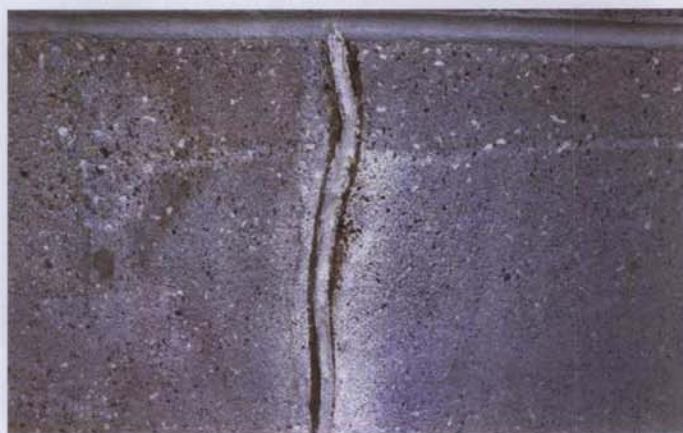
Figure 19. A high-speed grinder is used to widen a crack in preparation for installation of a sealant. This process is called "routing." After the crack is prepared, the sealant is installed to prevent moisture infiltration through the crack. Although sealant repairs can provide a durable, watertight repair for moving cracks, they tend to be very visible.
