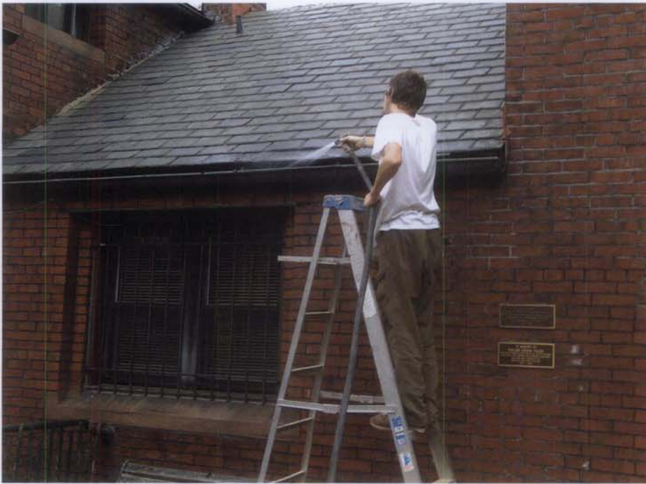
Figure 3. Keeping gutters clean of debris can be one of the most important cyclical maintenance activities. On this small one-story addition, a garden hose is being used to flush out the trough to ensure that the gutter and downspouts are unobstructed. Gutters on most small and medium size buildings can be reached with an extension ladder and a garden hose. Photo: Bryan Blundell.
