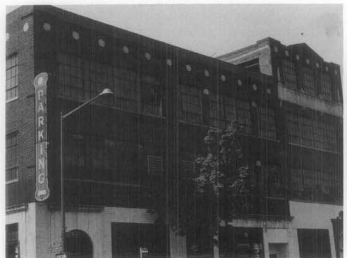
Fig. 5 Windows often provide a strong visual element to relatively simple or unadorned industrial or commercial buildings. This design element should be taken into consideration when evaluating the significance of the windows. Photo: Michael Auer.
