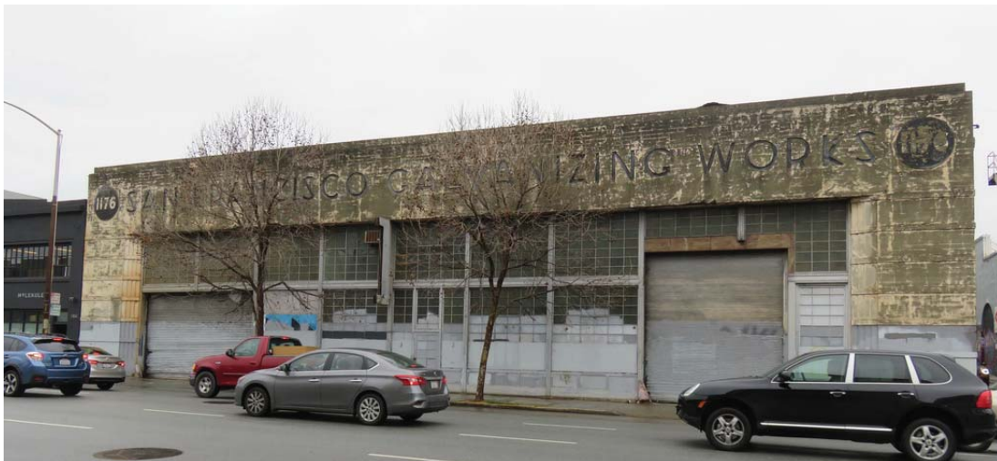
Overview of primary, Harrison Street façade of 1170 Harrison Street (ARG, 2018).
