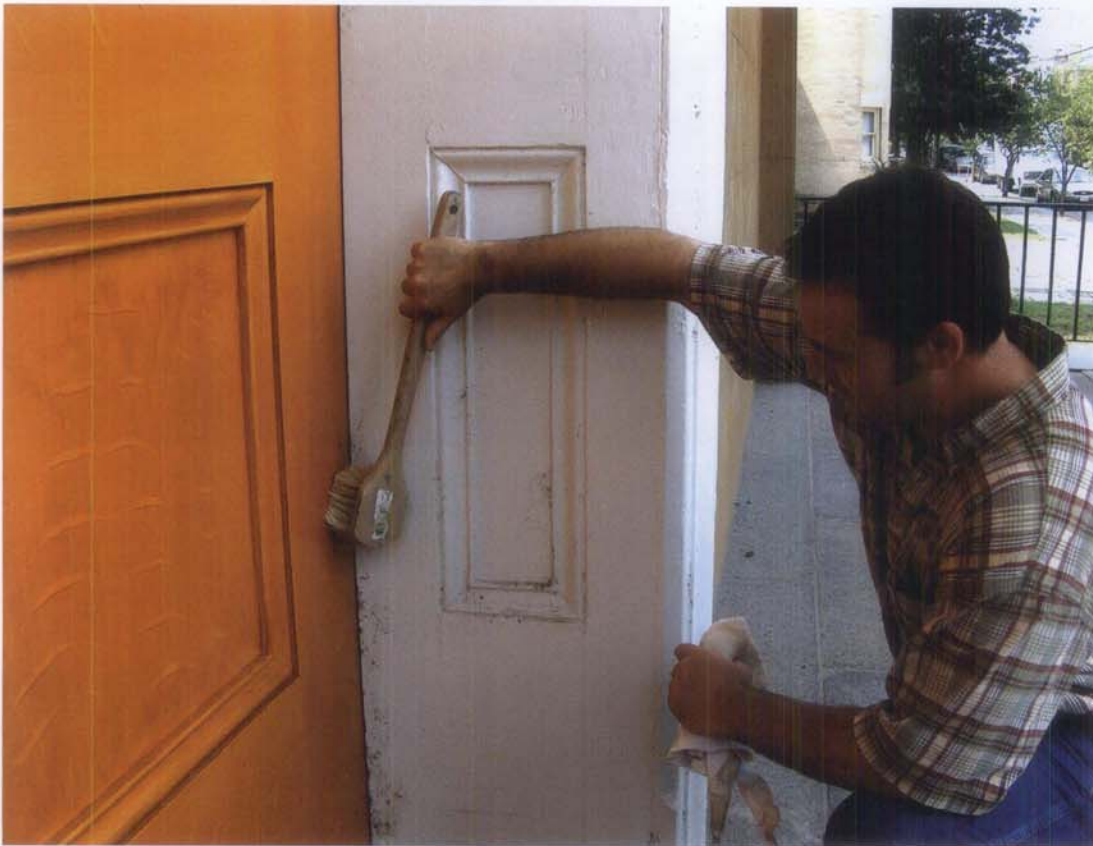
Figure 9. To help extend a repainting cycle, dirt and spider webs should be removed before permanent staining occurs. In this case, a natural bristle brush and a soft damp cloth are being used to remove insect debris and refresh the surface appearance.
