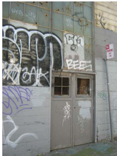
Detail view of entrance on secondary façade. Source: Page and Turnbull
