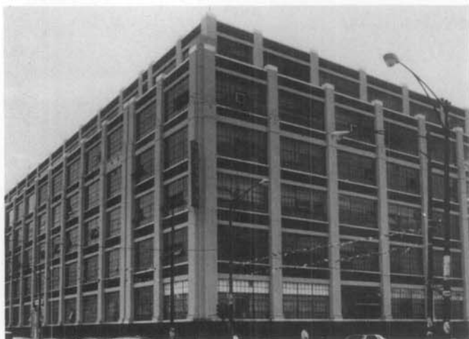
Fig. 10 a. A six-story concrete manufacturing building prior to the replacement of the steel pivot windows. Photo: Charles Parrott.
