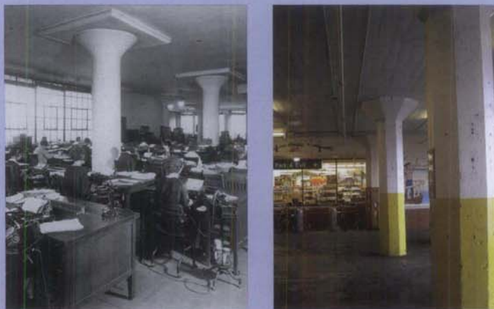
Figure 11. Whether in a circa 1925 office (left) or in a parking garage and retail facility (right), exposed concrete structures help characterize these building interiors. Photo: Minnesota Historical Society (left).
