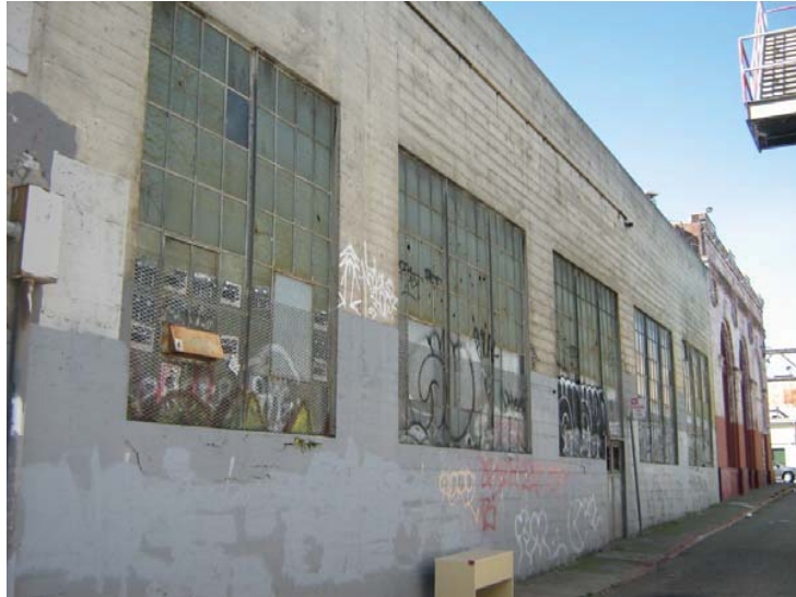
View of secondary façade on Berwick Place. Source: Page and Turnbull
