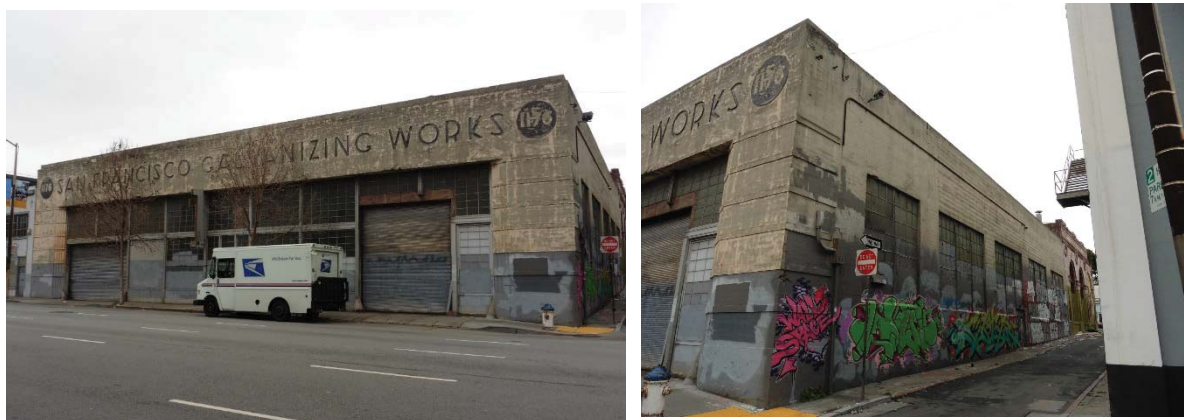
Figure 1: (Left) Harrison Street façade; (Right) Berwick Place façade.
