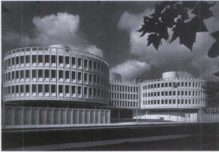
Figure 5. Following World War II, architects and engineers took advantage of improvements in concrete production, quality control, and advances in precast concrete to design structures such as the Police Headquarters building in Philadelphia, Pennsylvania, constructed in 1961. Photo: Courtesy of the Philadelphia Police Department.
