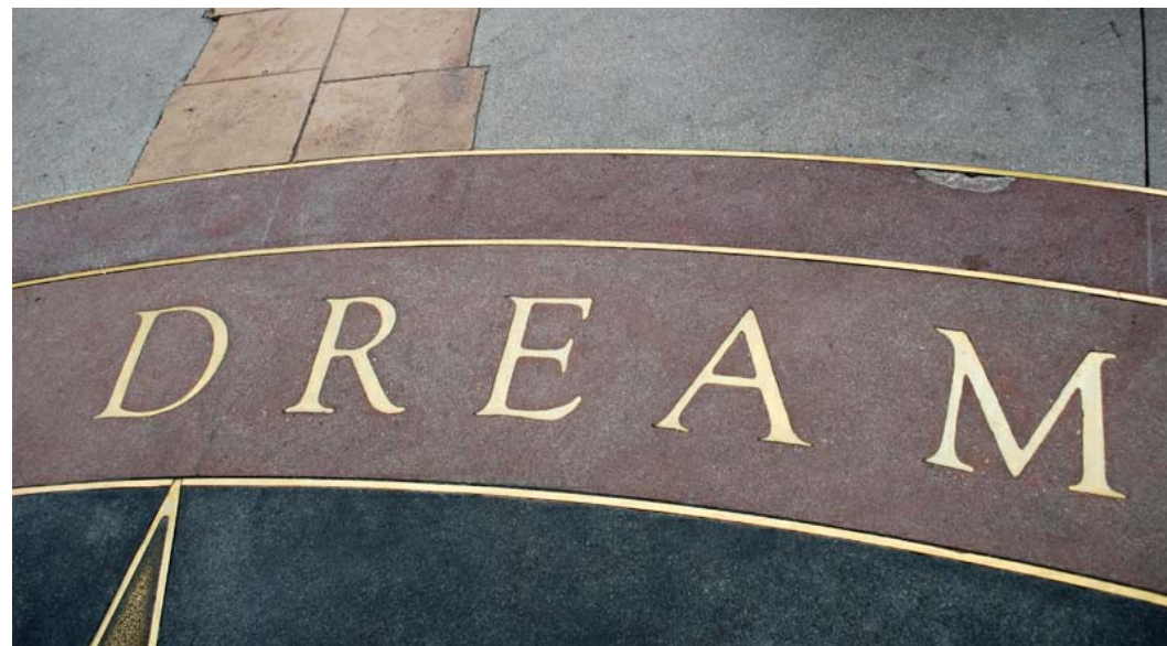
FIGURE 1. REFERENCE BRASS INLAY IN CONCRETE
