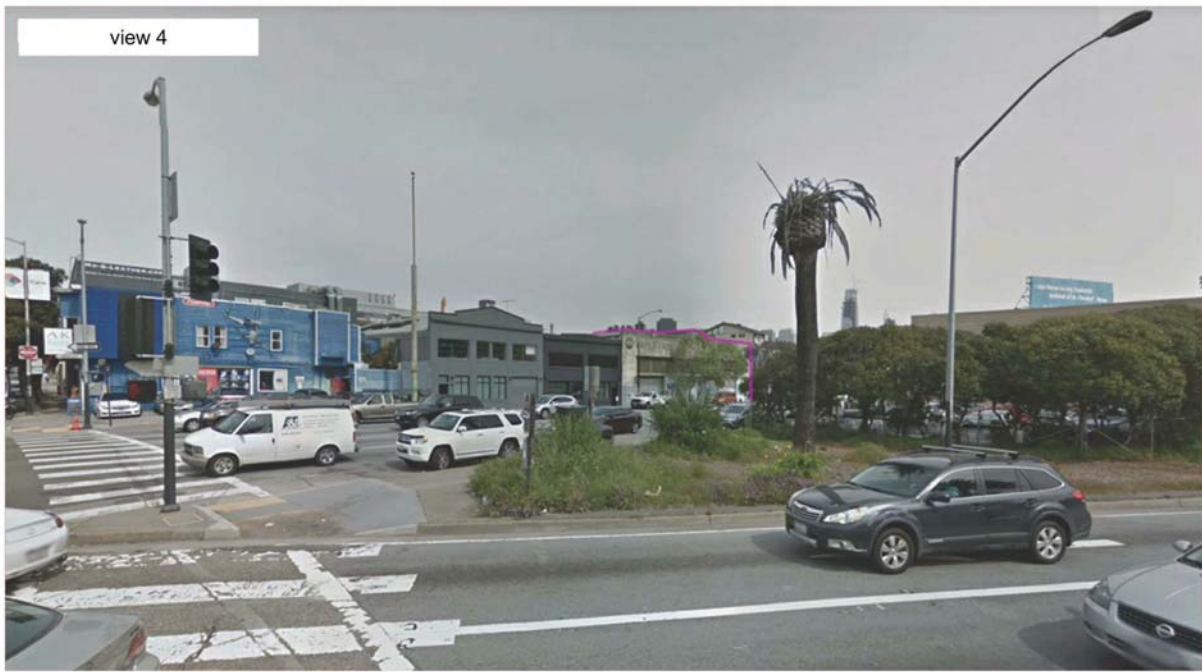
workshop 1 view 4 - Existing 1170 Harrison Street
