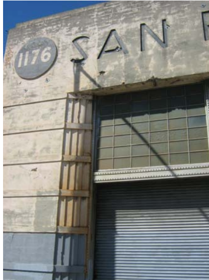
Detail view of ornament on primary façade. Source: Page and Turnbull
