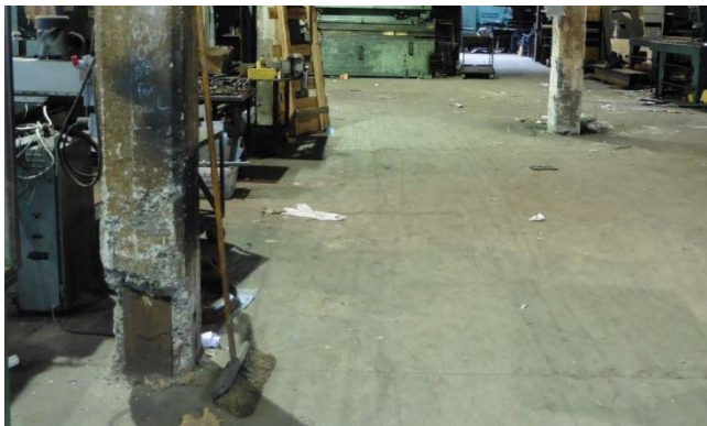
Figure 21: Section of poured concrete flooring within west warehouse space.
