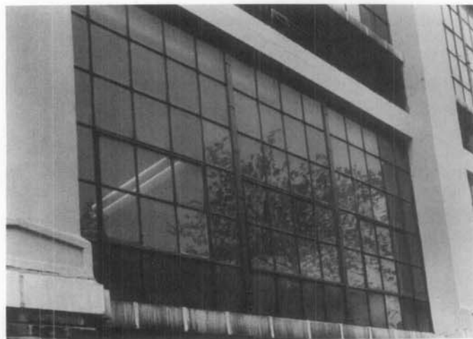
Fig. 10 b. Close-up view of the new replacement steel windows which matched the multi-lighted originals exactly. Photo: Charles Parrott.
