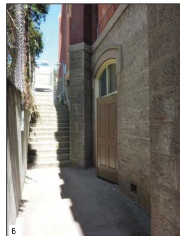
6 LOOKING NORTH AT ELEVATOR SITE
