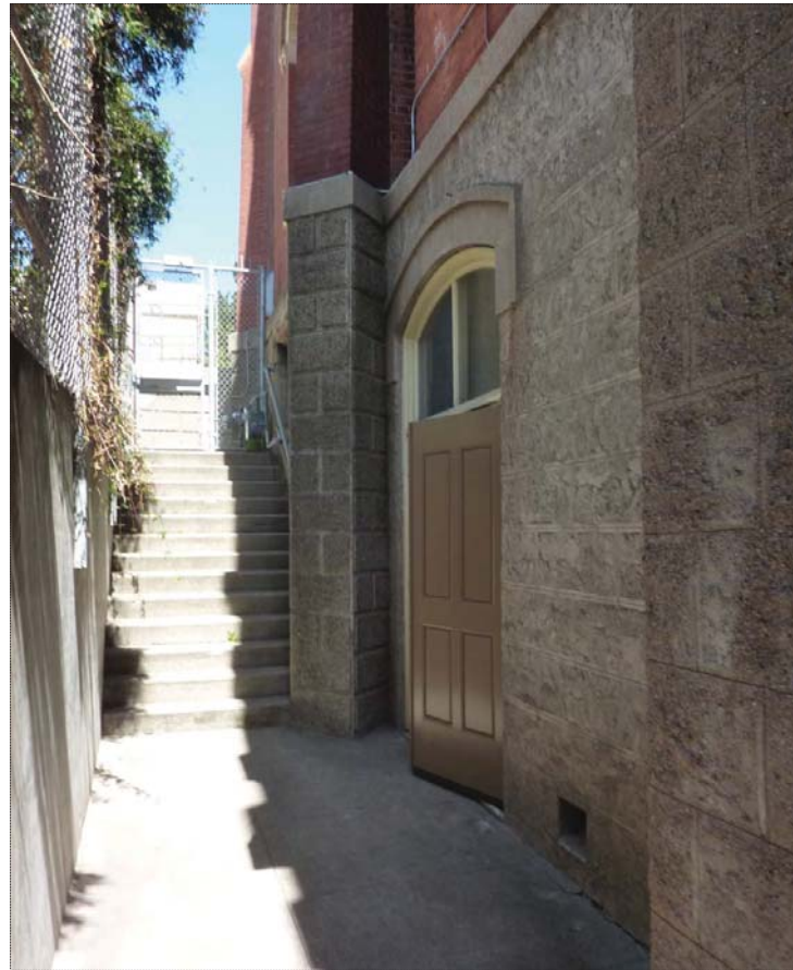
LOOKING NORTH AT EXTERIOR LOCATION OF PROPOSED ELEVATOR
