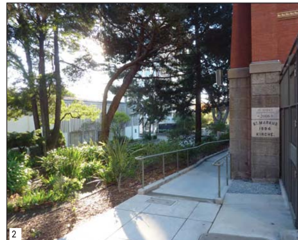
2 LOOKING SOUTH FROM NORTH EAST CORNER OF CHURCH
