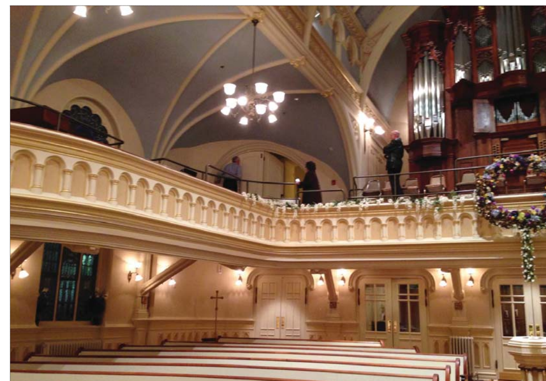
LOOKING NORTH-WEST FROM SANCTUARY TOWARDS DOORS LEADING TO ELEVATOR ACCESS VESTIBULES AT MAIN AND BALCONY LEVEL.
