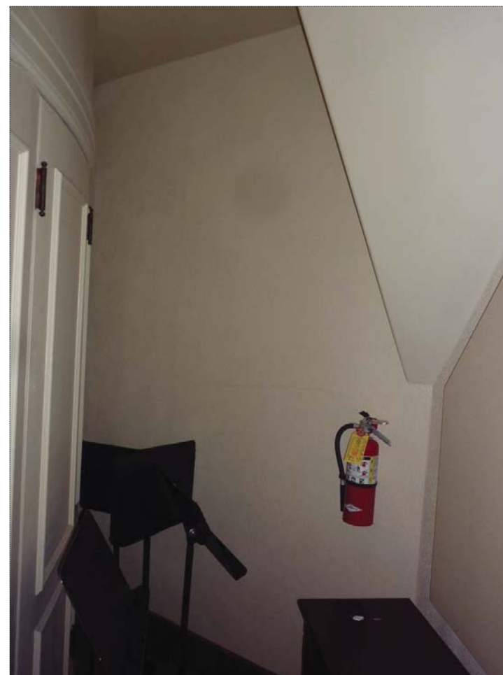
LOOKING WEST TOWARDS PROPOSED ENTRANCE TO ELEVATOR LOBBY
