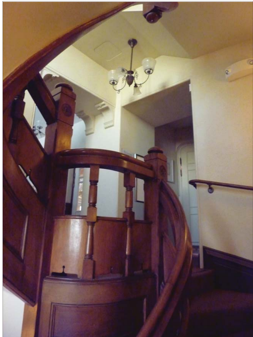
LOOKING SOUTH-EAST TOWARDS ENTRANCE TO PROPOSED ELEVATOR ACCESS VESTIBULE
