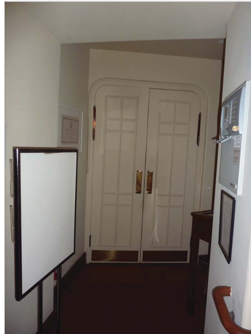
LOOKING SOUTH THROUGH PROPOSED ELEVATOR ACCESS VESTIBULE TOWARD SANCTUARY
