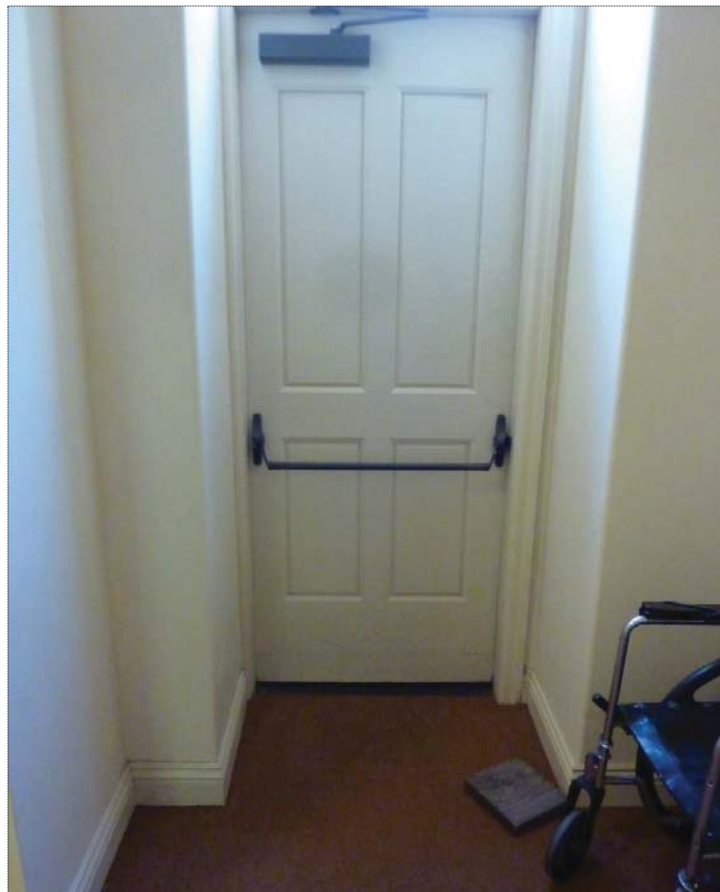
LOOKING WEST AT LOCATION OF OPENING TO ELEVATOR LOBBY
