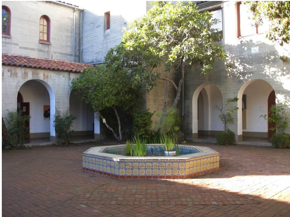
8. View northeast of the courtyard. Source: Page & Turnbull
