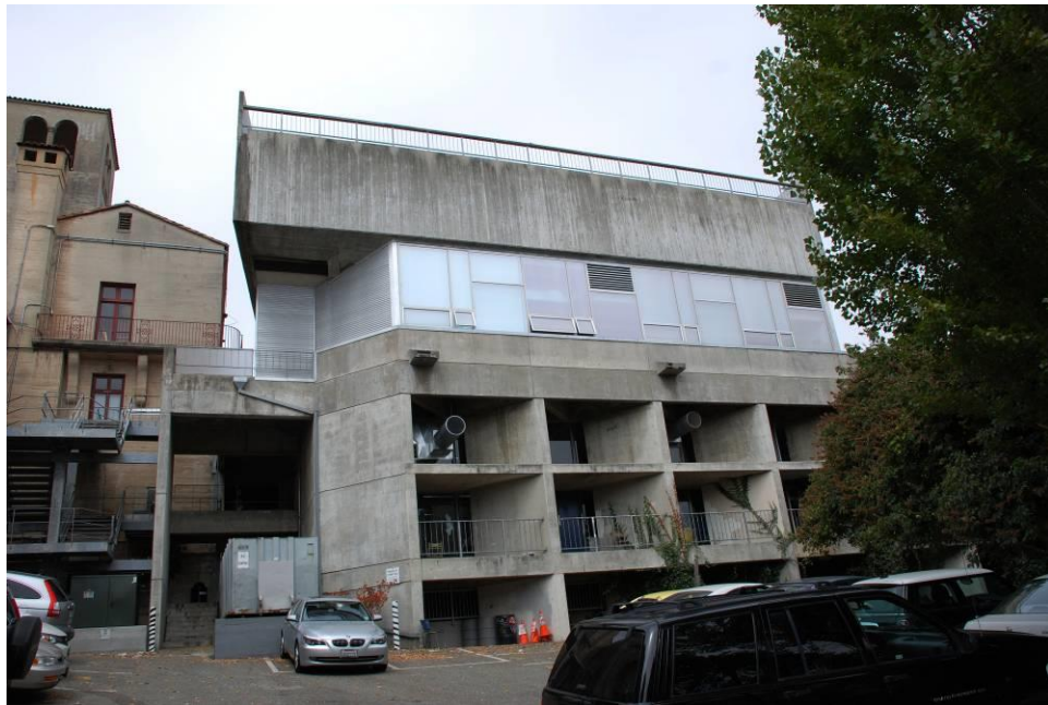
14. Detail of the east facade of the Addition. Source: Page & Turnbull
