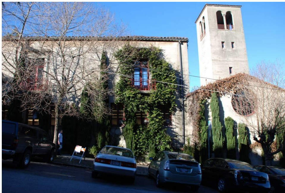
2. Detail of the west end of the south facade. Source: Page & Turnbull
