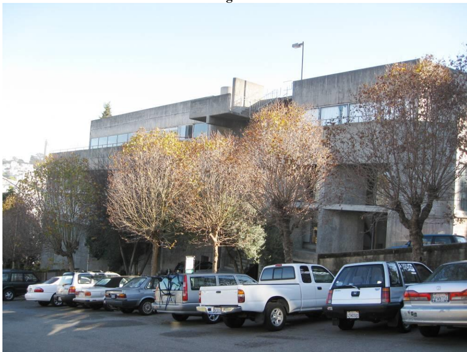
16. North facade of the Addition facing Francisco Street. Source: Page & Turnbull
