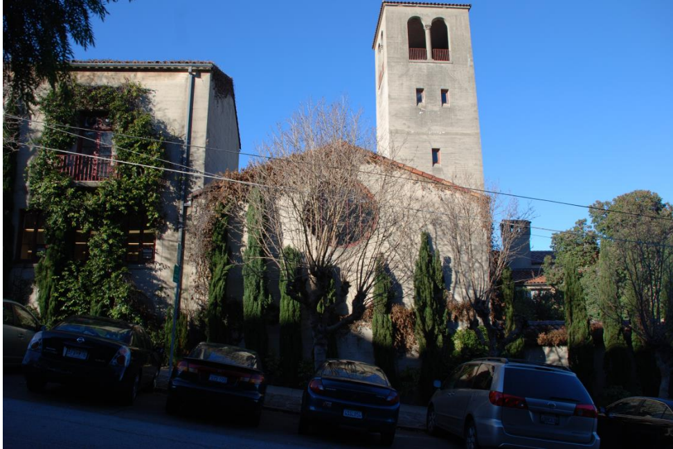
3. Detail of the south (primary) façade, at center. Source: Page & Turnbull
