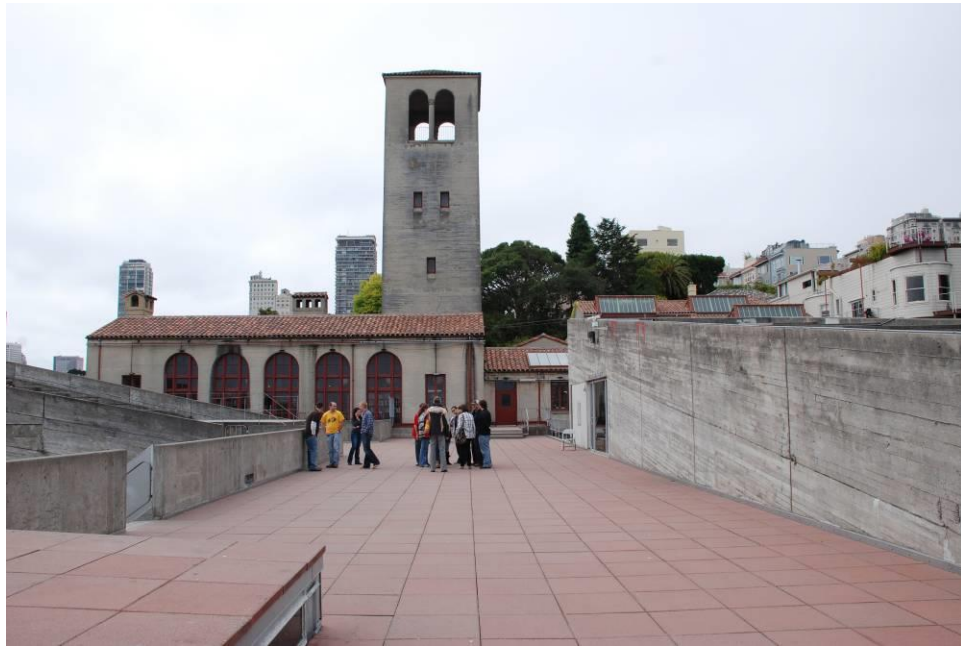
18. View south across the roof of the Addition toward the Original Building. Source: Page & Turnbull
