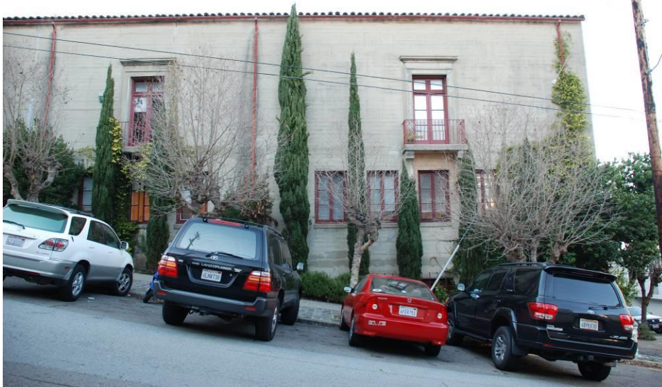
5. Detail of the east end of the south facade. Source: Page & Turnbull
