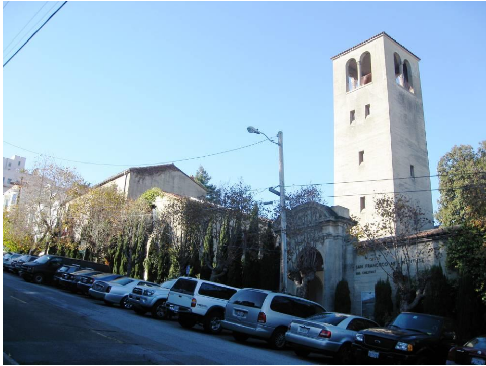
1. South (primary) facade of the original building facing Chestnut Street. View is northwest. Source: Page & Turnbull
