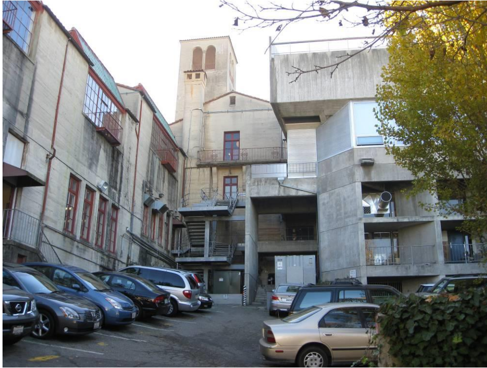
13. View west of the transition between the Original Building and the Addition. Source: Page & Turnbull
