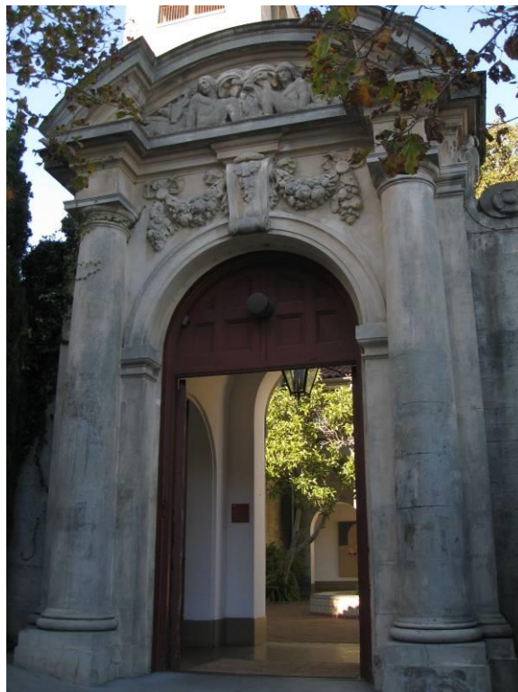
6. Detail of arched entry facing Chestnut Street, Source: Page & Turnbull
