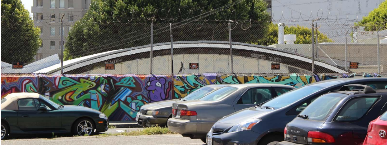
Figure 40. Former Hopkins Auto Repair Shop, rear façade, looking south.
