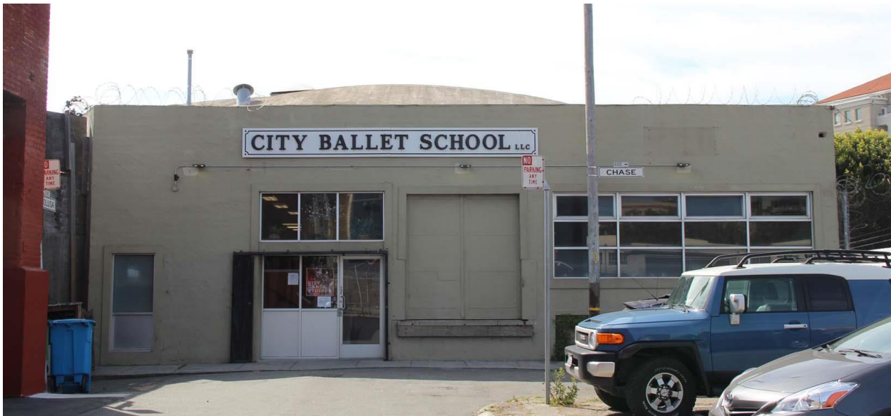
Figure 34. Salta Co. Building, rear façade, facing southeast.
