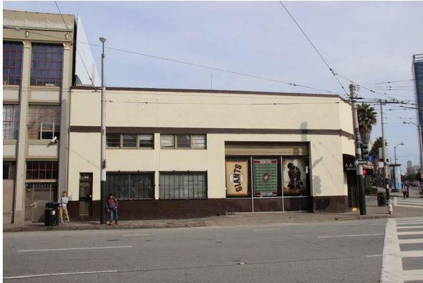
Figure 24. John McKee Building, southeast façade.
