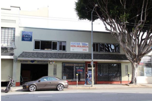
Figure 8. 42 Otis Street, looking northwest.
