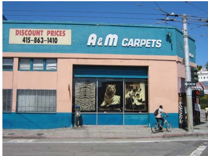
North half of south (Otis Street) elevation
