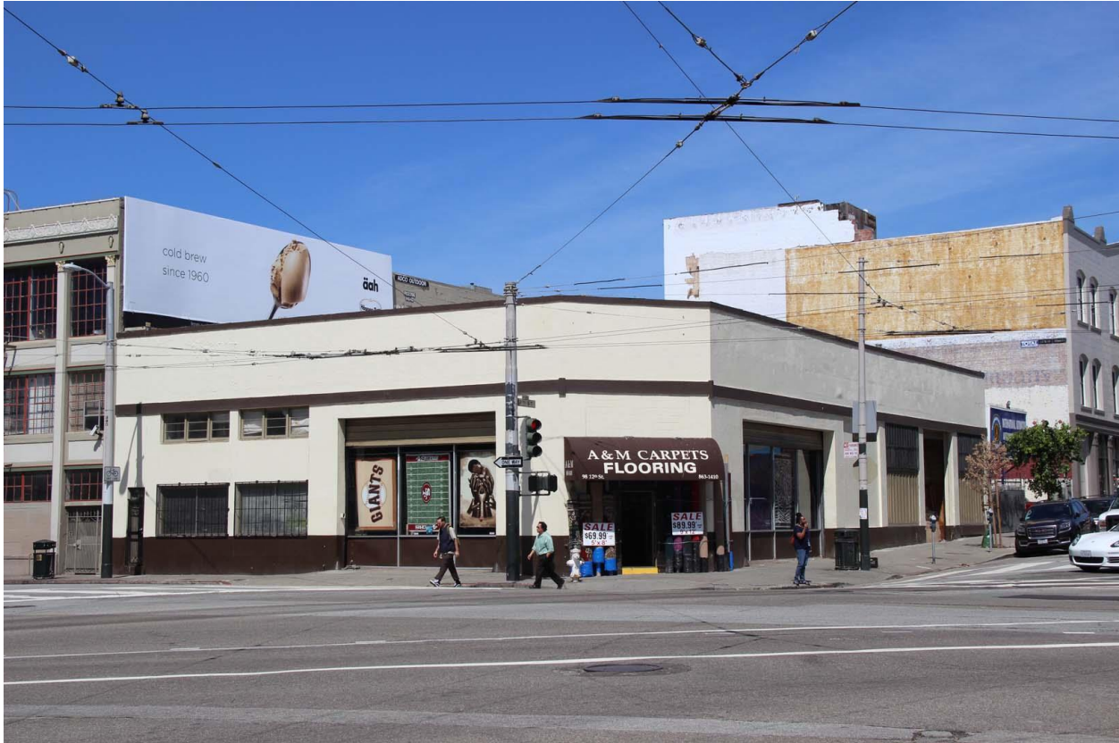
Figure 23. John McKee Building, overall view.
