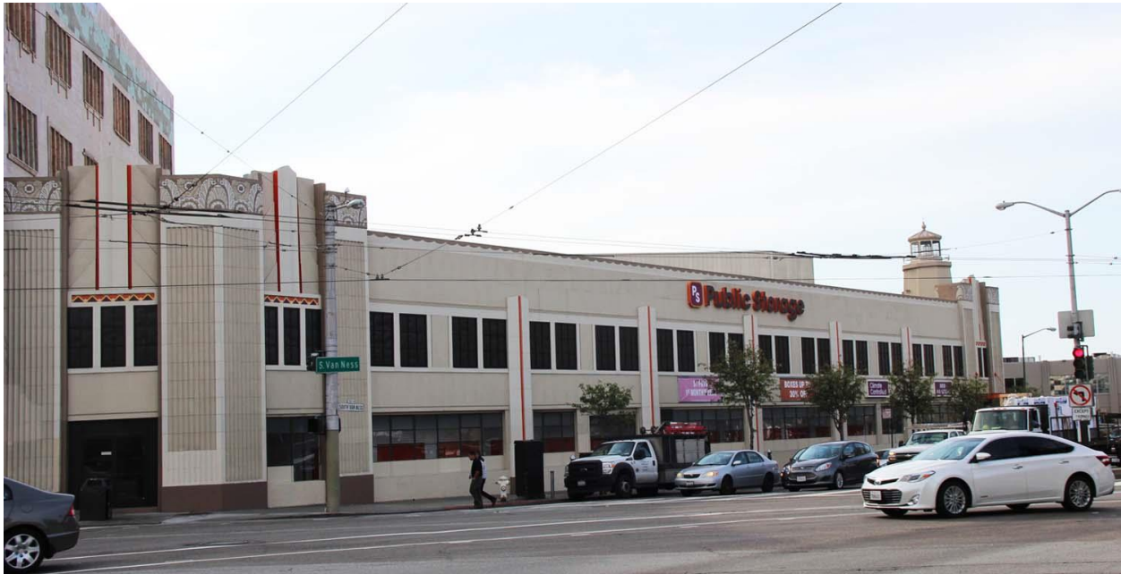
Figure 15. Recorder Printing Company Building at 99 South Van Ness Avenue, looking southeast.
