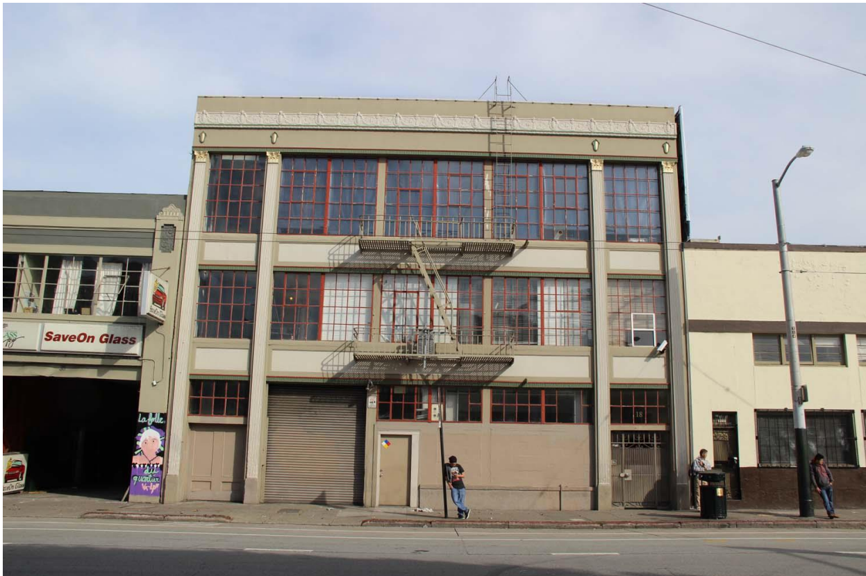
Figure 28. Former Lotus Fortune Cookie Co. Factory, primary façade, looking northwest.
