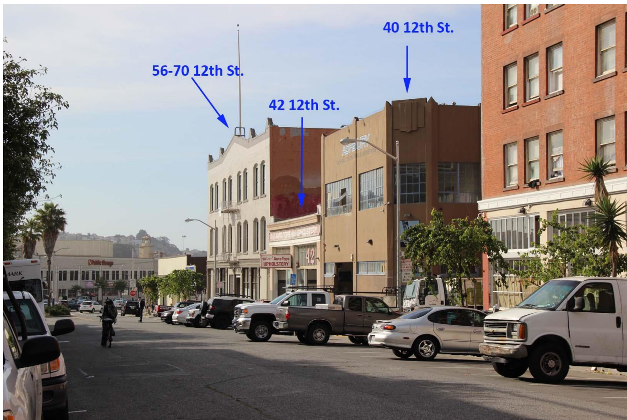
Figure 11. 12 th Street, looking southeast from Market Street.
