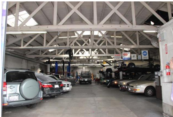
Figure 41. Former Hopkins Auto Repair Shop interior, looking northwest.
