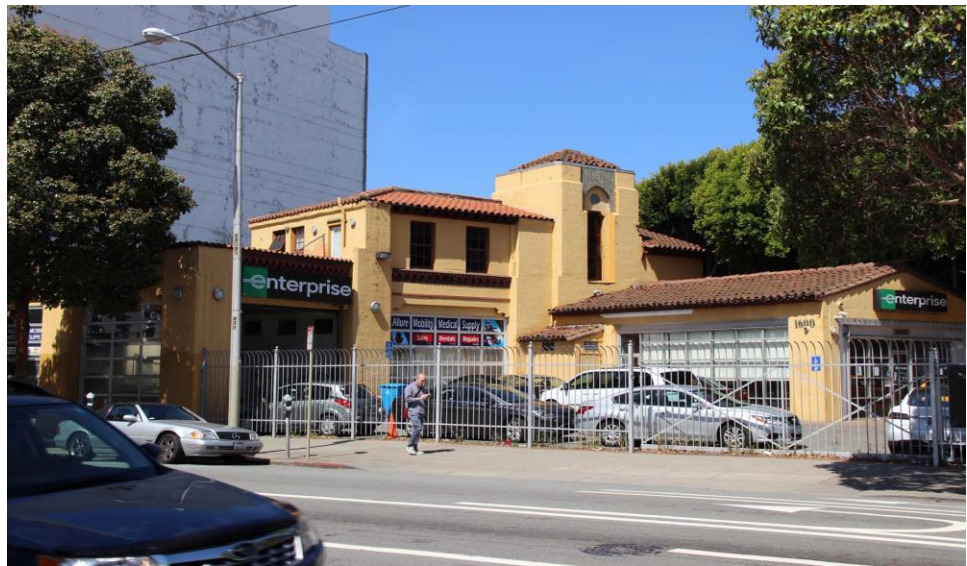
Figure 10. Granfield’s Service Station, 1600 Mission Street, looking west.
