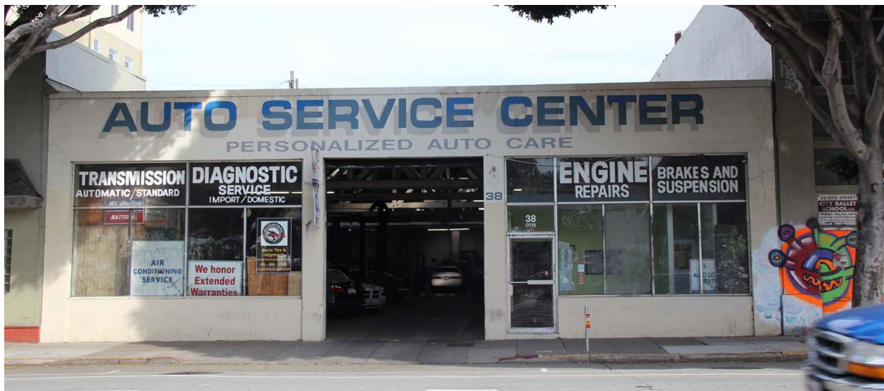
Figure 39. Former Hopkins Auto Repair Shop, primary façade, looking northwest.
