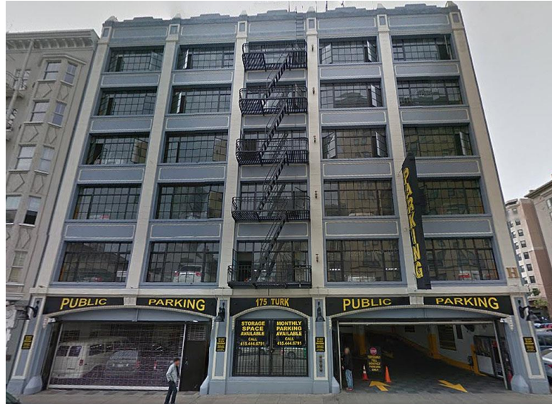
Figure 58. Bell Garage, 175 Turk Street Source: Google Maps
