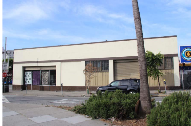
Figure 25. John McKee Building, northeast façade.
