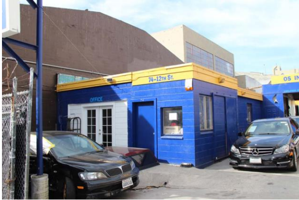
Figure 19. Former Mission-Van Ness Car Wash, office wing, looking southwest.
