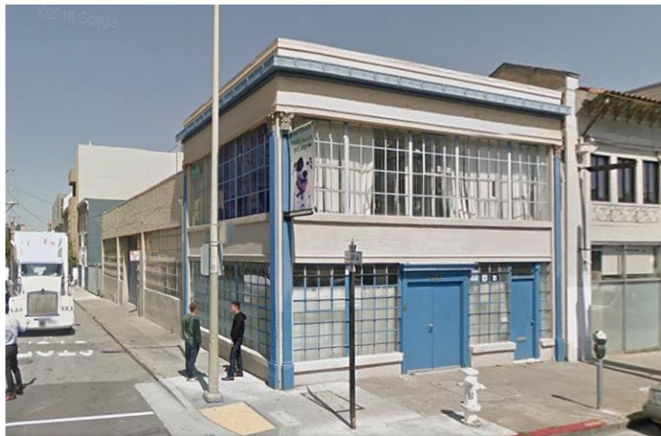
Figure 56. 234 9 th Street Source: Google Maps
