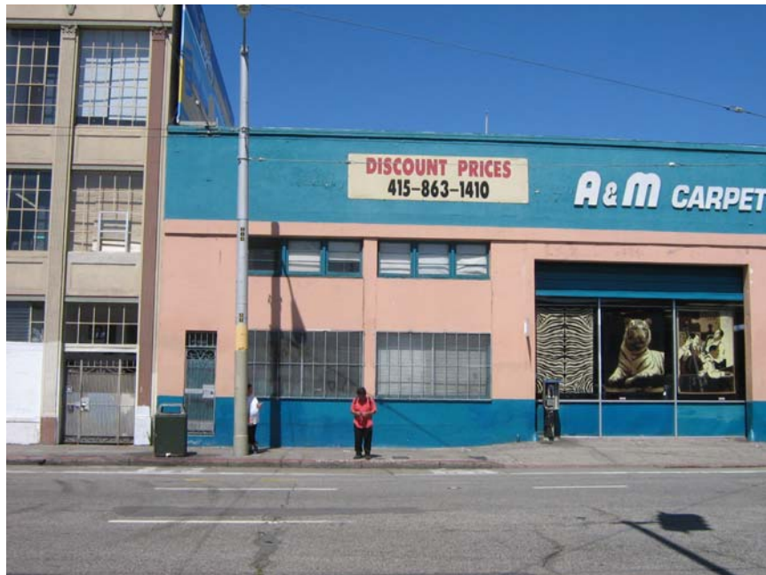
South half of south (Otis Street) elevation
