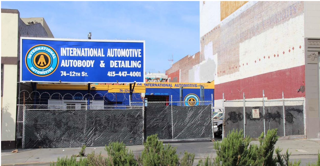
Figure 18. Former Mission-Van Ness Car Wash, looking southwest from South Van Ness Avenue.
