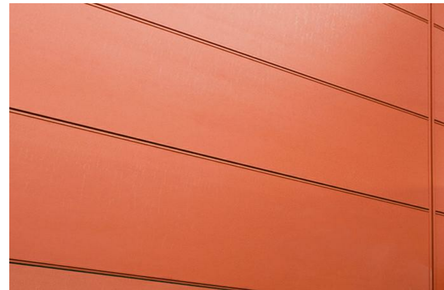
C. Stucco Reveal Joint
