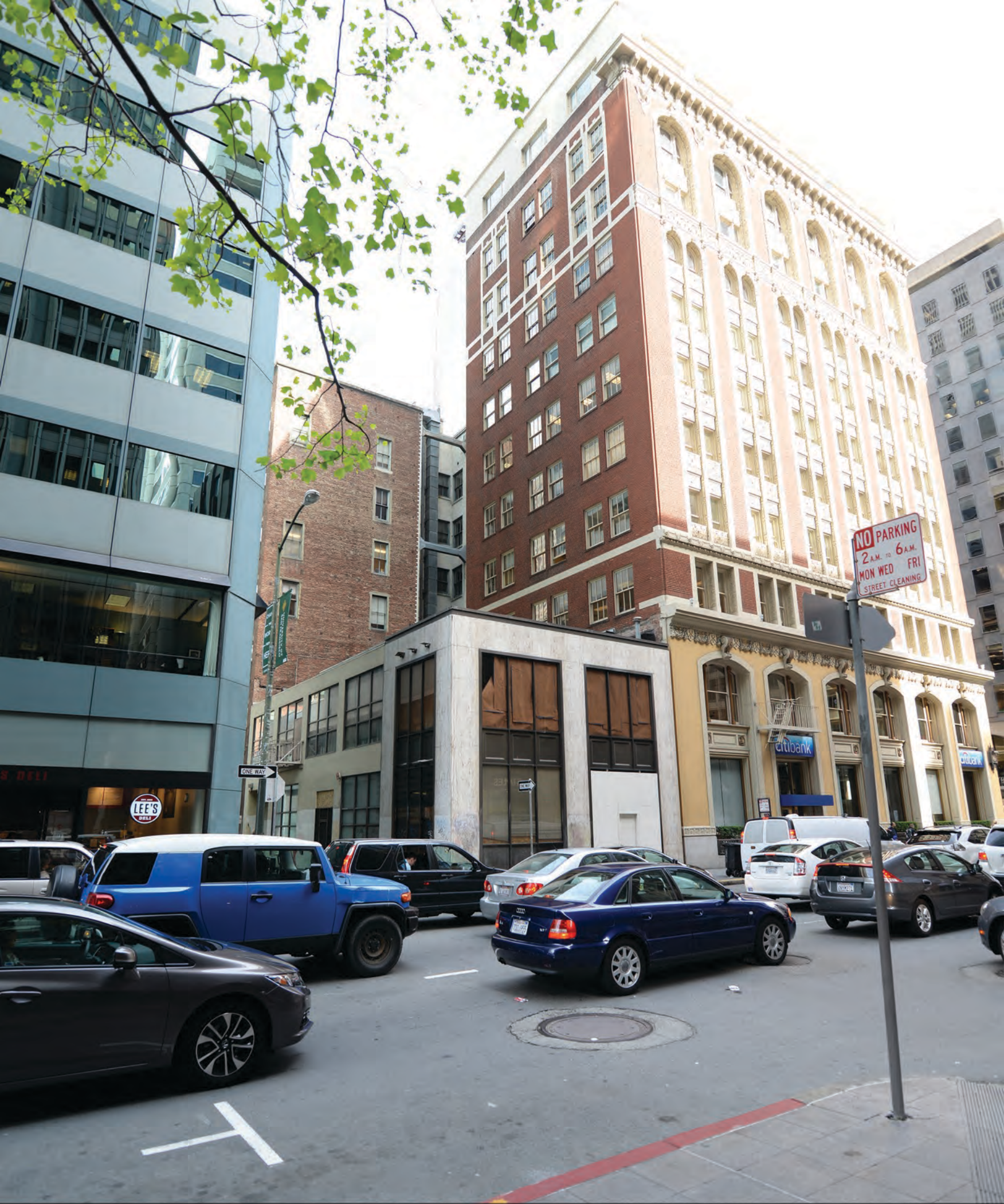
3. FRONT FACADE OF SUBJECT BUILDING, LOOKING SOUTH-EAST
