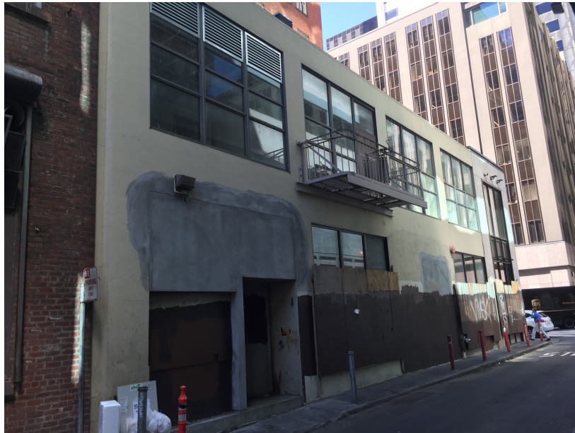
North facade, looking southwest from Halleck Street.
