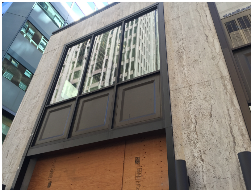
Detail of upper story bay, primary facade.
