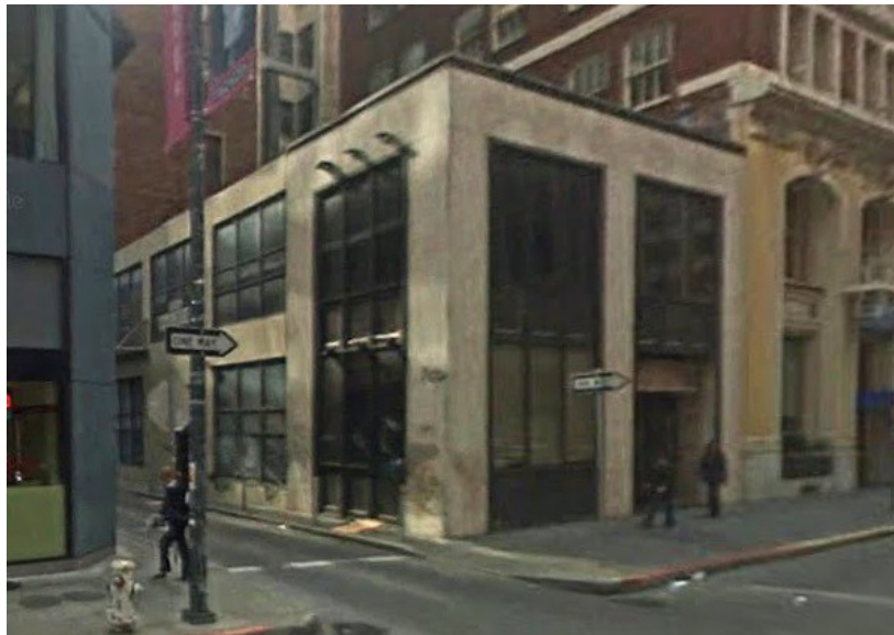
View of north facade before being boarded up (2008, Google street view).
