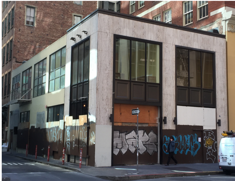
North and primary (west) facades, looking southeast.
