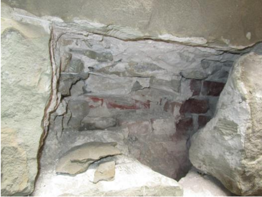
Original Construction: Brick backup wall behind Colusa sandstone veneer
