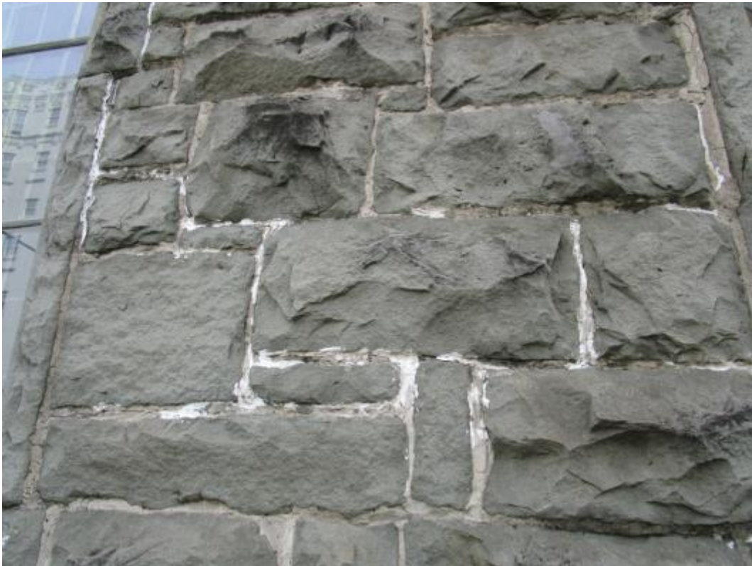
Colusa sandstone to be stabilized, cleaned and selectively repointed
