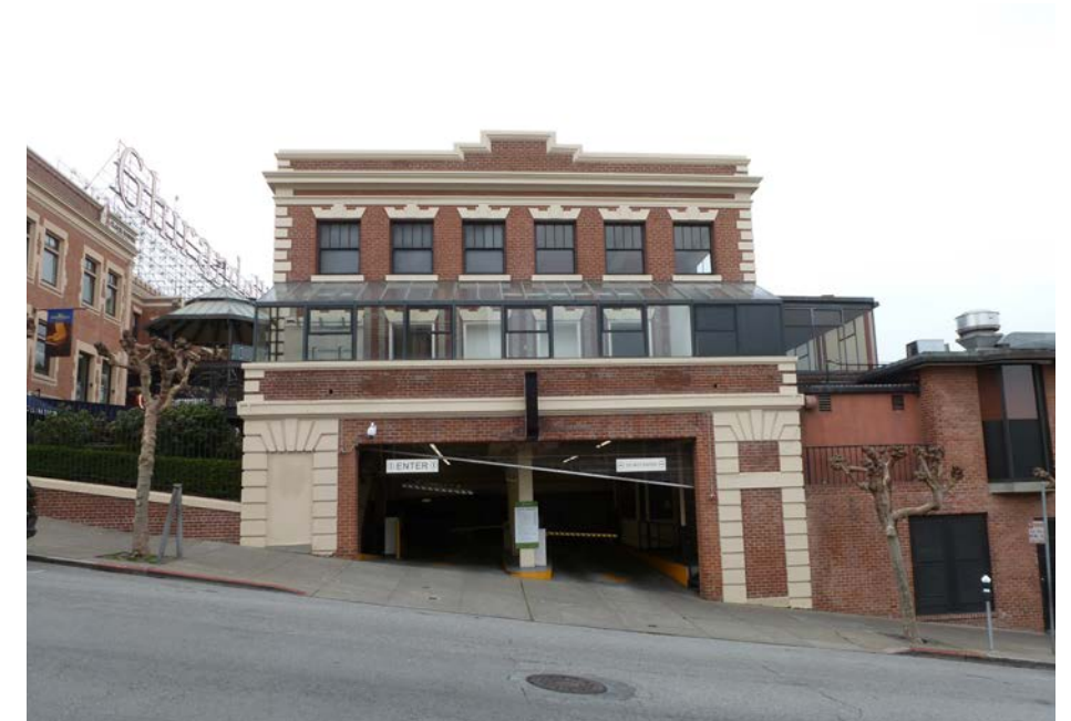
Apartment Building, east facade
