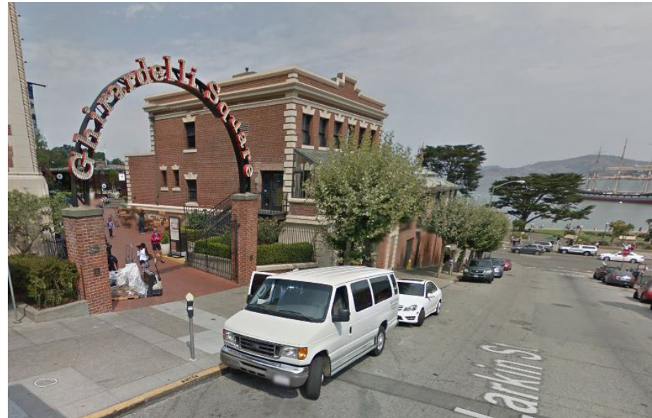
1: View looking northwest (mechanical equipment minimally visible), Google Maps, 09-18-2015
