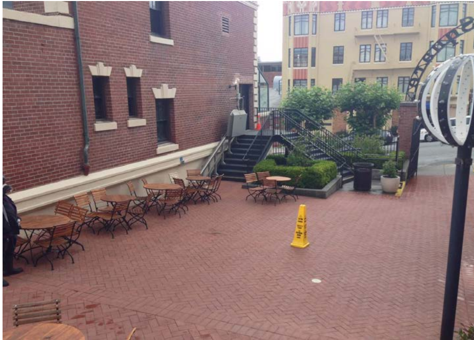
Existing ADA entrance to the Apartment Building
