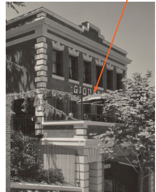
Photo of the east elevation of the Apartment Building shortly after the 1960s work. Note that the existing glass shed addition on the east side had not yet been constructed.
