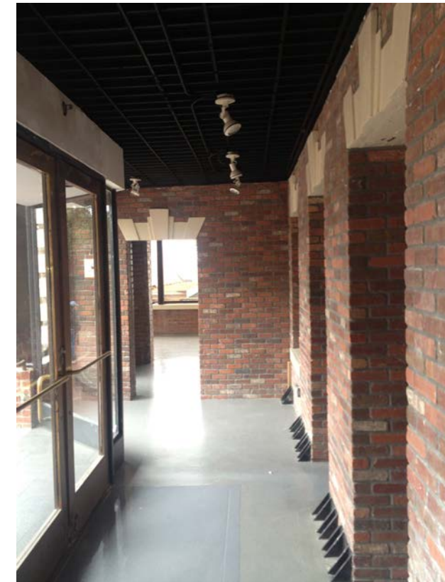
Photo of existing ceiling at proposed outdoor seating area.
