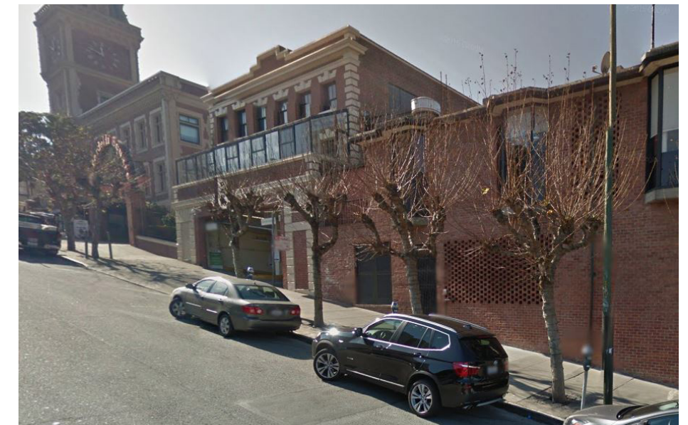
3: View looking southwest (mechanical equipment not visible), Google Maps, 09-18-2015
