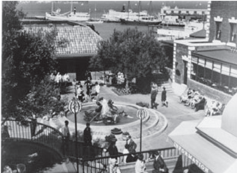
6. View looking north, Fountain Plaza and Apartment Building in view. Note that there are no steps at the Apartment Building and the storefront spans straight across the two projecting wings of the building (Aquaticpark.org)
