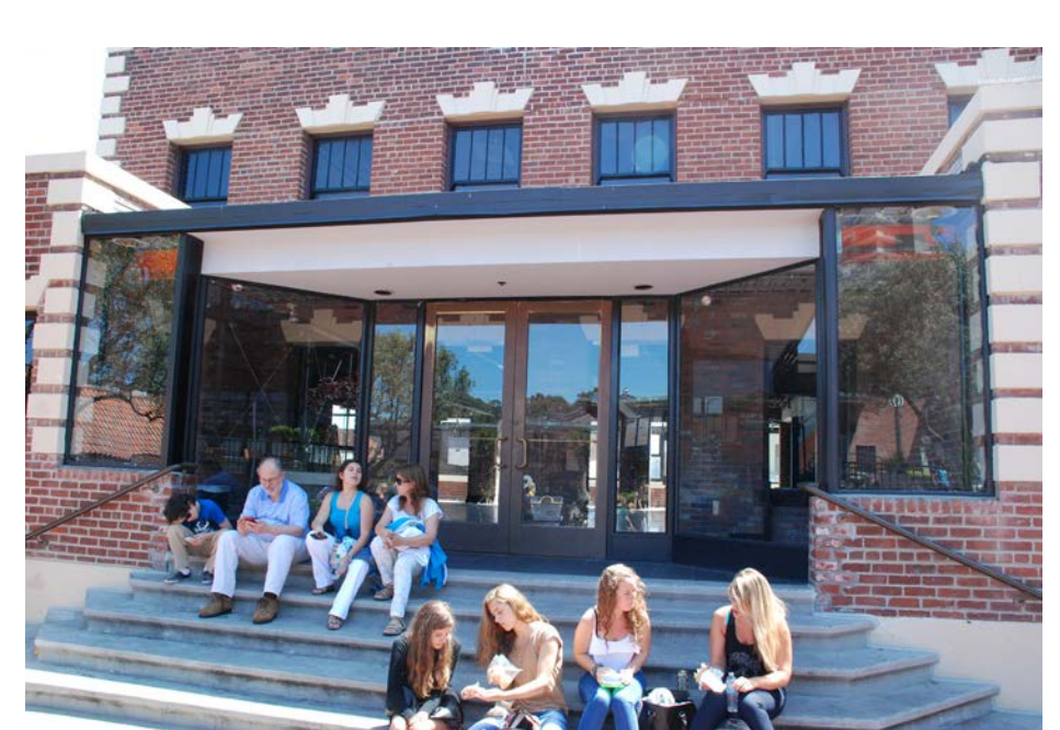
Apartment Building, close up view of existing storefront at west facade
