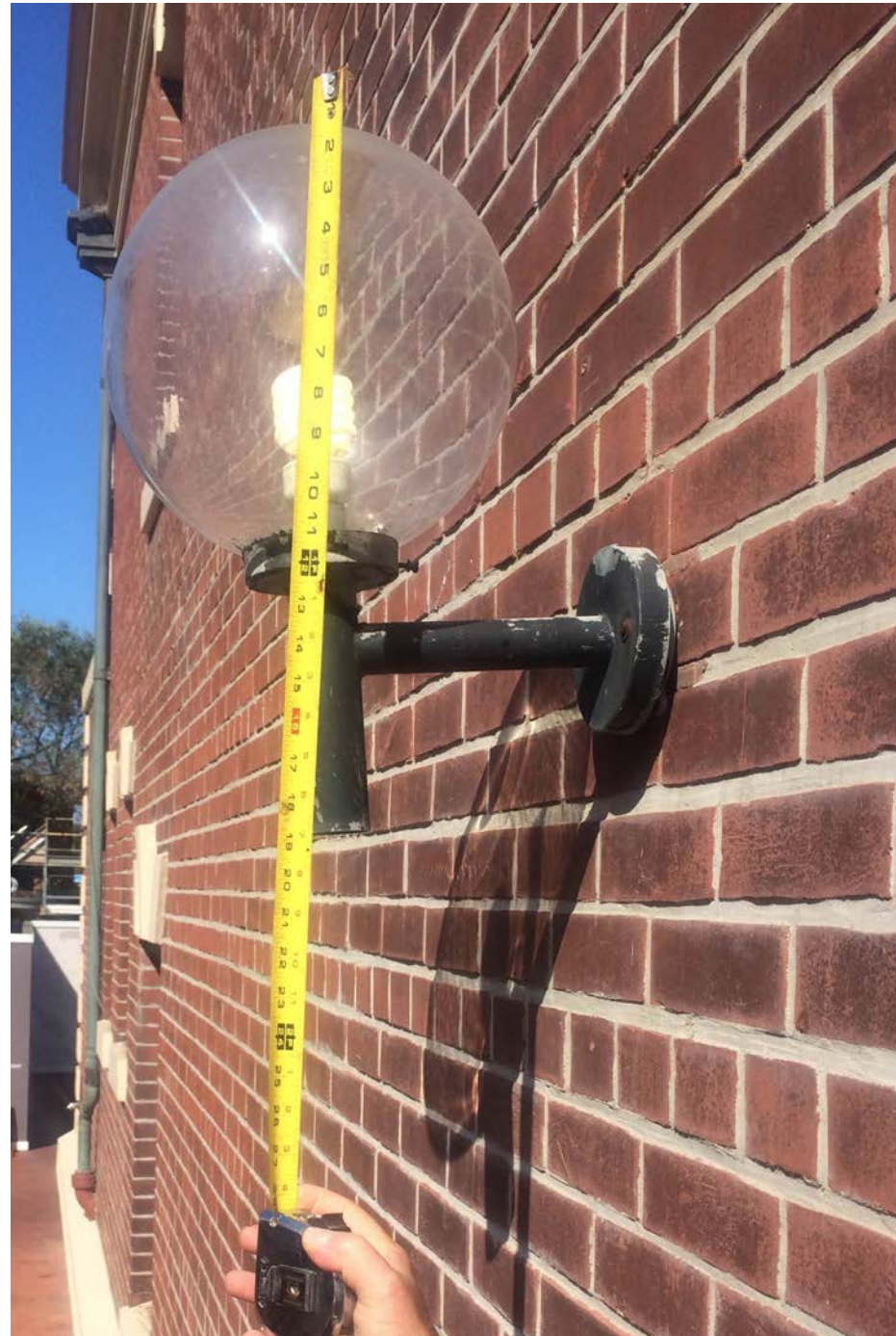
Photo of existing sconce. (E) light to be retained at west facade. (E) at south facade to be relocated to west facade.
