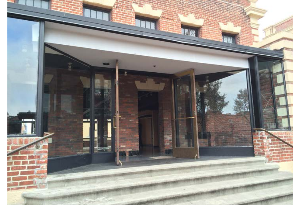
Non-historic storefront addition at west facade of Apartment Building
