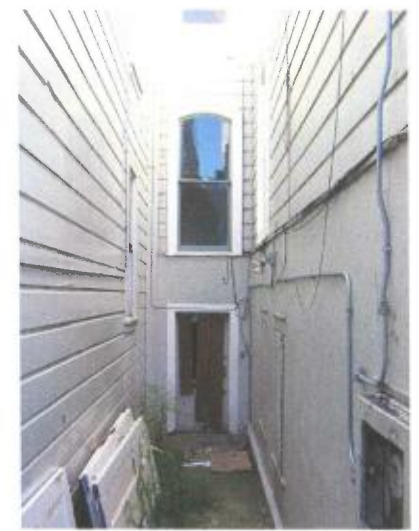
South walkway showing location for new door
