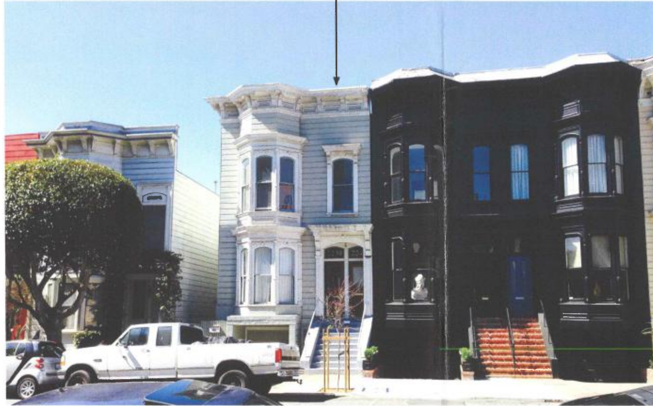
East facade and adjacent properties
