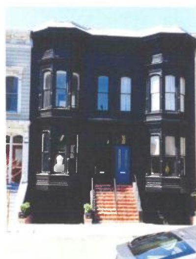
Neighboring properties to the north 2245 and 2247 Webster Street
