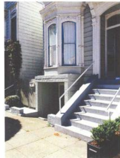
Existing bay where work is to occur (remove brick, add trim)
