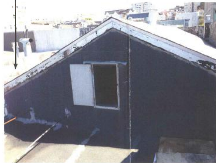
Existing roof, looking east
