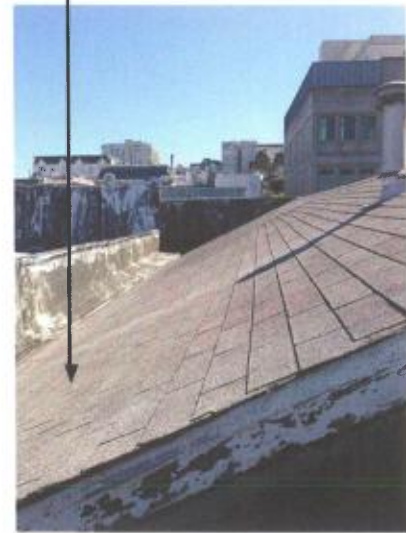
Existing roof, looking east
