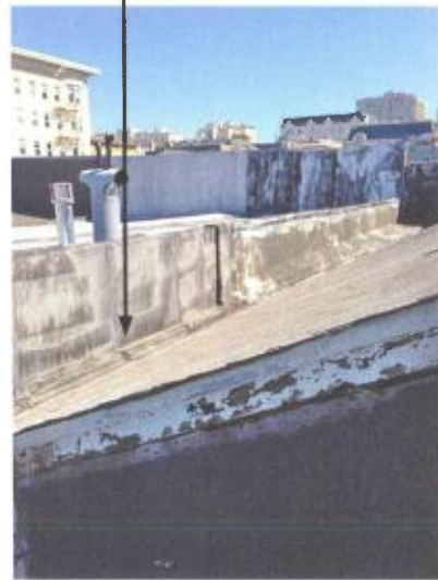
Existing roof, looking east
