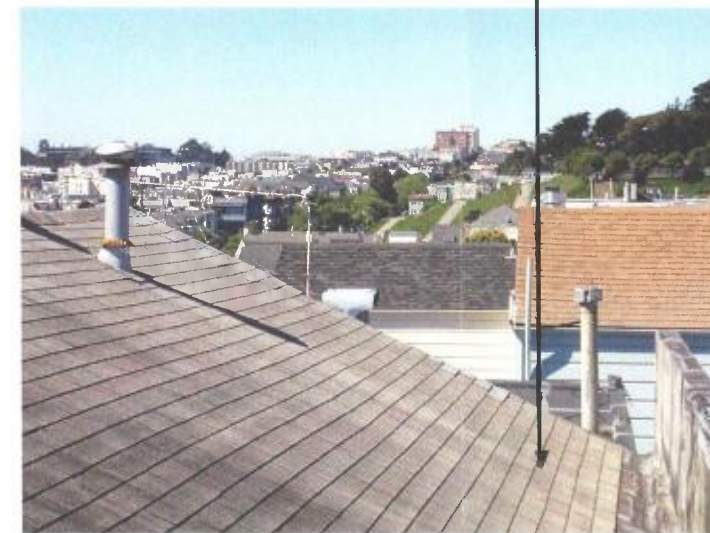
Existing roof, looking west
