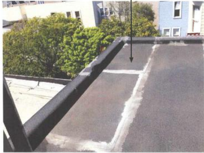
Existing roof deck, looking west
