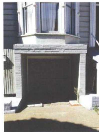
2239-41 Webster Street Subject Property
