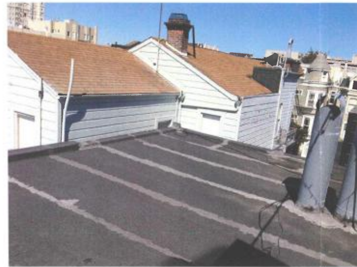
Existing roof deck, looking northwest
