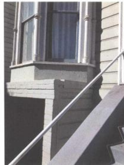
Existing bay where work is to occur (remove brick, add trim)
