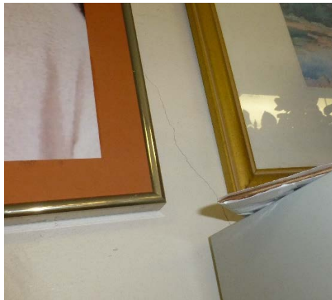
Figure 14: Cracking of plaster wall.
