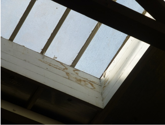
Figure 21: Water damage to wood paneling near skylight.
