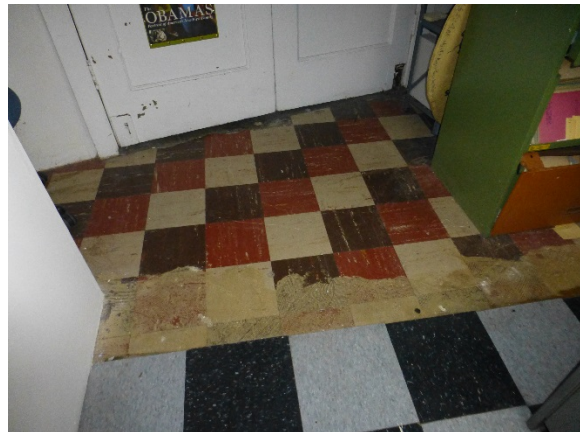
Figure 28: Exposure of multiple layers of flooring.
